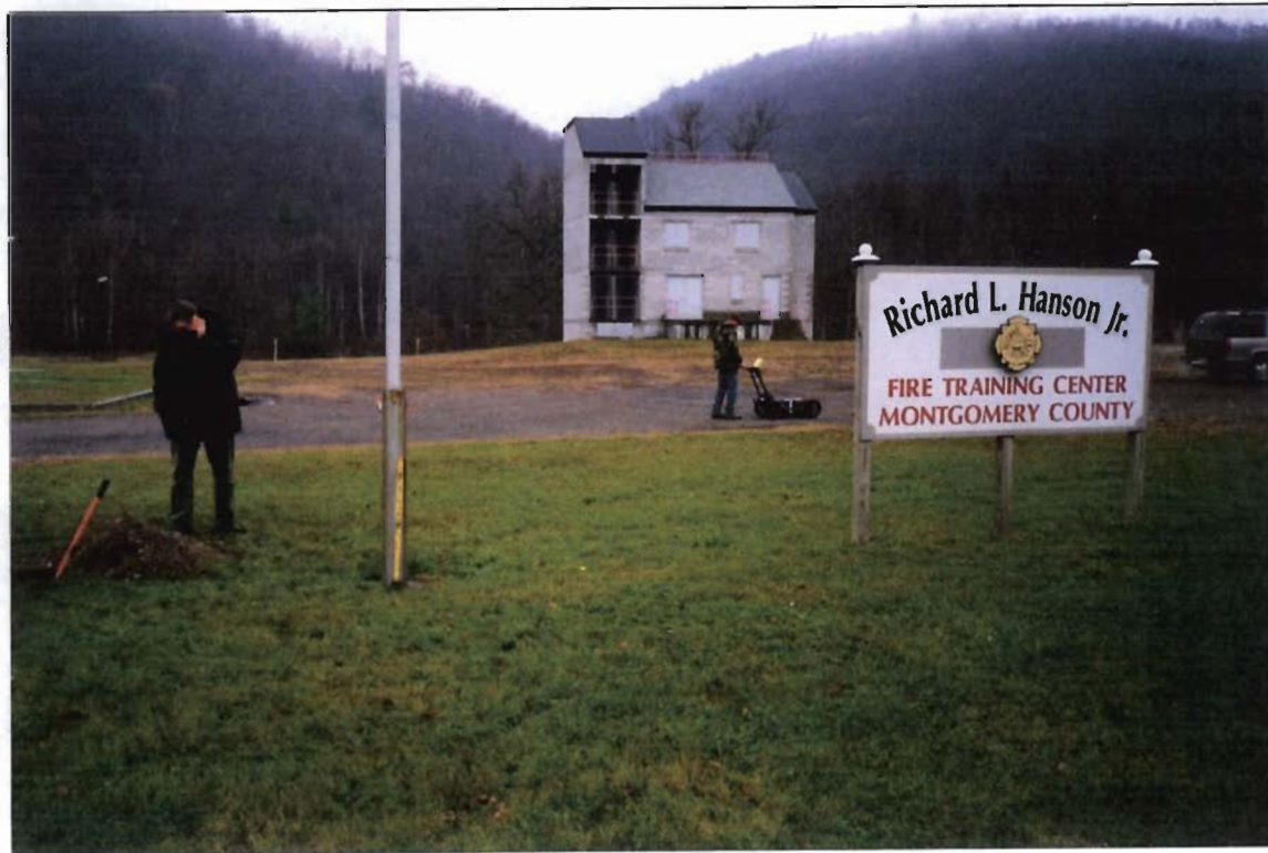
General Site Photo
