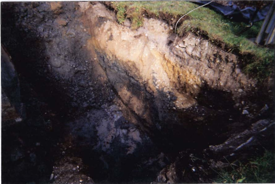
Subsurface conditions after excavation of contaminated soil. Note: residual contamination and stained soil in the sidewalls of the tank excavation.
