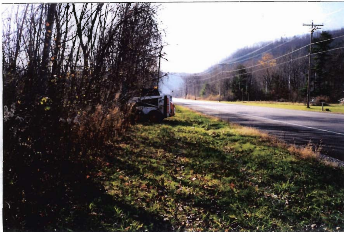
Installation of monitoring well MW-19 located along NYS Route 5.
