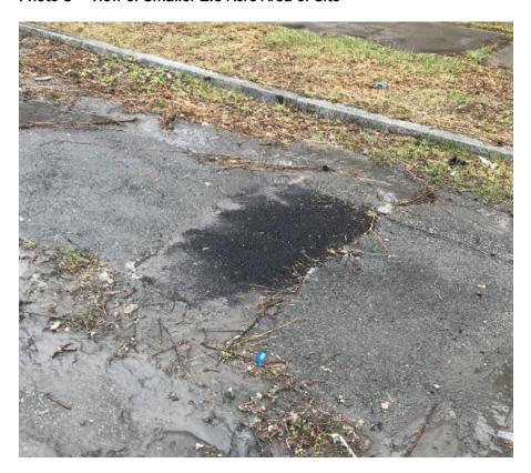
Photo 4 - View of Asphalt Patch Where Vacuum Excavation Occurred
