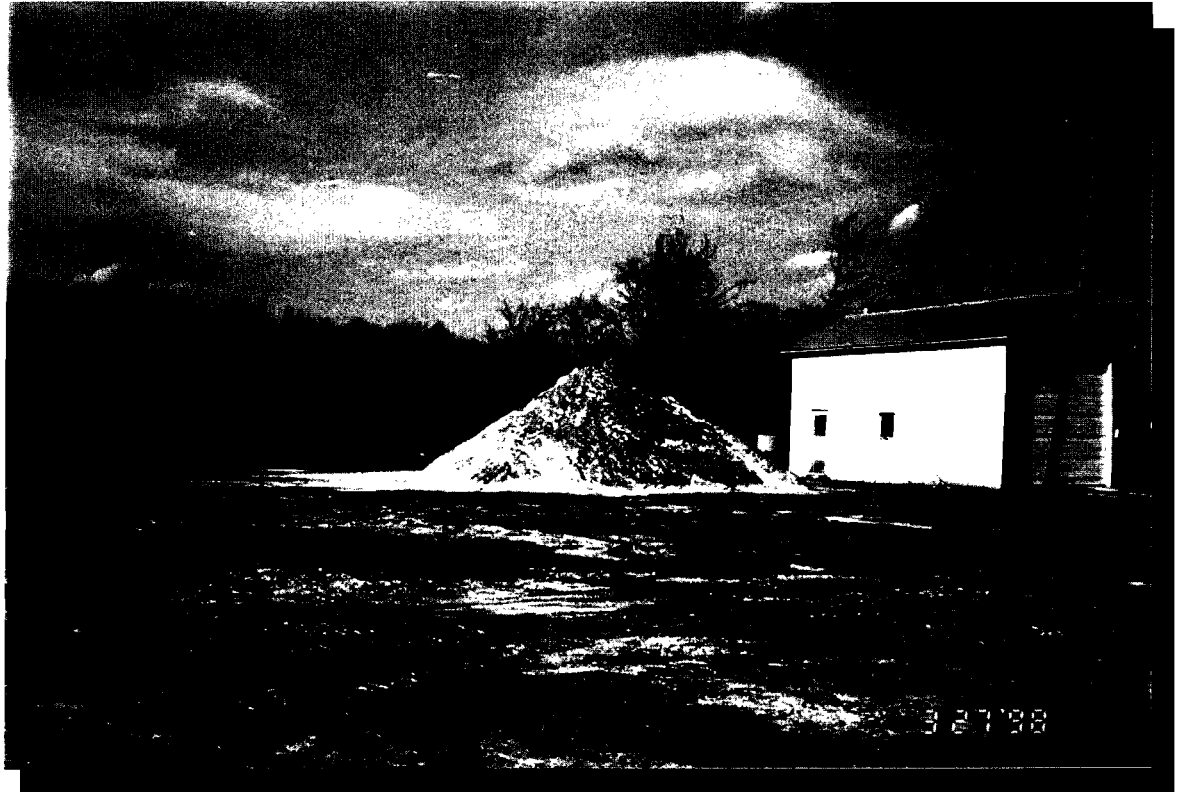
Photo #9 Uncovered road salt and salt precipitate visible near the Town of Gainesville garage (looking northeast).
