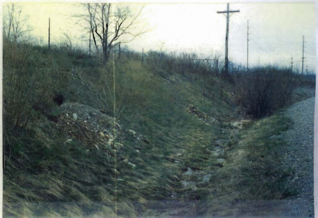
VIEW OF DITCH RECEIVING LEACHATE / FACING NORTH
