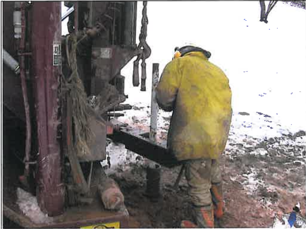
Photo 5. Photo of driller installing monitoring well at B-6.
