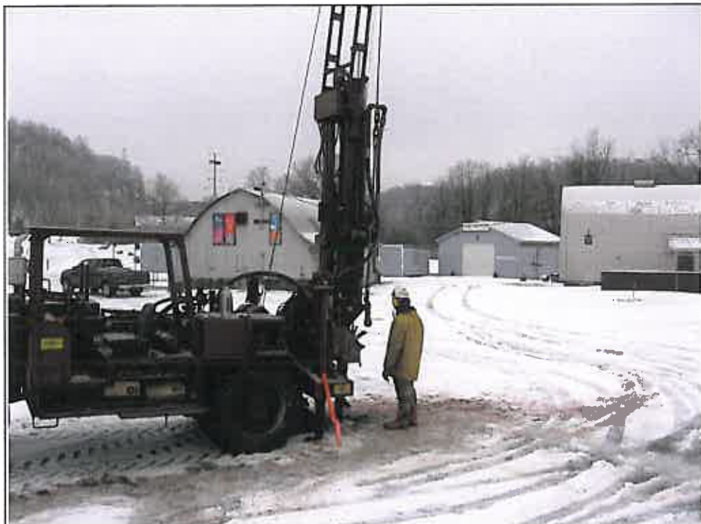
Photo 4. Photo of CME 550 ATV drill rig.
