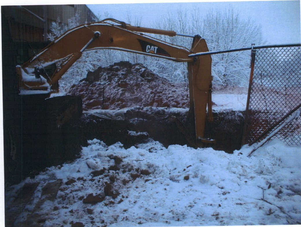
Photo 1: Excavating OU3 soil, clean stockpile visible in background.
