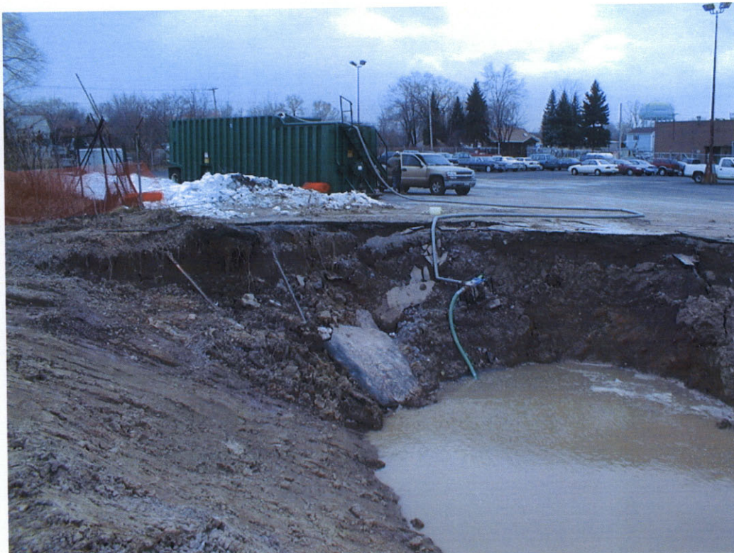
Photo 12: Pumping water from excavation into a portable storage tank.
