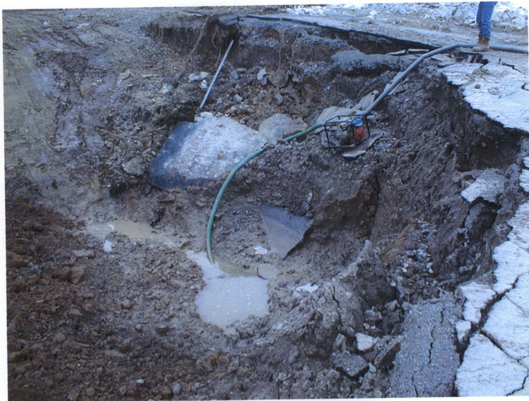
Photo 14: Excavation has been completely dewatered.
