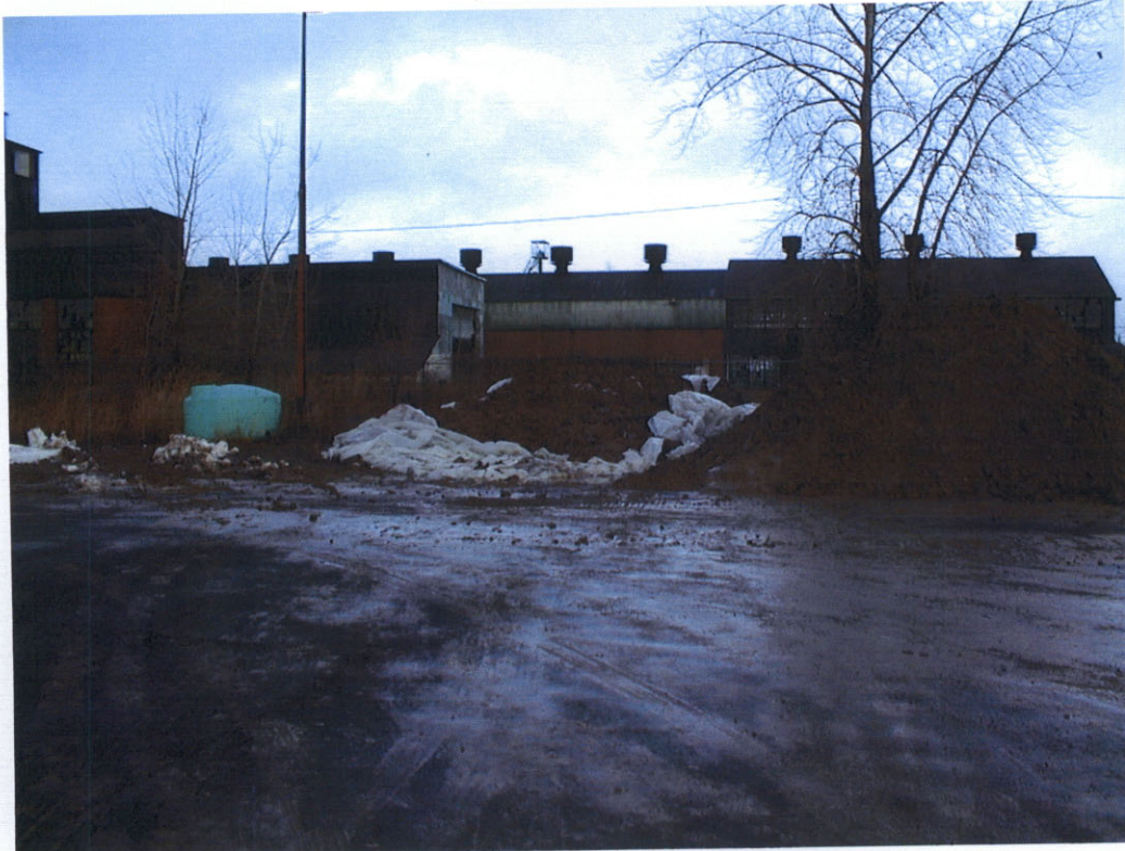
Photo 11: Action-level soil stockpiled on plastic sheeting prior to disposal
