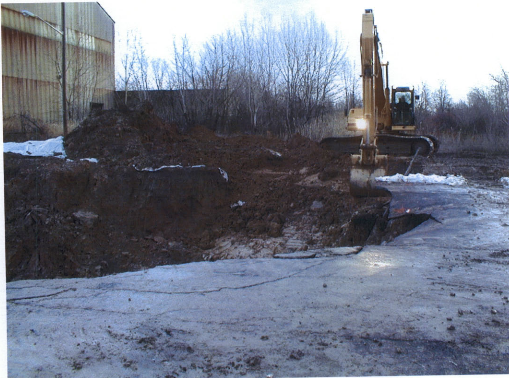
Photo 9: Backfilling excavation with clean stockpiled soil.
