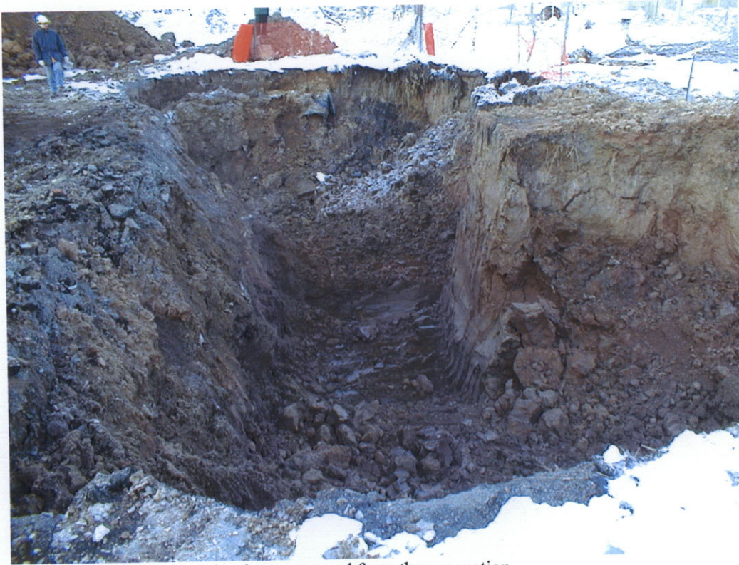
Photo 5: Action-level soil has been removed from the excavation.
