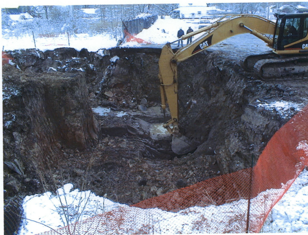
Photo 8: Excavating down to a maximum depth of 21 feet.
