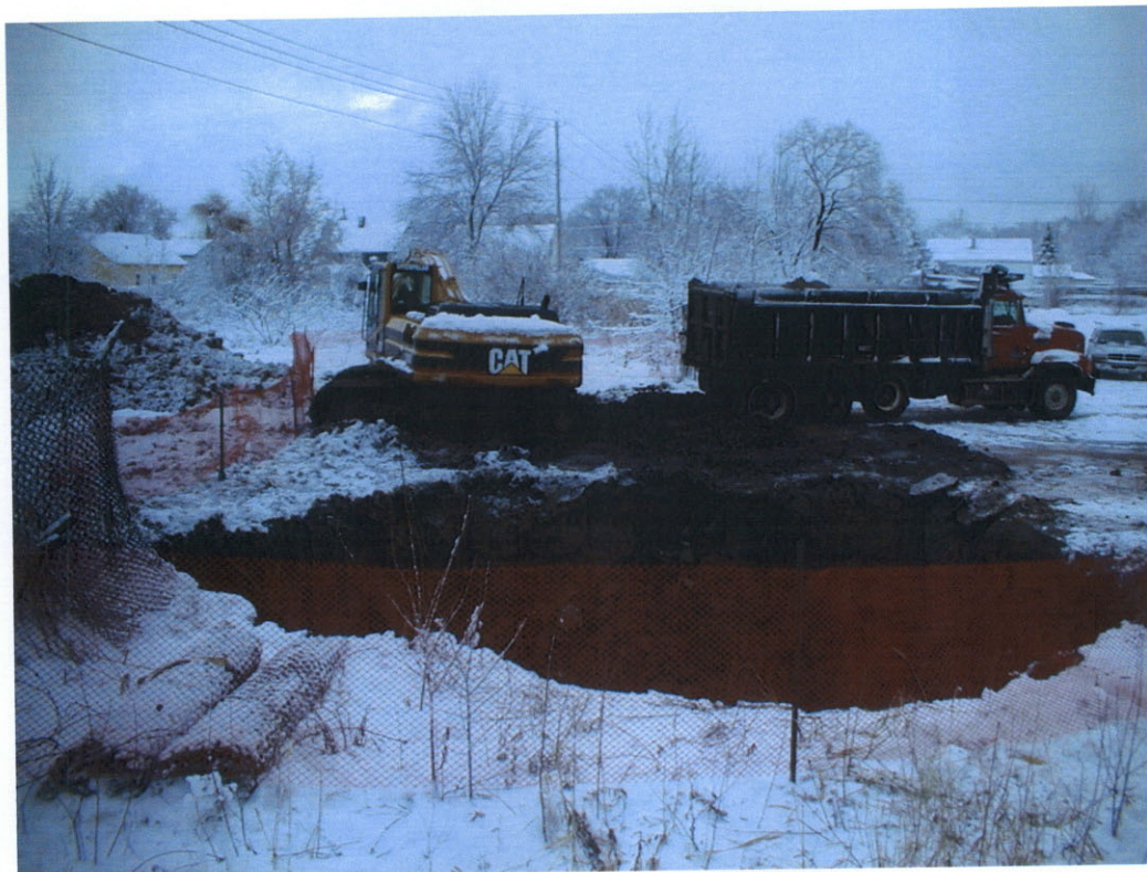
Photo 2: Excavating non-hazardous soil from OU3 for disposal.
