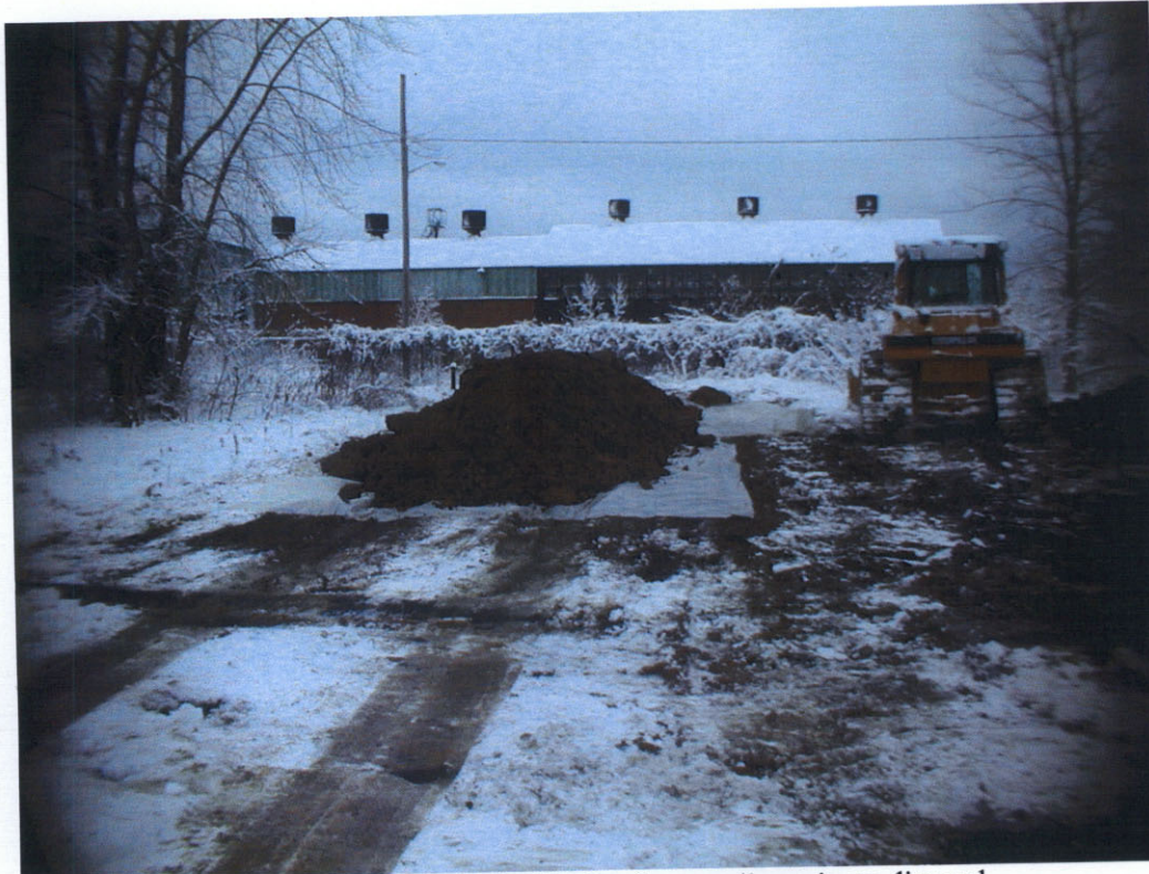
Photo 3: On-site soil stockpiled on plastic sheeting for sampling prior to disposal.
