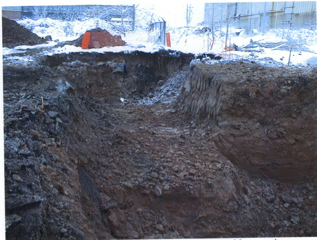
Photo 4: Action-level soil identified during the IRM has been exposed for excavation.
