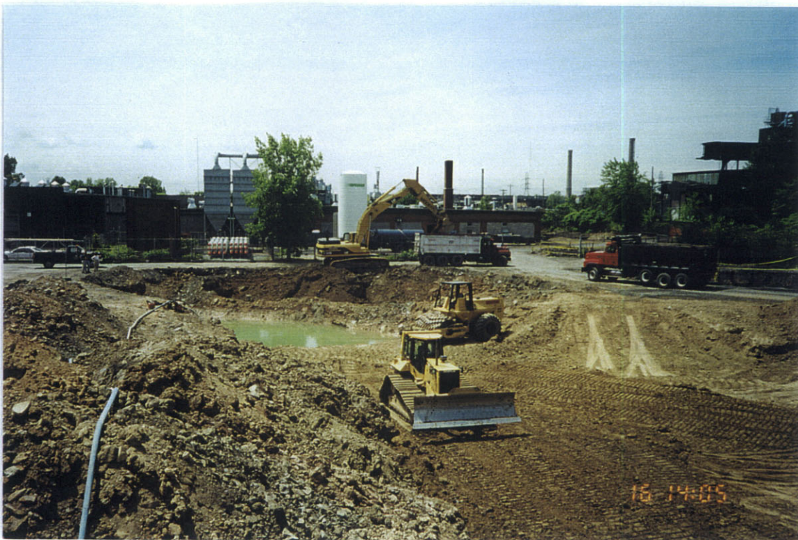
Photo 6: West view of activity in west end of area 2A.
