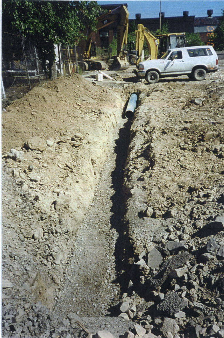
Photo 17: North view of trench and installation of new drain pipe.
