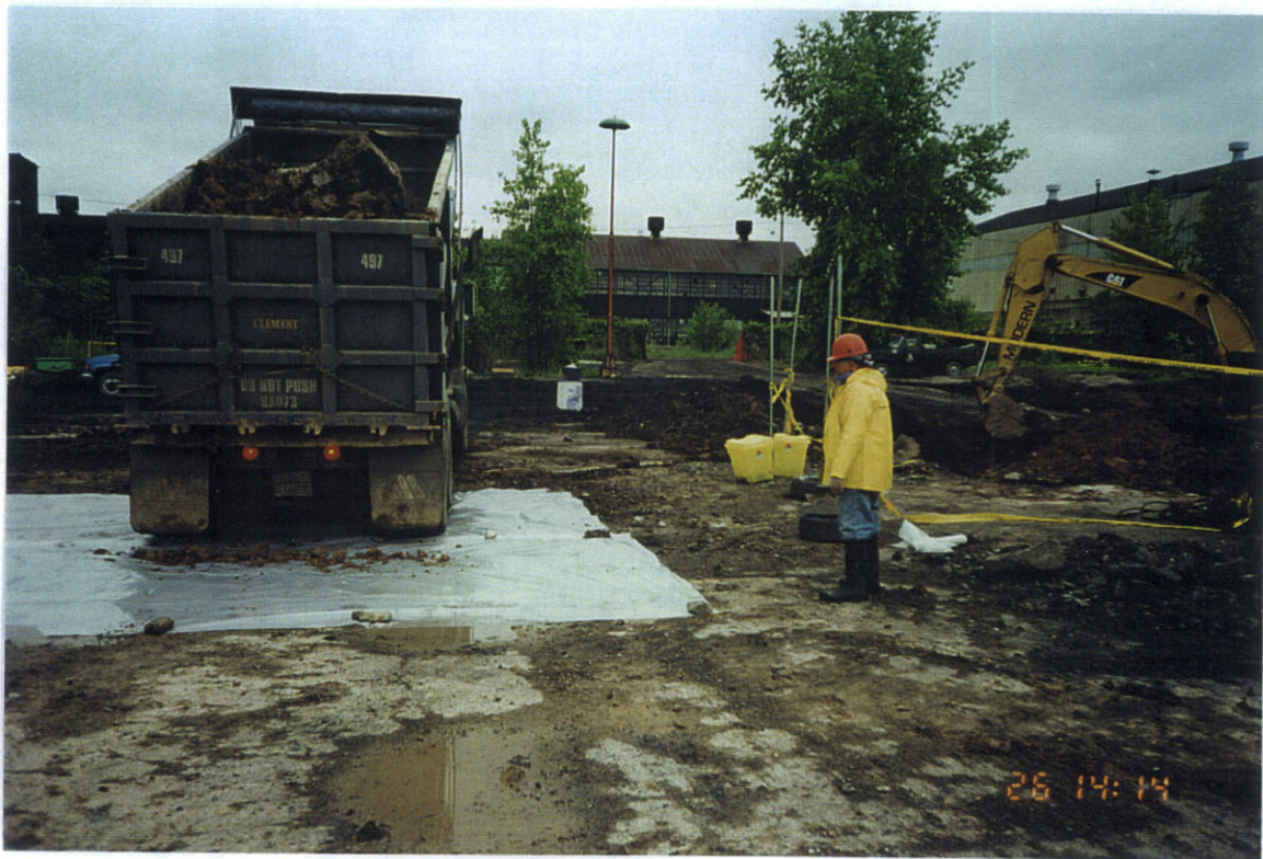
Photo 12: Stockpiling contaminated soil on plastic sheeting.
