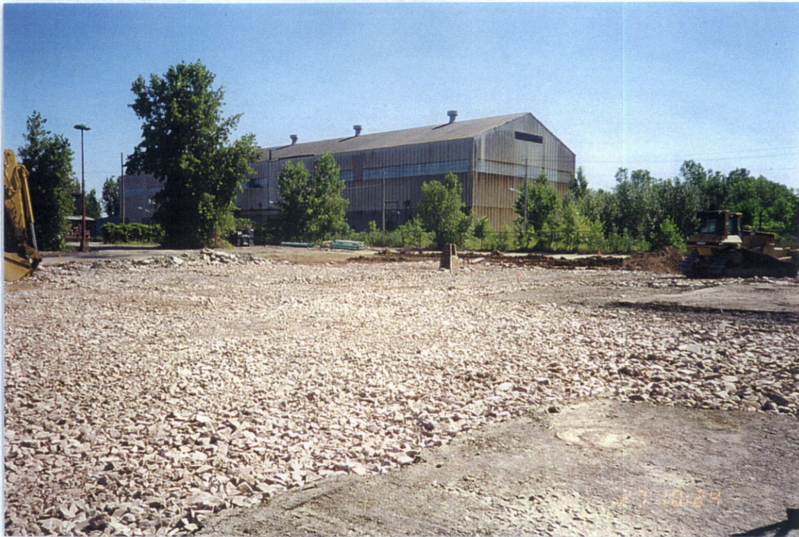
Photo 18: North-east view of areas 2A and 2B backfilled and stone placed.
