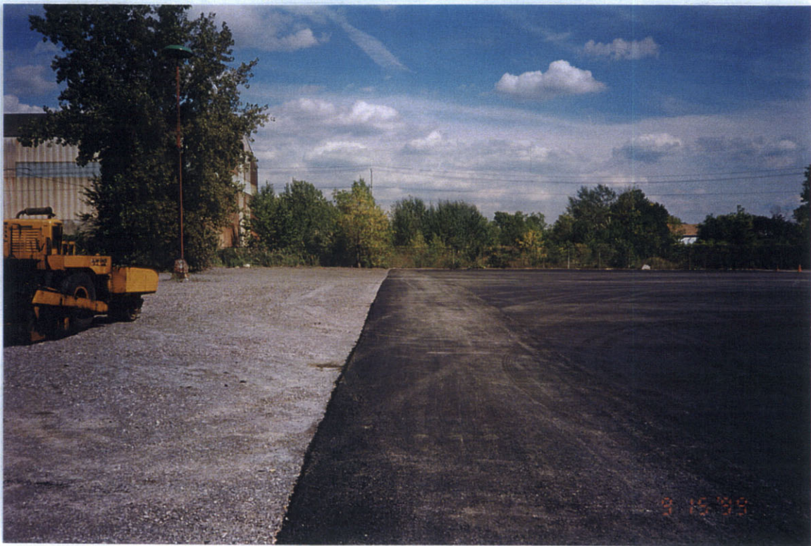
Photo 19: East view of extent of paving in area 2A.
