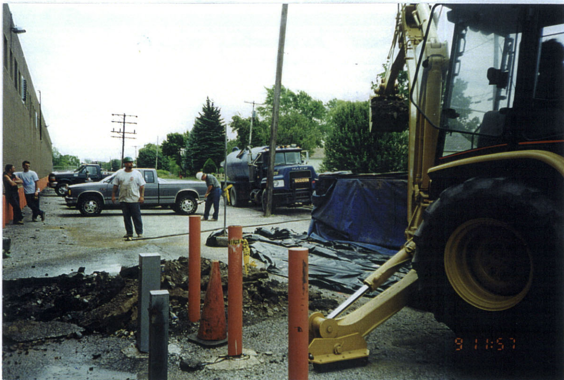
Photo 16: East view of soil from area 5 being loaded directly into roll-offs.
