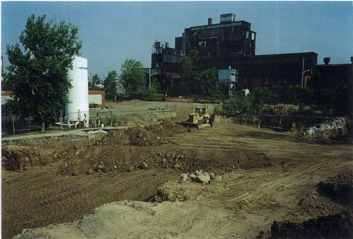
Photo 15: North view of backfilling in areas 2C and 1D-extension.
