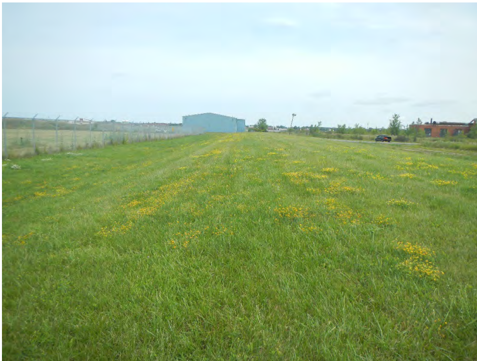
Photo 16 - View of south side of cap
