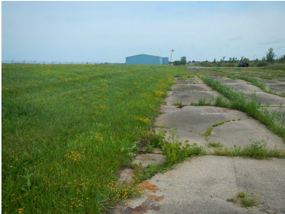
Photo 22 - View of east side of cap
