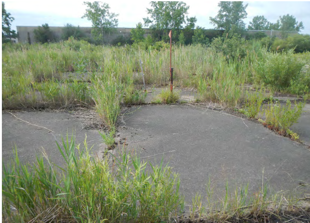
Photo 28 - View of concrete area east of Site with monitoring wells
