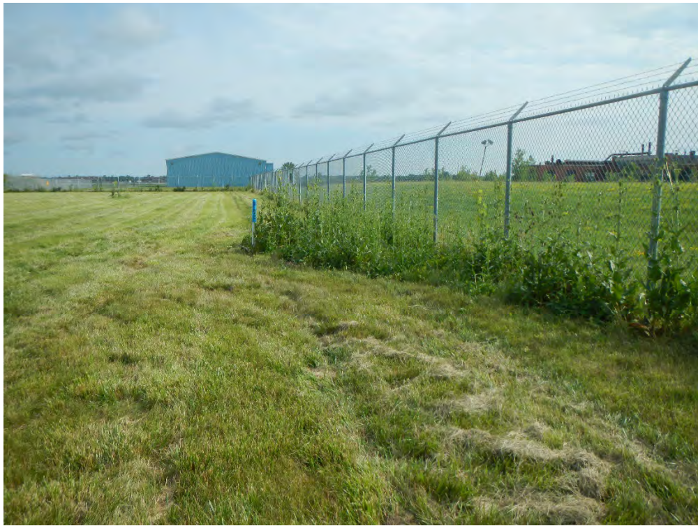
Photo 7 - View of west side of cap viewed from NFTA property
