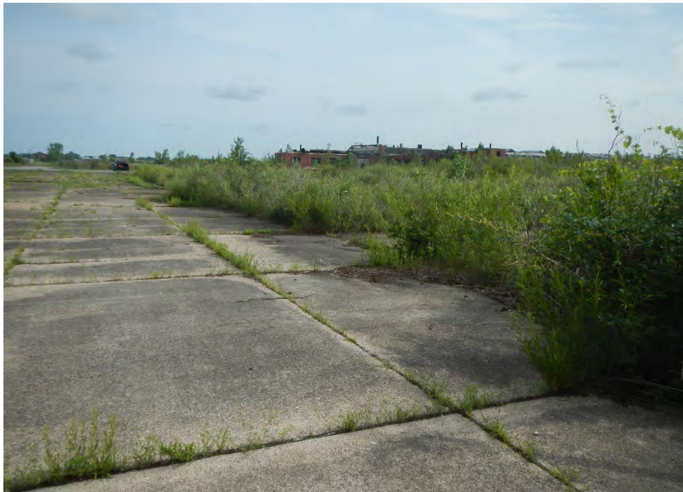
Photo 29 - View of concrete area east of Site with monitoring wells
