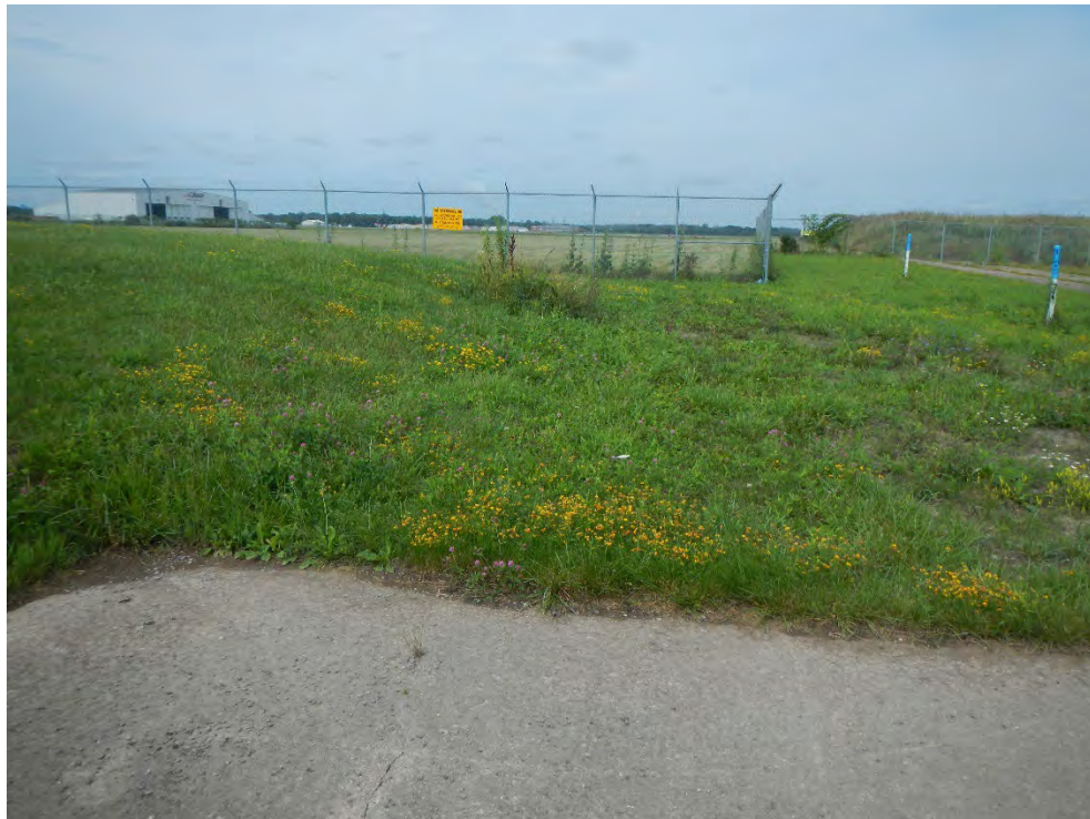
Photo 9 - View of north side of cap
