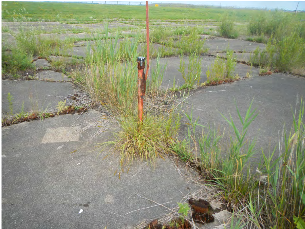
Photo 24 - View of OMW-5 east of Site
