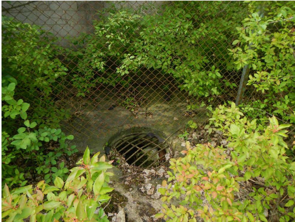
Photo 32 - View of MH at south edge of Site
