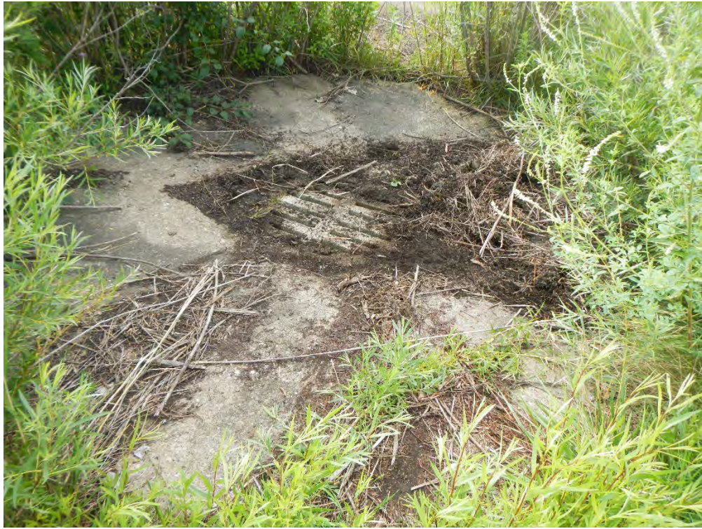
Photo 31 - View of manhole MH A-10
