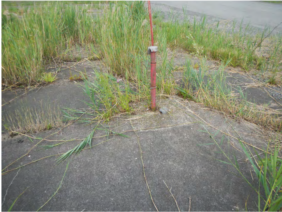
Photo 25 - View of OMW4-81 east of Site
