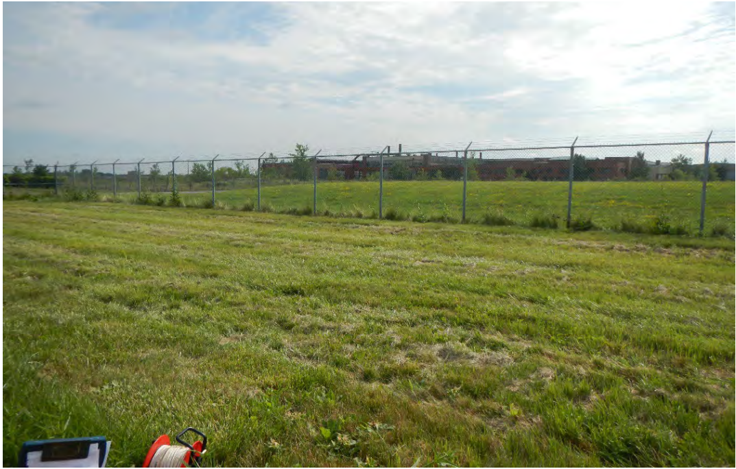
Photo 3 - View of west side of cap viewed from NFTA property
