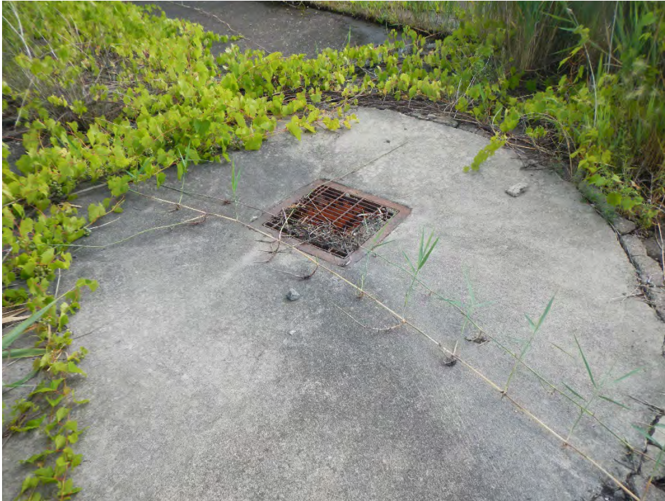
Photo 26 - View of MH A-9 east of Site
