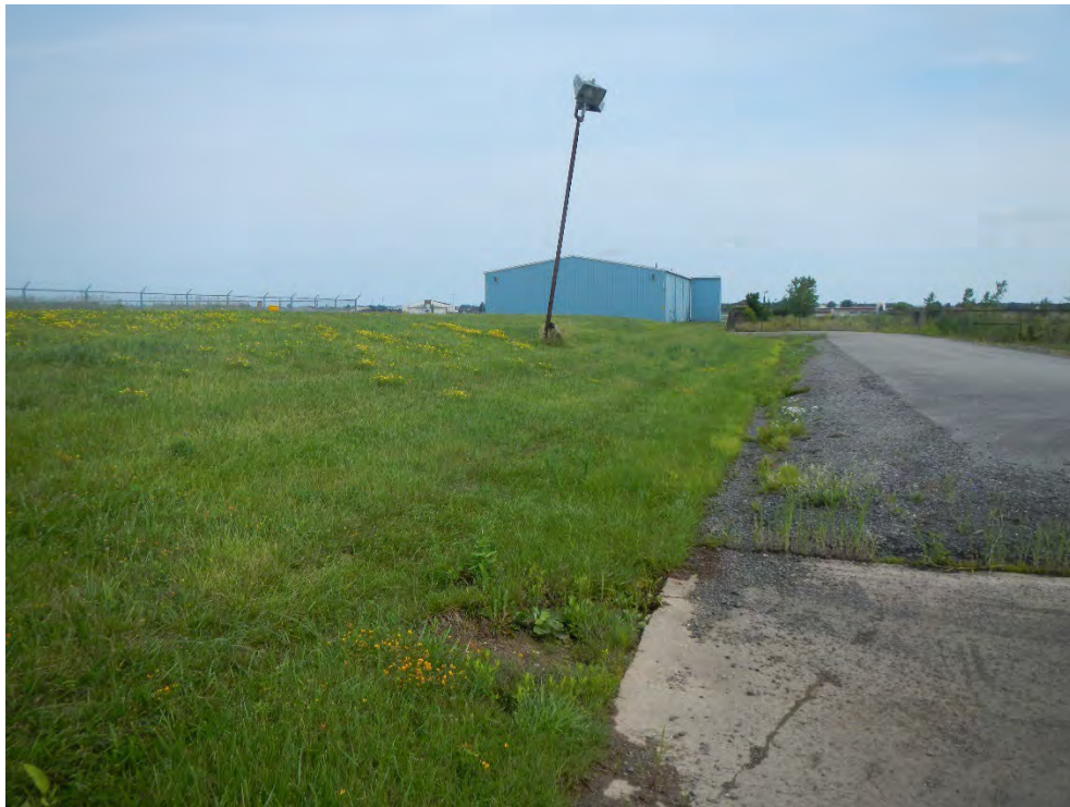
Photo 23 - View of east side of cap
