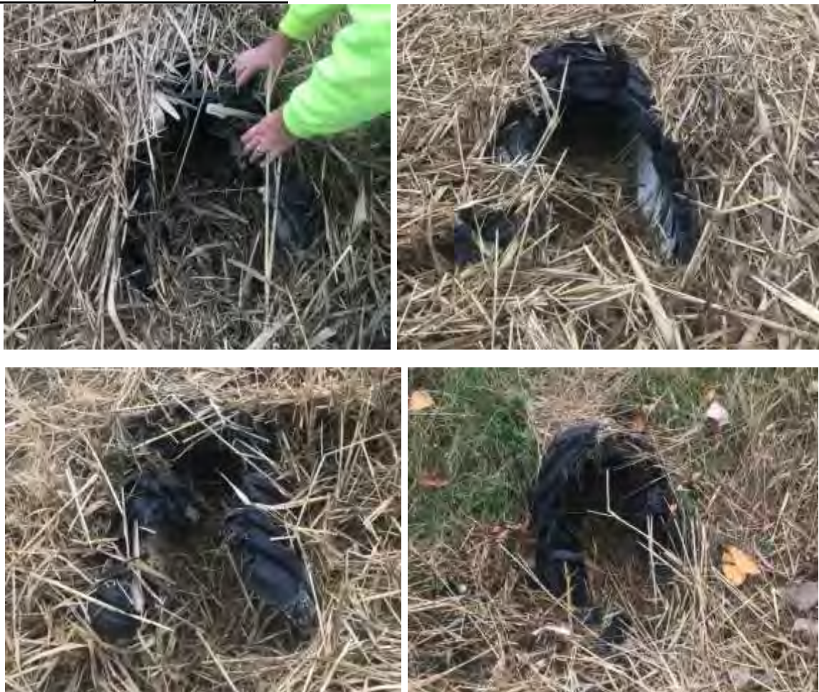
Minor damage to culverts, no standing water 10/26/20 NWP
