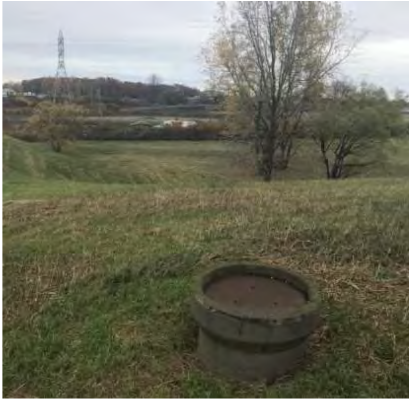
From road on top of cell 2 looking North
