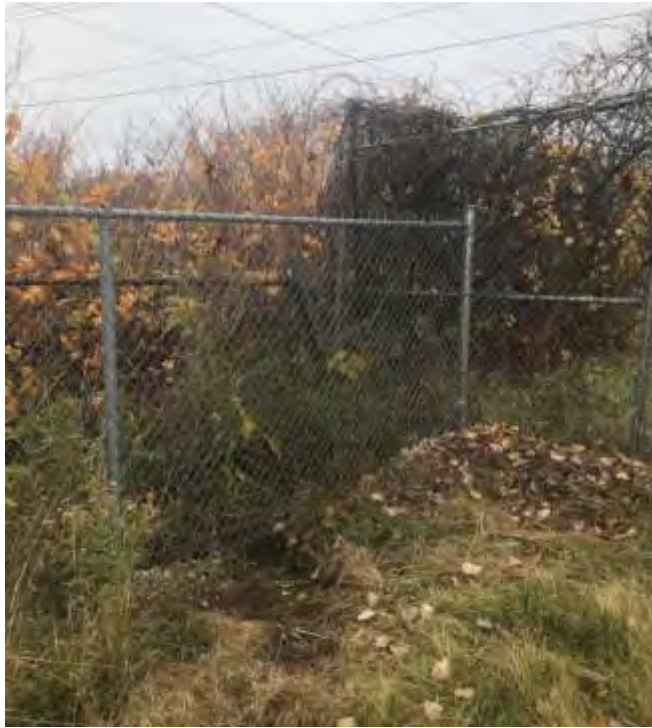
Northeast corner fencing, good condition 10/26/20 NWP
