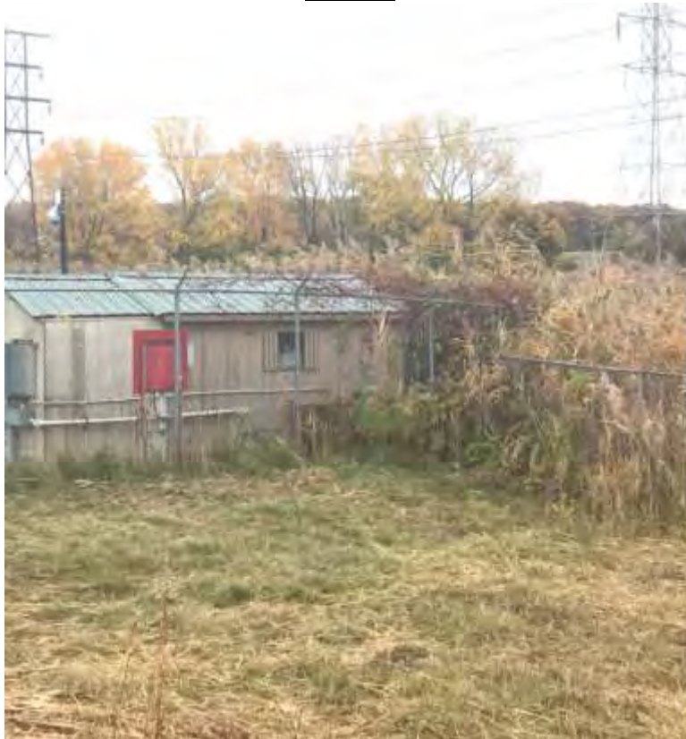
Southeast corner fencing, good condition 10/26/20 NWP
