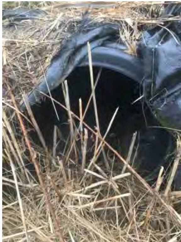
Surface water drainage culvert SW-1, undamaged
