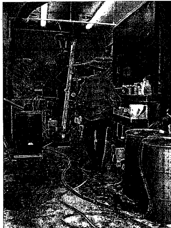
Photo 8: View of water/sludge being pumped to 55-gallon drums
