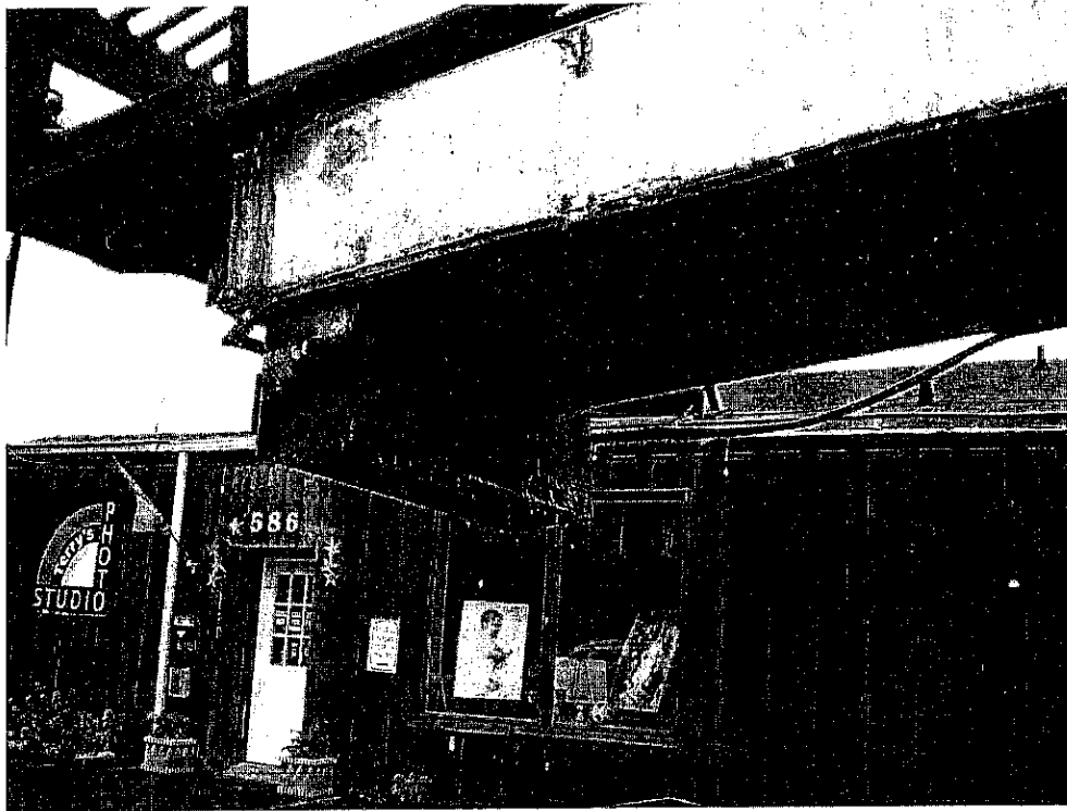
Photo 3: View of rust, calcium, and algae on bottom of tray
