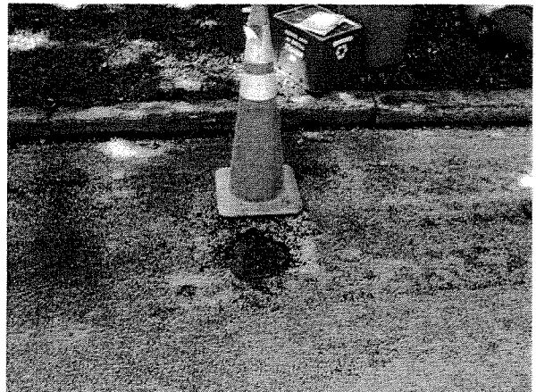
There appears to be no damage to this MW
