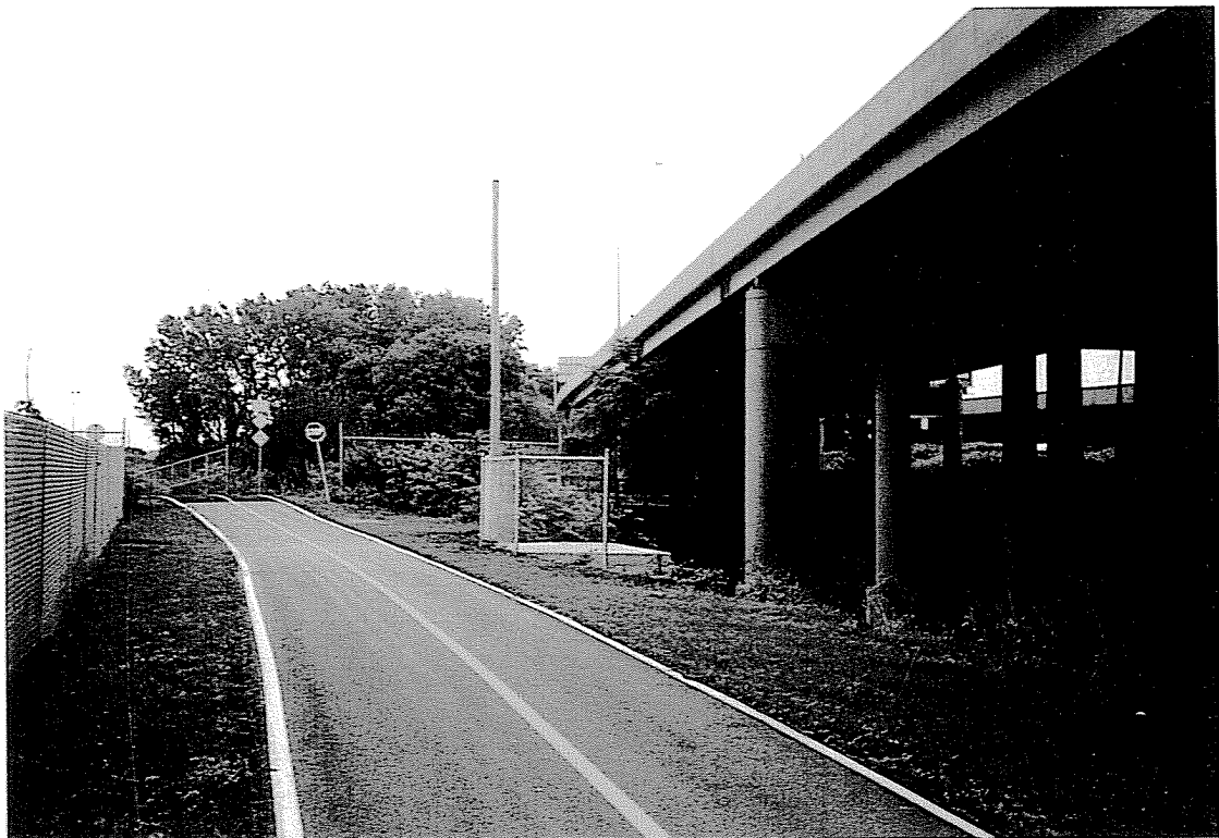
6B. Completed system (from south).
