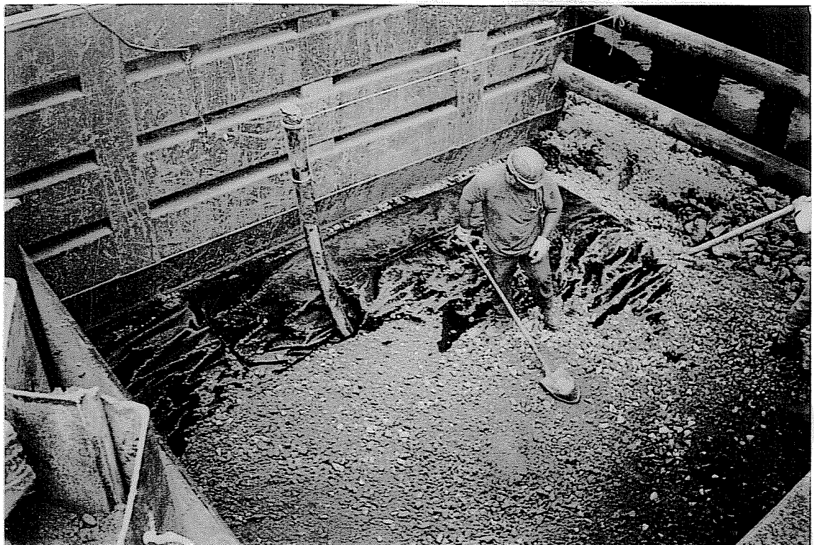
4B. Placing vault sub-base.
