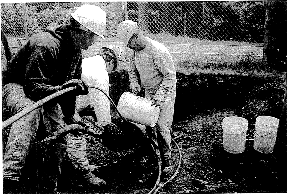
2B. Installing well materials.
