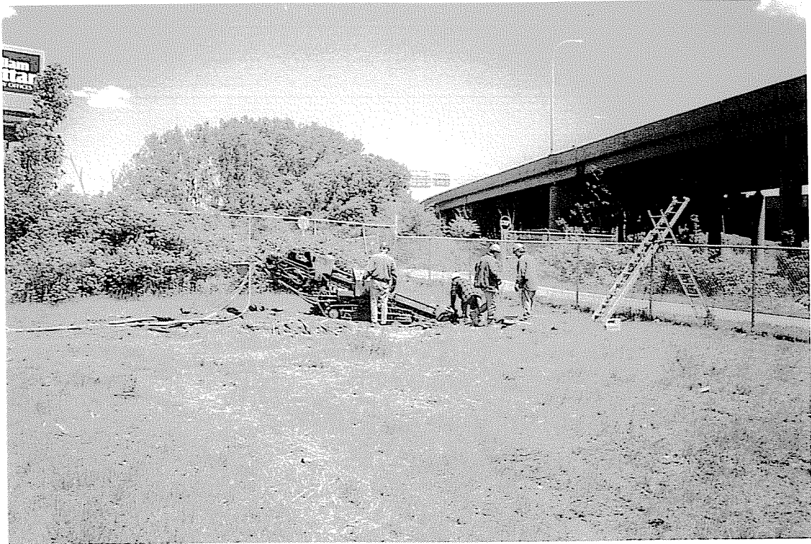
1A. Directional drilling to target area.
