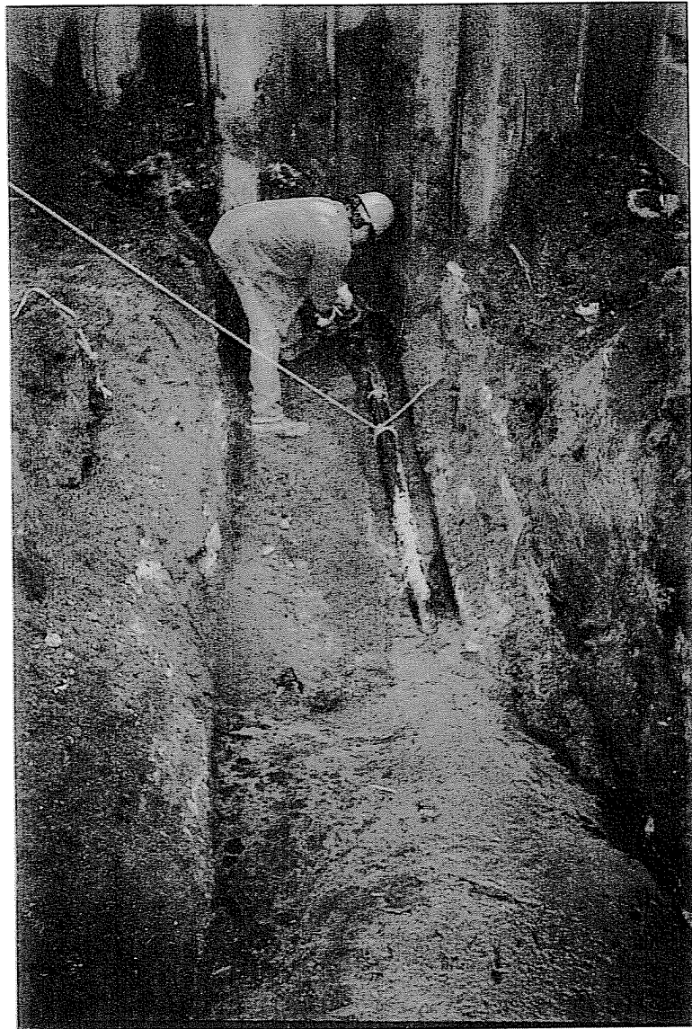
4A. Cutting HDPE pipe.
