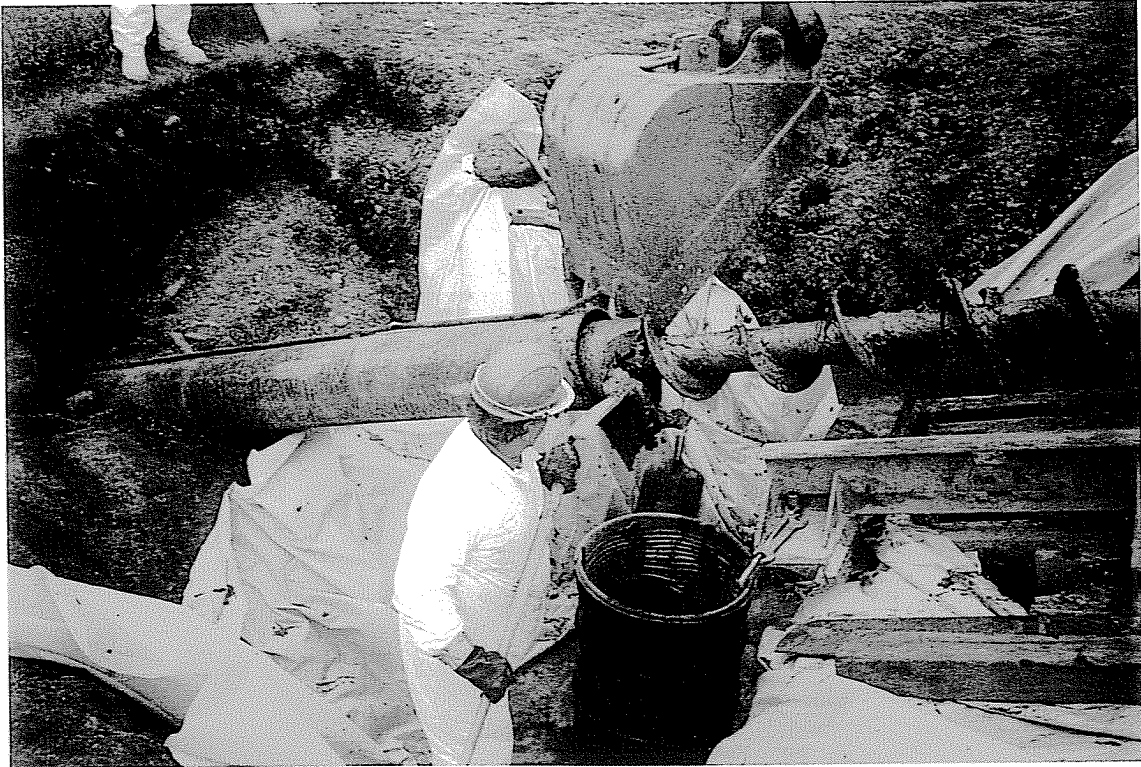
2A. Containerizing drill cuttings.
