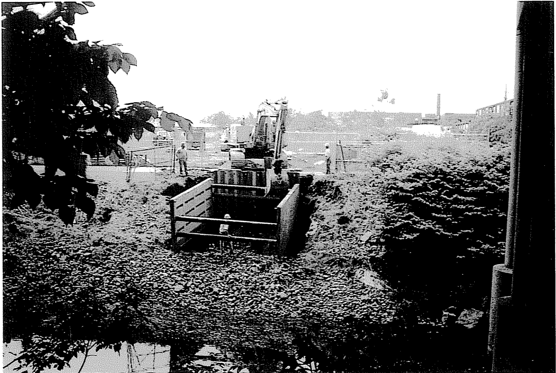
3B. Vault Excavation
