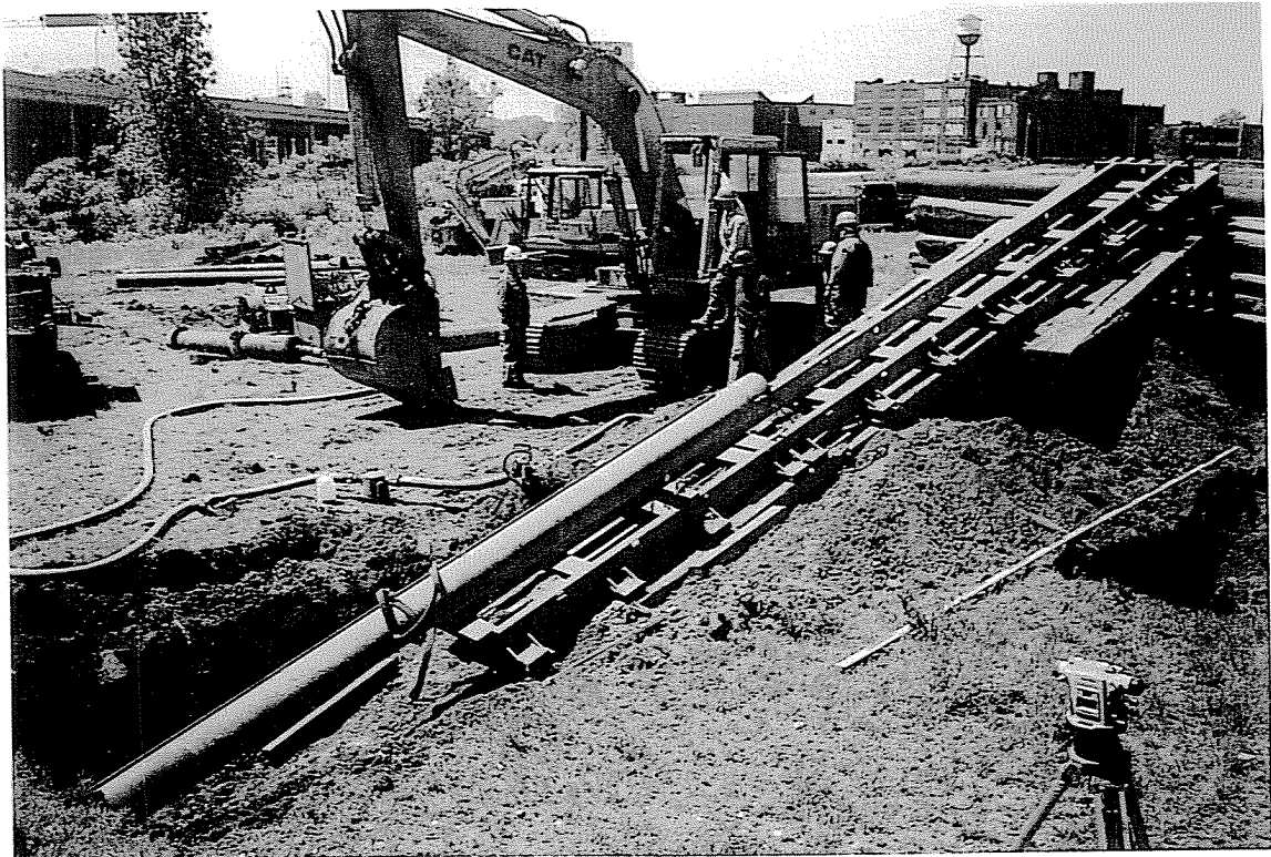
1B. Driving 12-inch casing over directional drill string.
