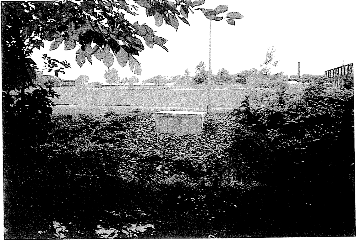
6A. Completed system (from east).
