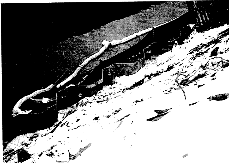
Figure 2 Top of wall prior to backfill
