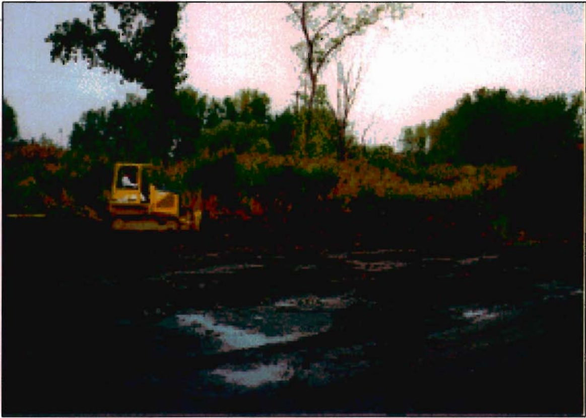
Grading restoration of excavated area (October 5, 2001).
