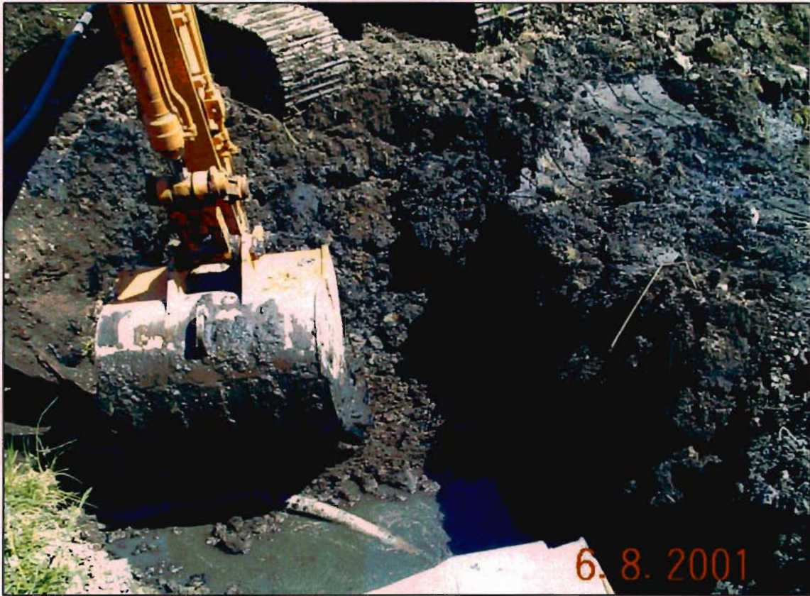
Excavation of sump for groundwater removal.
