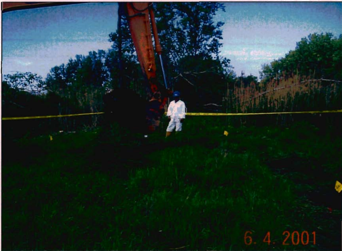
Excavation of cover soil.
