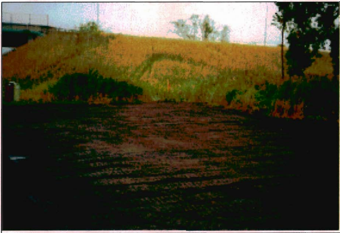
Completed site restoration (October 5, 2001).
