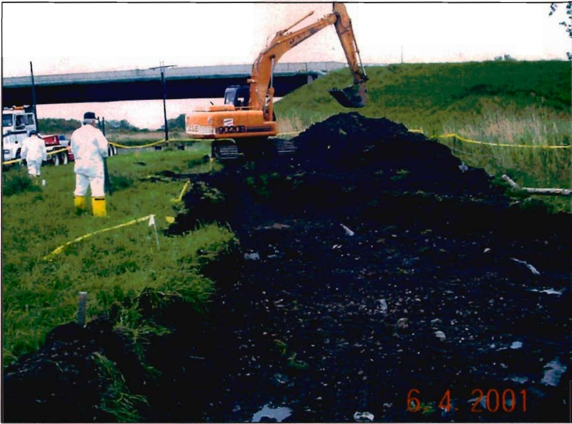
Stockpiling of cover soil for use as backfill material.
