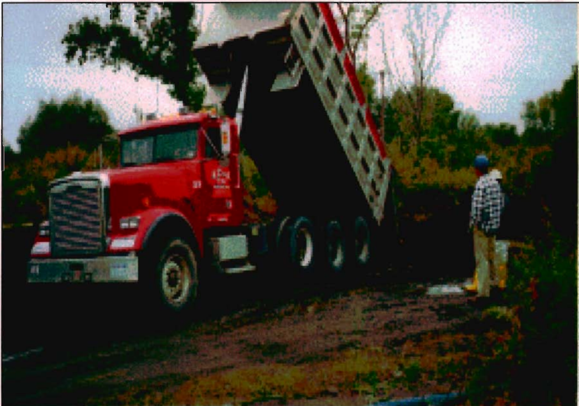
Transporting of backfill to site (October 5, 2001).
