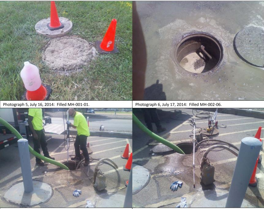
Photograph 7, July 24, 2014: Wand loosening sediment at CSMH-002. Photograph 8, July 24, 2014: Pumping sediment from CSMH-002.
