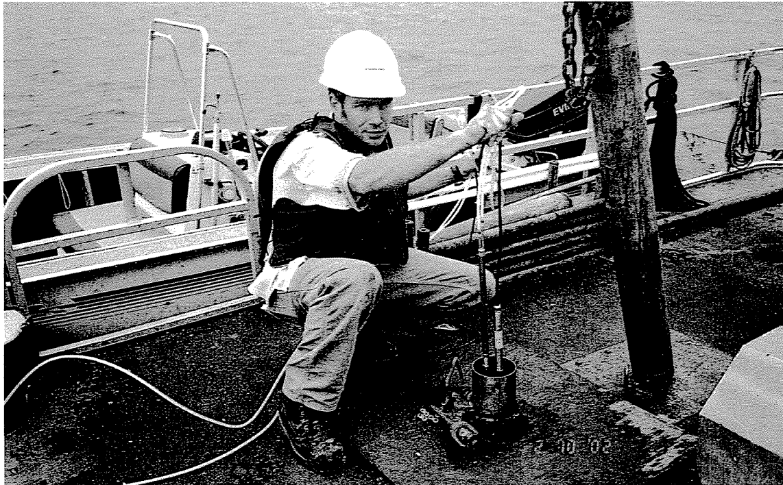
Photo No. 3. Vibrating wire piezometer and double valve pump were simultaneously lowered to depth.
