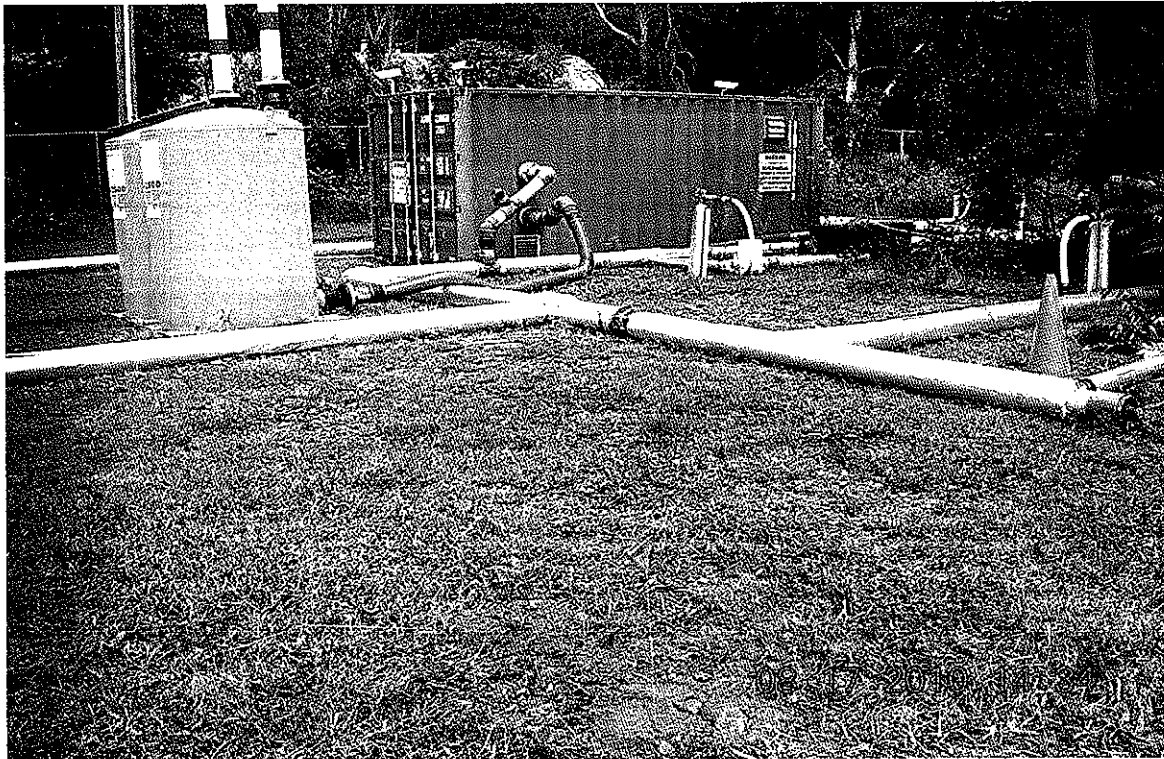
2. View facing north of Soil Sampling Location S-001-1824-0002.
