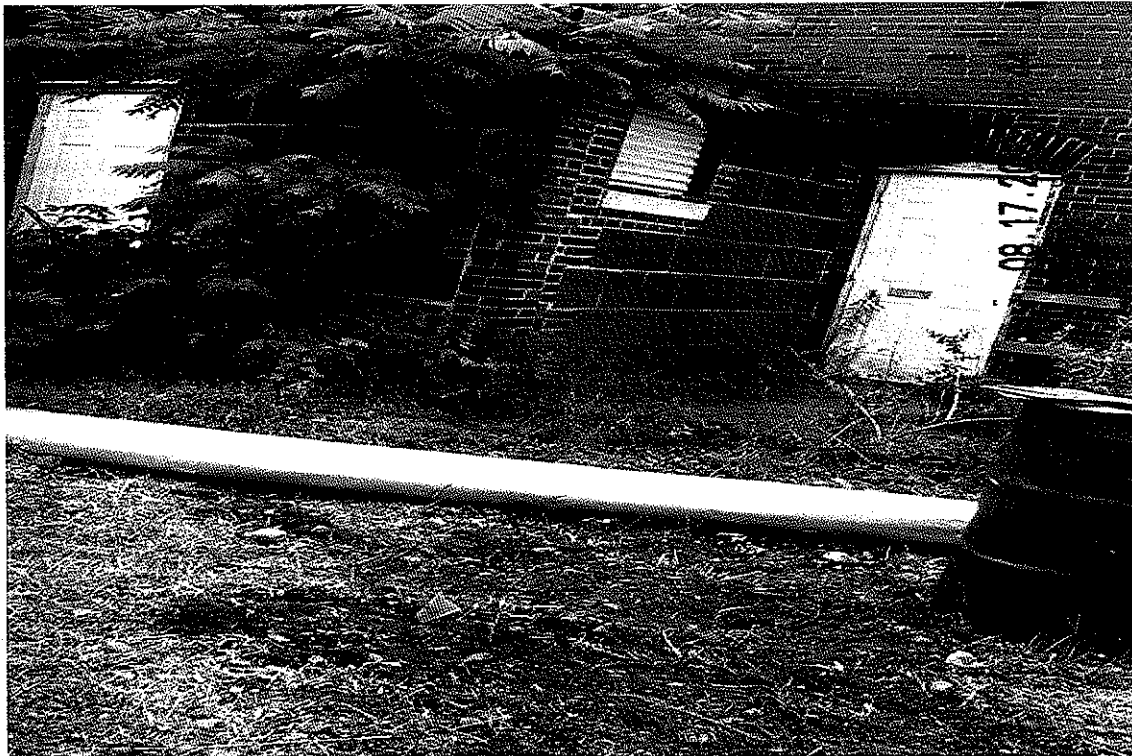
10. View facing southwest of Soil Sampling Location S-001-1824-0010/S-001-1824-0011 (Field Duplicate).
