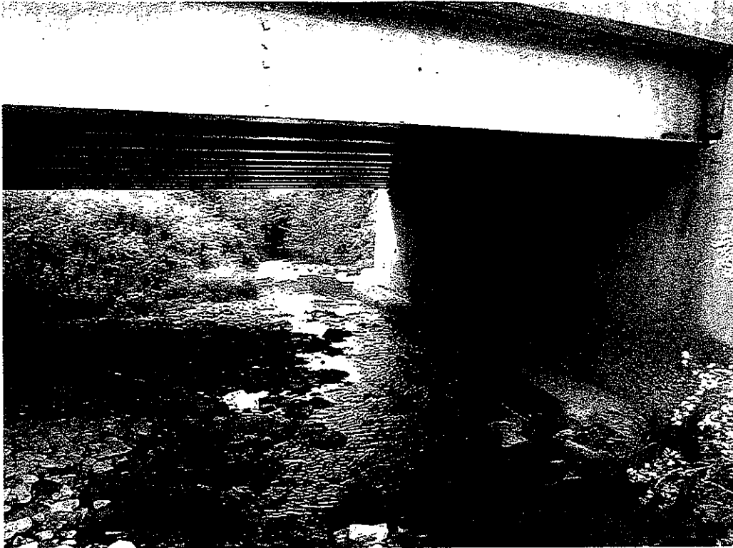
Site Number 5. Whig Street Creek at Rte. 353
