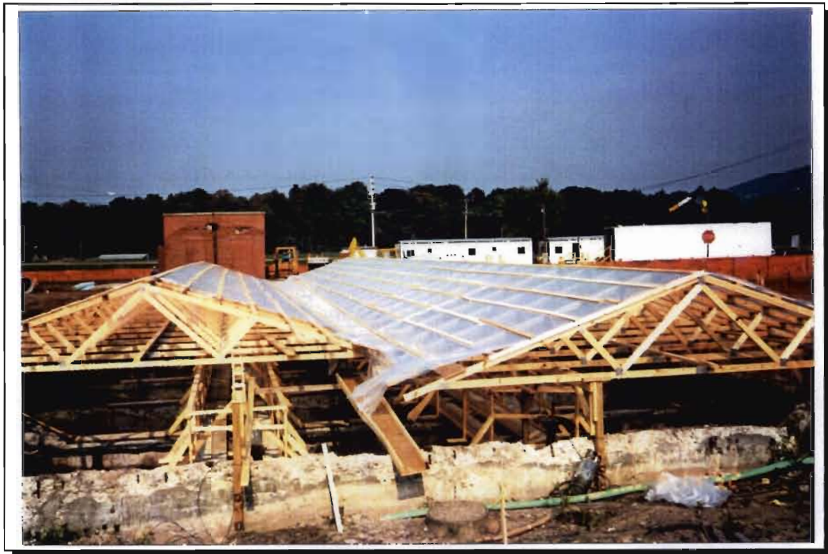
Photograph 3. Temporary access walkways and cover.
