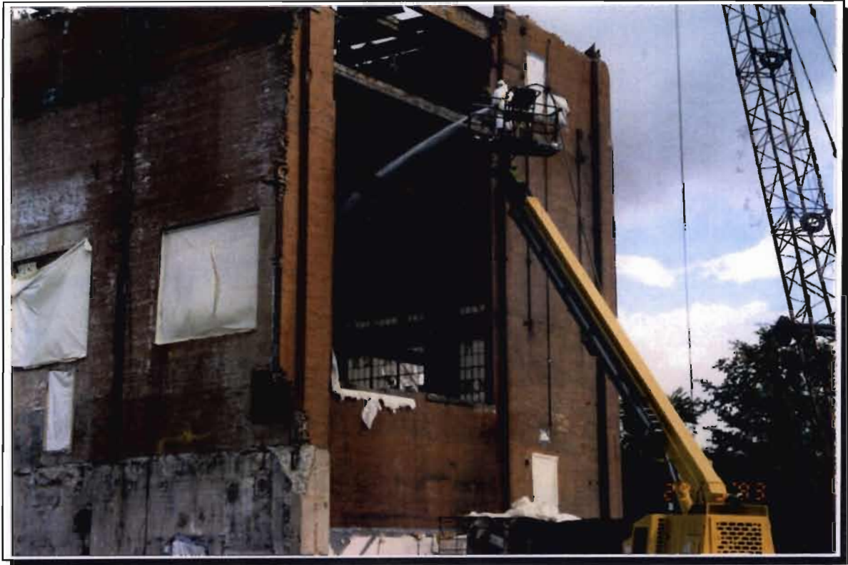
Photograph 7. Use of amended water to control dust.
