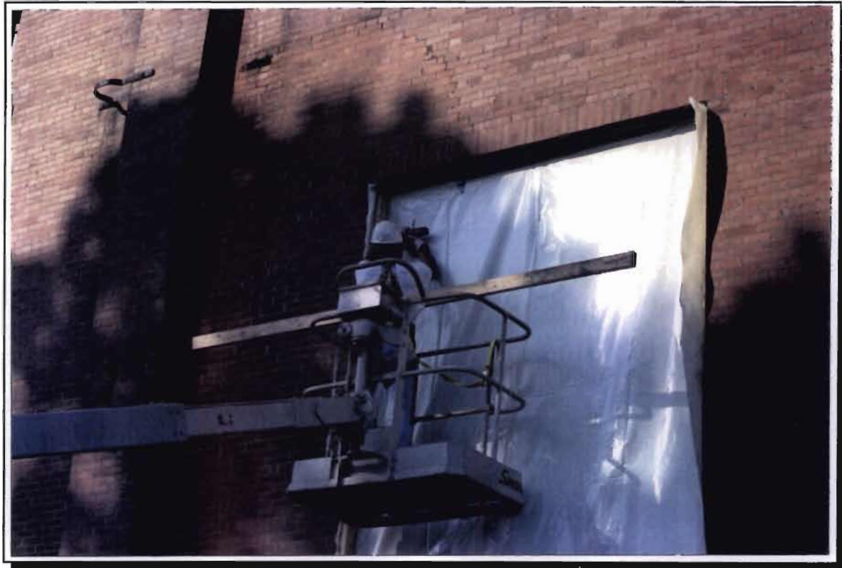
Photograph 4. Erecting plastic barriers over openings.
