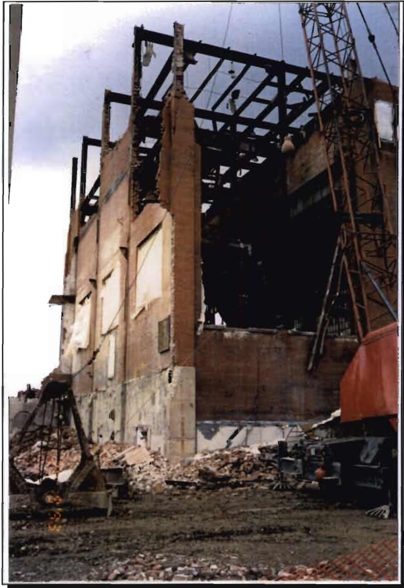
Photograph 6. Partial demolition of powerhouse.
