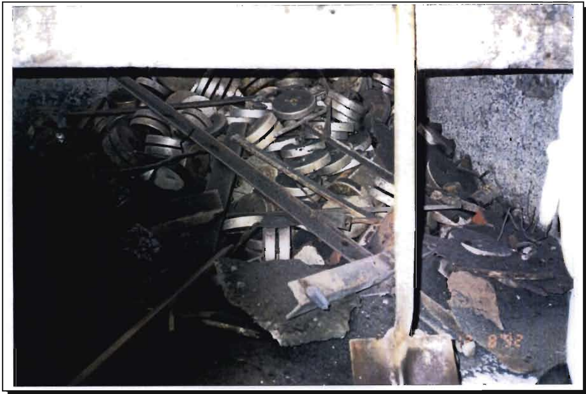
Photograph 10. Example of debris to be cleaned and left in separator.
