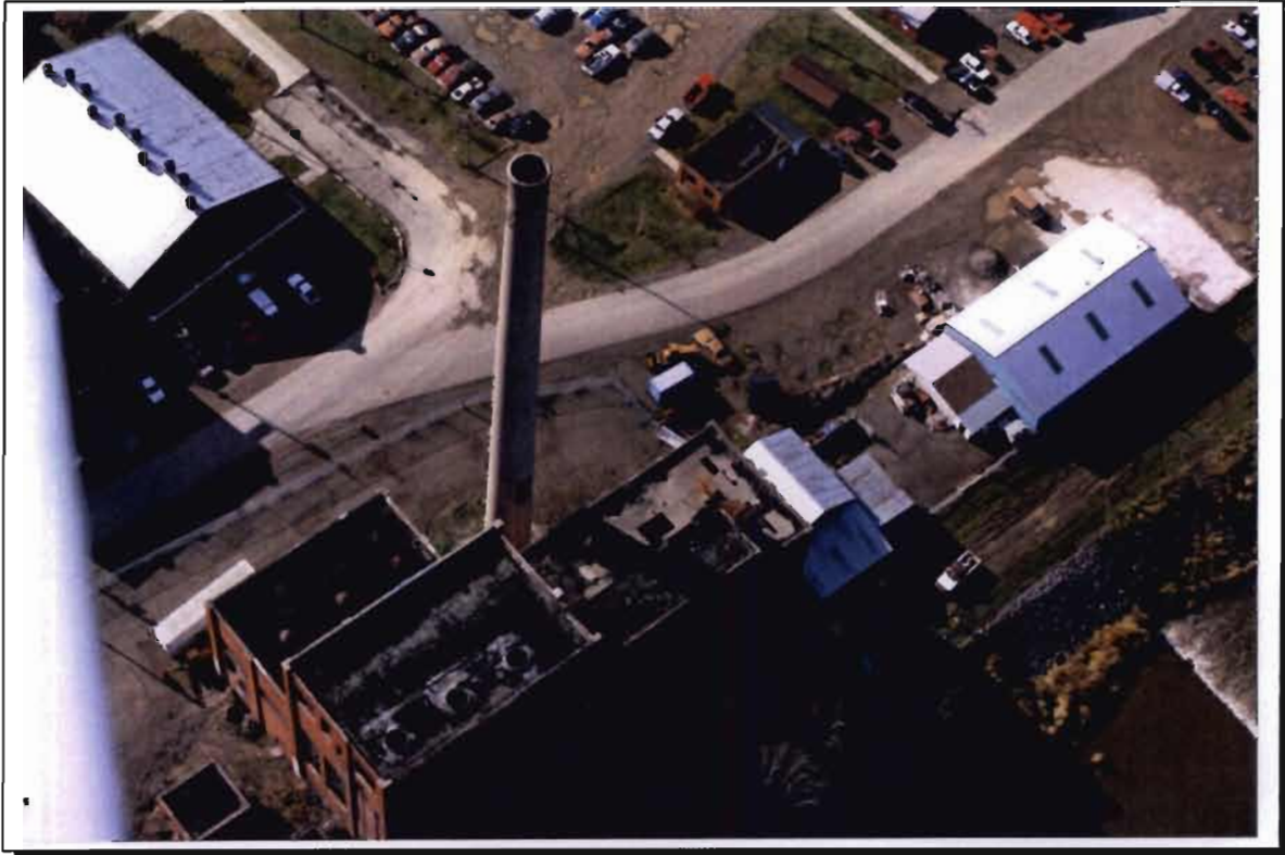
Photograph 1. General view of powerhouse, smokestack and small storage buildings.
