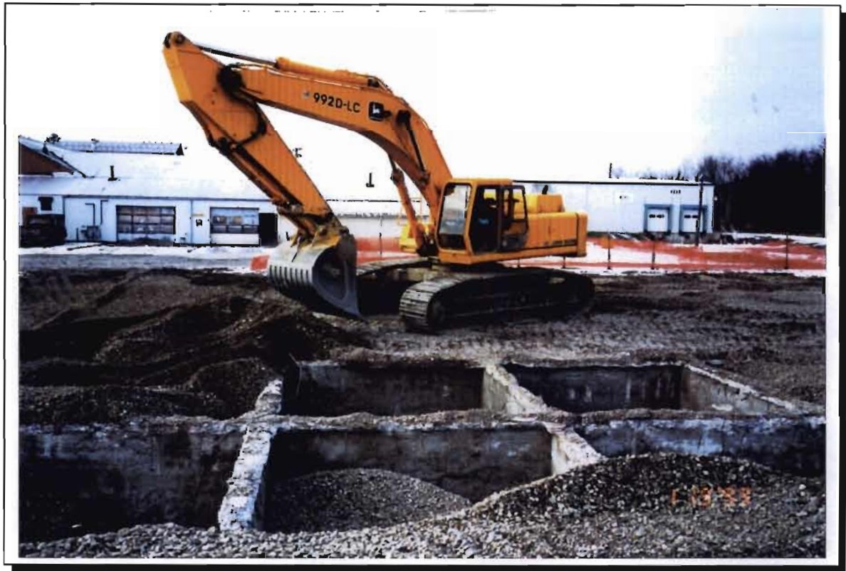
Photograph 12. Backfilling of separator with cell walls demolished below grade.
