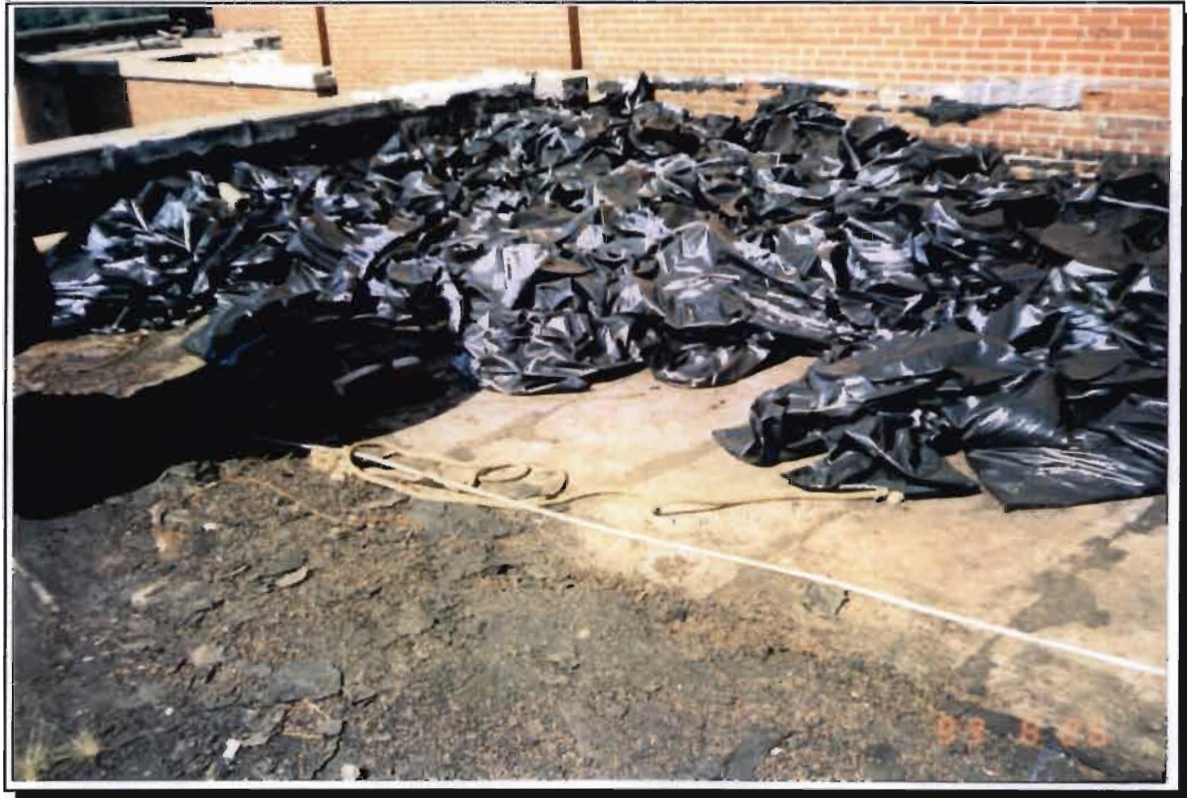
Photograph 5. ACM removal from turbine room roof.
