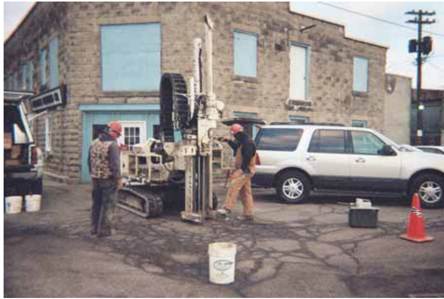
Date: 1/23/06 Subject: Direct-Push activities at the Former Liberty Street Dry Cleaners Site boring LS-BH-05 Photographer: Robert Meyers
