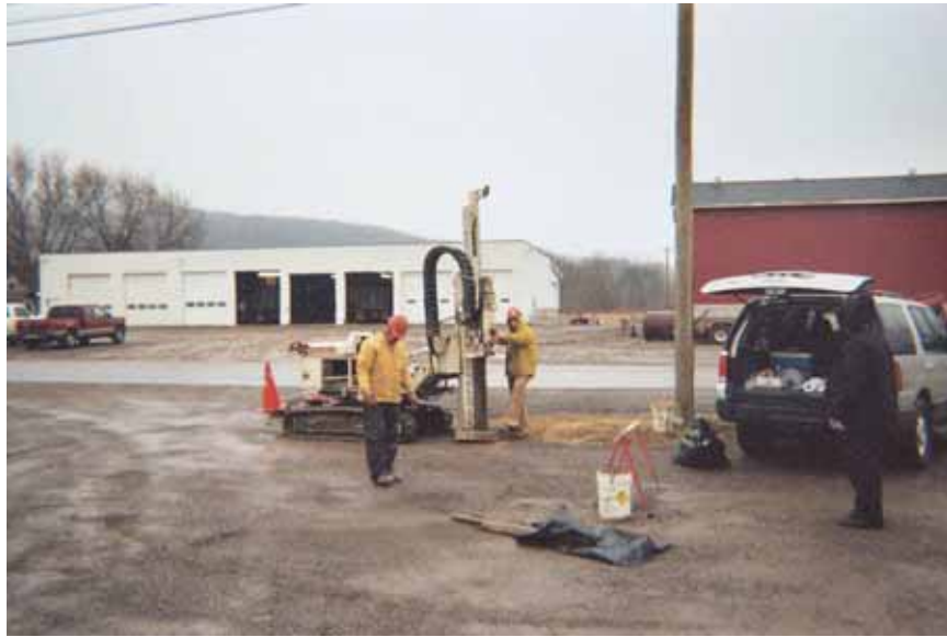
Date: 1/24/06 Subject: Direct-Push activities at the Canisteo Town Garage Site boring TG-BH-04 Photographer: Stephanie Reynolds Smith
