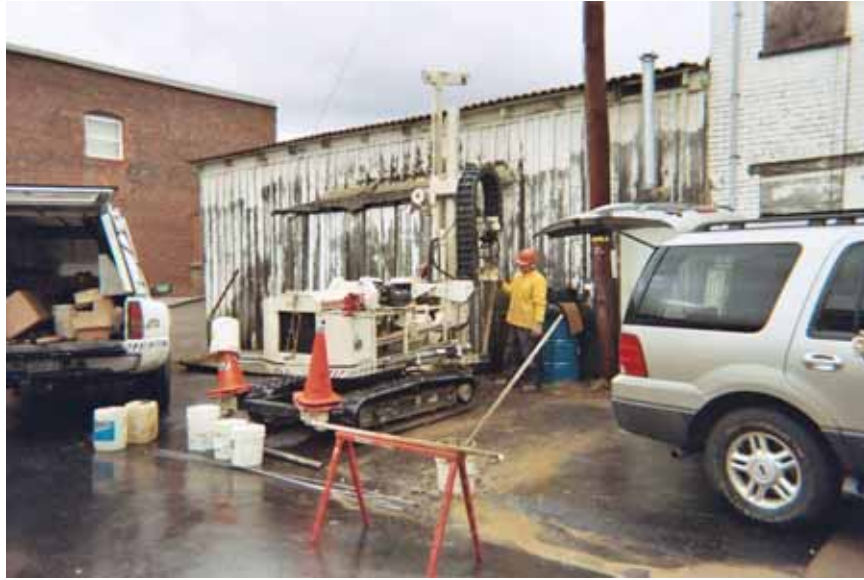
Date: 1/23/06 Subject: Direct-Push activities at the Former Liberty Street Dry Cleaners Site boring LS-BH-03 Photographer: Robert Meyers
