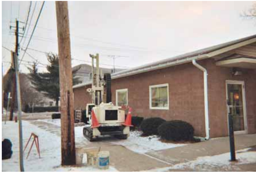
Time/Date: 1/26/06 Subject: Direct-Push activities at the Former Depot Street Dry Cleaner Site boring DS-BH-06 Photographer: Stephanie Reynolds Smith
