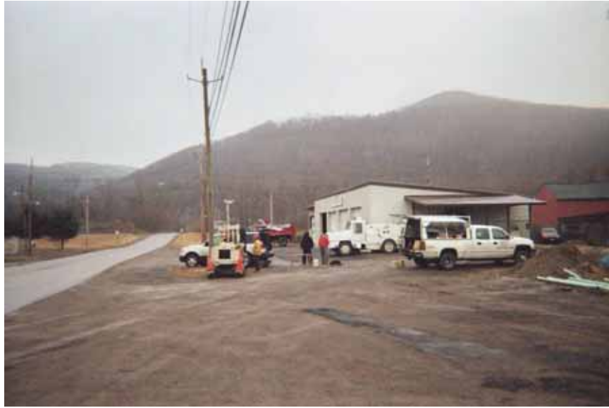
Date: 1/24/06 Subject: Direct-Push activities at the Canisteo Town Garage Site boring TG-BH-03 Photographer: Robert Meyers
