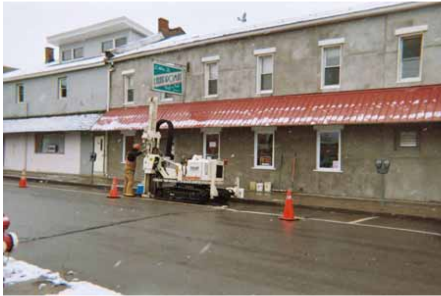
Date: 1/23/06 Subject: Direct-Push activities at the Former Liberty Street Dry Cleaners Site boring LS-BH-06 Photographer: Robert Meyers
