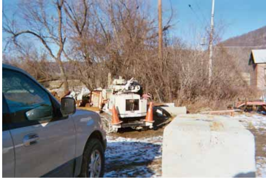
Date: 1/24/06 Subject: Direct-Push activities at the Canisteo Town Garage Site boring TG-BH-01 Photographer: Stephanie Reynolds Smith
