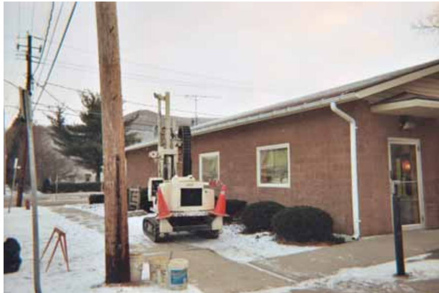
Time/Date: 1/26/06 Subject: Direct-Push activities at the Former Depot Street Dry Cleaner Site boring DS-BH-06 Photographer: Stephanie Reynolds Smith
