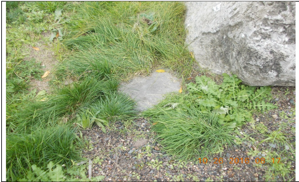
Animal burrow filled in with concrete.
