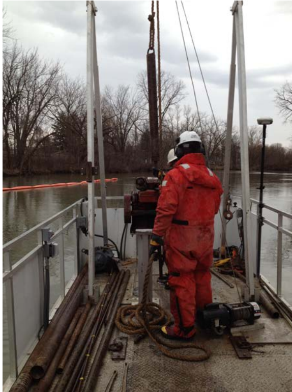
Typical Cat Head Split Spoon Sampler – Safety Method
