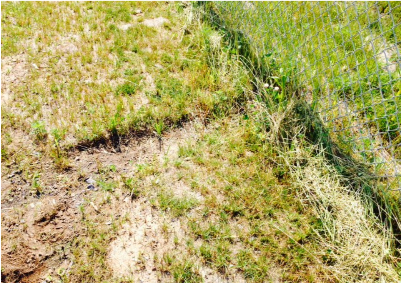
Photo 13 - Minor Erosion Near Edge of Asphalt Cap
