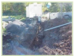
E & E directed the excavation and disposal of 2,800 tons of TCE-contaminated soil.
