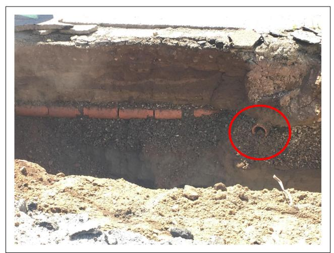
Photo #13: Photo taken during the original excavation with a lateral pipe shown on the western side of the excavation. Former Erwin Cleaners December 18, 2018
