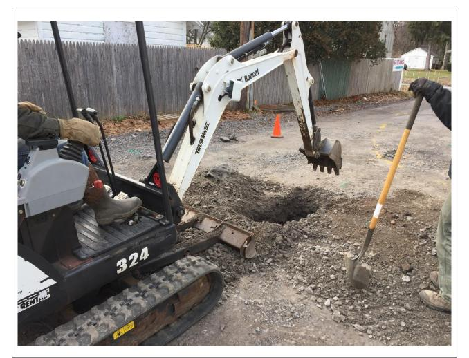
Photo #15: Excavation of Test Pit 2. The goal of this pit was to find evidence of a probable pipe seen with the GPR. The test pit was dug to the western edge of the original excavation, but the pipe was not found. Former Erwin Cleaners December 18, 2018
