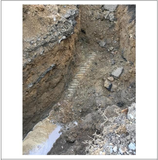
Photo #21: Approximate location of the last detection of the probe. Evidence suggests a blockage is here, though the pipe is intact and does not appear damaged. Former Erwin Cleaners December 18, 2018
