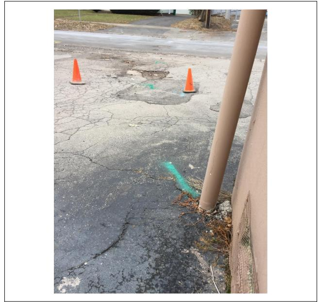
Photo #10: Investigation of a pipe that was discovered by Parsons during a previous investigation where the pipe was found to be connected to the stormwater sewer. Probing determined that the line was connected to a stormwater drain on the neighboring building. Former Erwin Cleaners December 18, 2018
