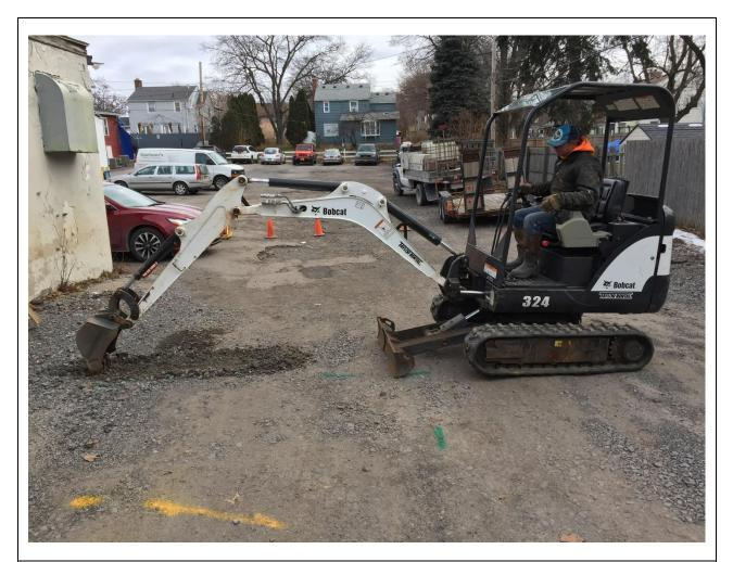
Photo #12: Excavation of Test Pit 1. The goal of this was to find a pipe previously seen in photographs of the initial excavation to confirm its status (See Photo #13). Former Erwin Cleaners December 18, 2018
