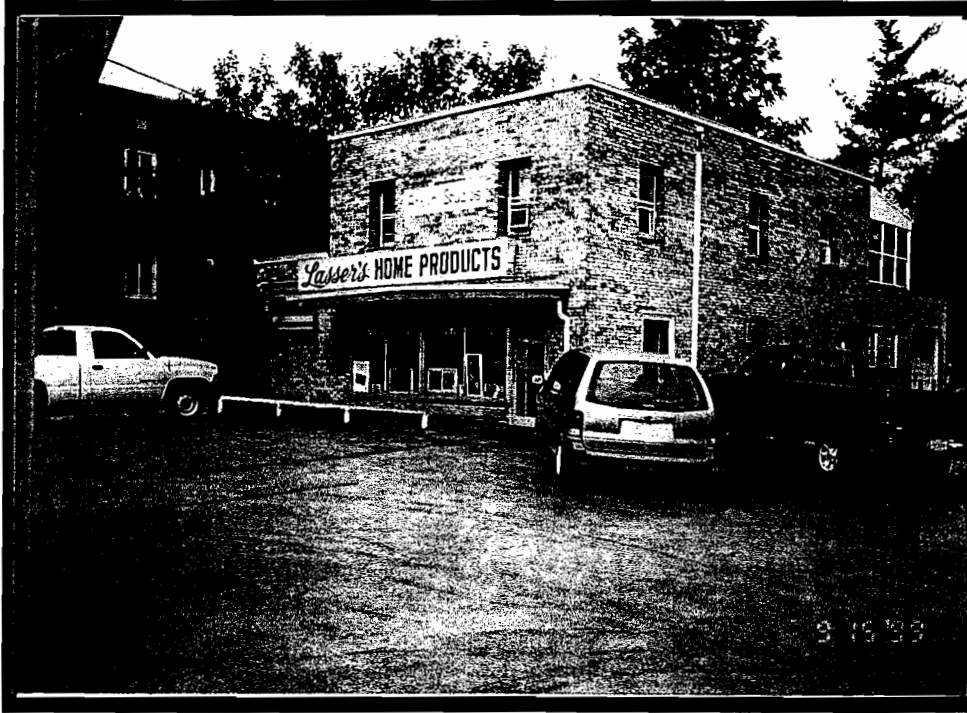
View of the Site
