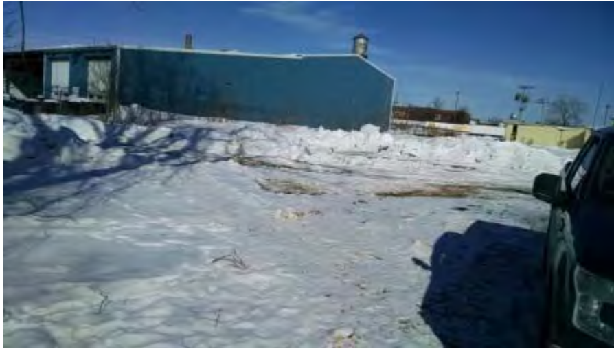
March 6, 2015 - View northeast, work area after soil bins have been removed.
