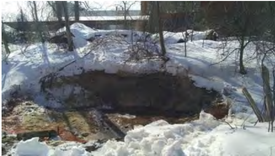
March 6, 2015 - View west, post excavation after site cleanup, excavation has filled with water.
