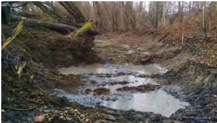
December 3, 2014 - View south, excavation backfilling with water.
