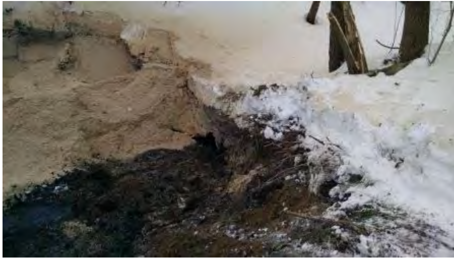
March 4, 2015 - View west, north side of excavation after adding sawdust.
