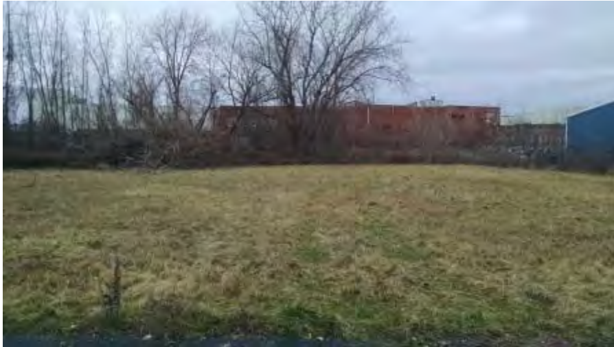
December 1, 2014 - View west, pond excavation area and staging area prior to beginning work.
