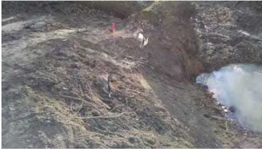
December 4, 2014 - View south, culvert showing the eastern edge of the excavation.
