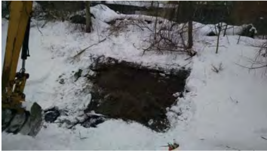
March 3, 2015 - View west, post excavation barrier.
