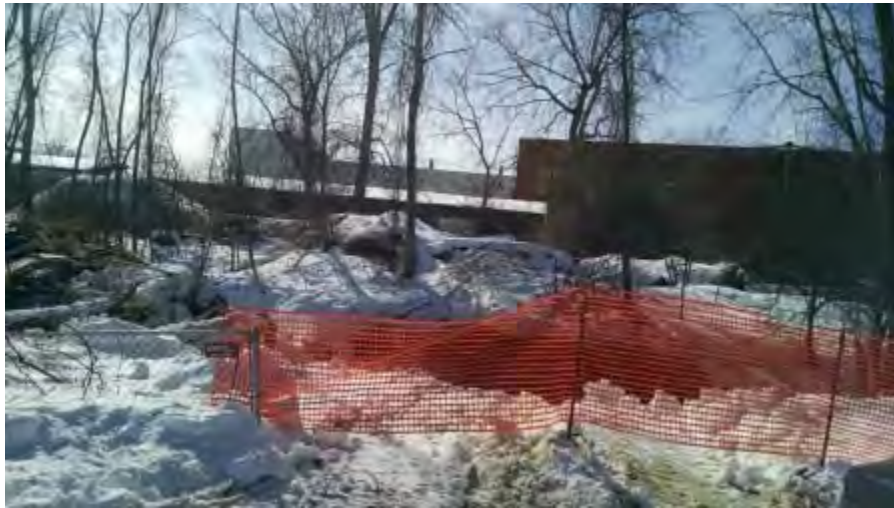
March 6, 2015 - View west, post excavation with barrier.
