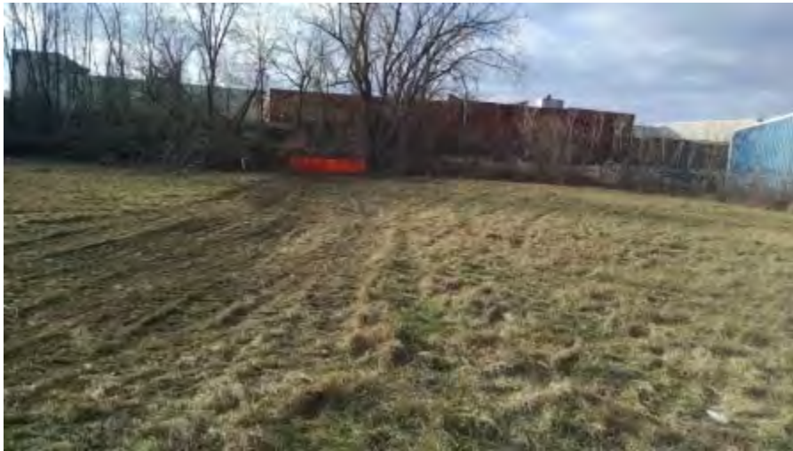
December 4, 2014 - View west, post excavation after site cleanup.
