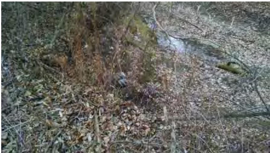
December 1, 2014 - View south, culvert in the center of the photo marks east edge of excavation area.
