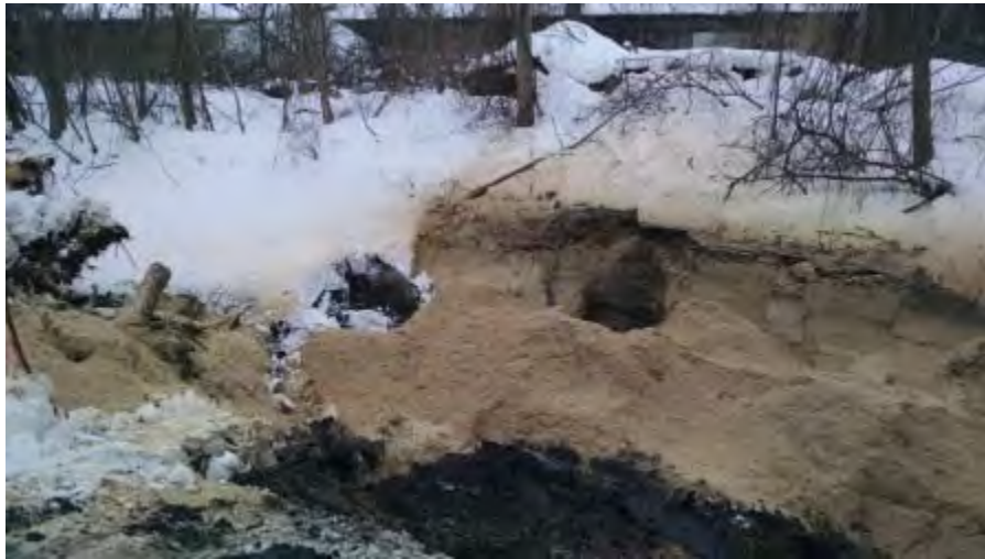
March 4, 2015 - View southwest, excavation after adding more sawdust.
