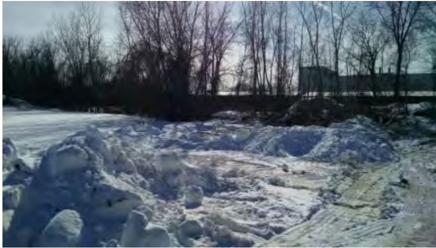
March 6, 2015 - View southwest, staging area after excavators were removed from site.
