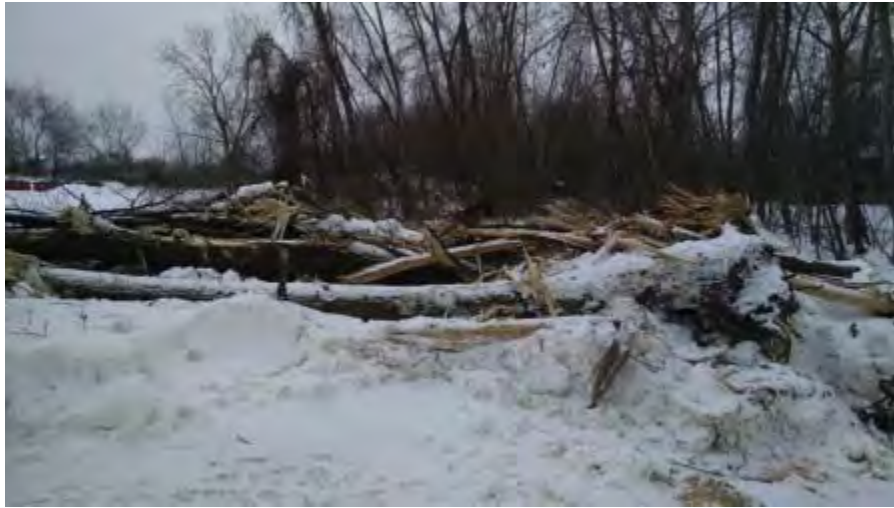
March 5, 2015 - View south, trees removed for access to sump pond.
