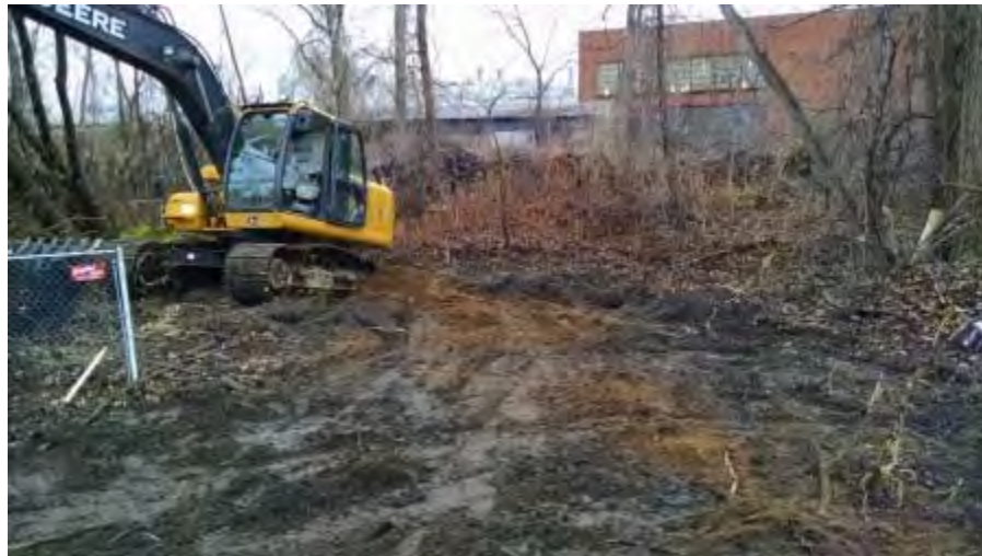
December 3, 2014 - View west, excavator cleared vegetation to allow access to excavation.
