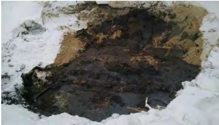
March 4, 2015 - View west, excavation after sawdust has been mixed in.
