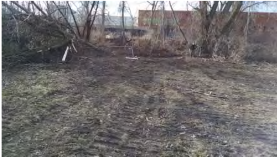
December 4, 2014 - View west, post excavation work area.
