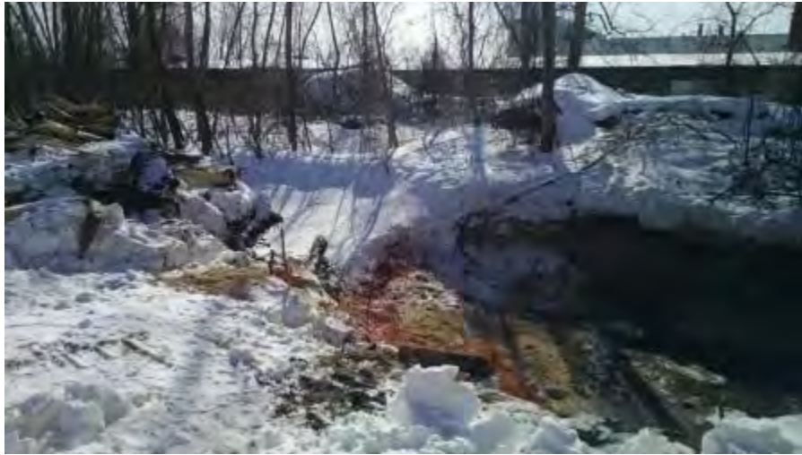
March 6, 2015 - View southwest, post excavation after removal of equipment.
