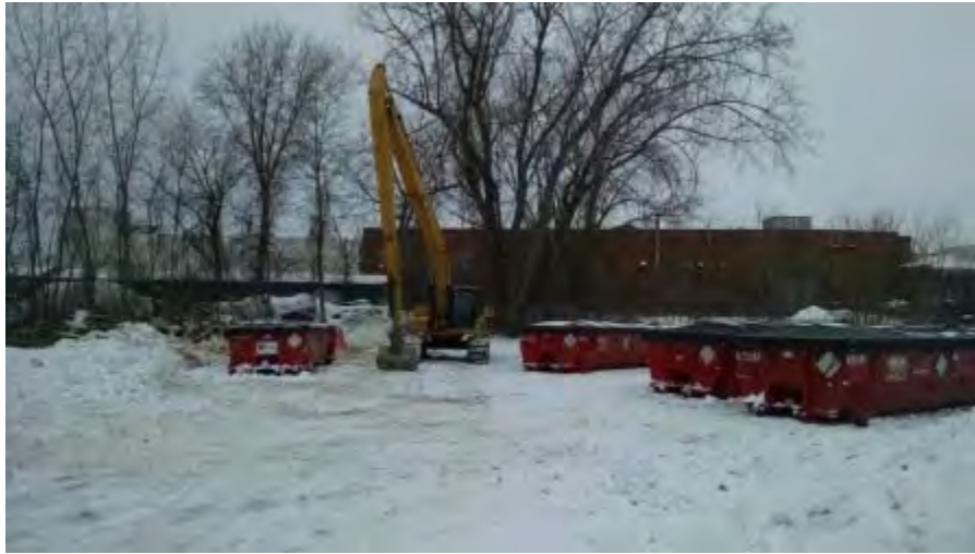
March 5, 2015 - View west, work staging area with soil bins.
