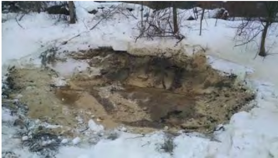
March 5, 2015 - View west, more sawdust added to excavation.
