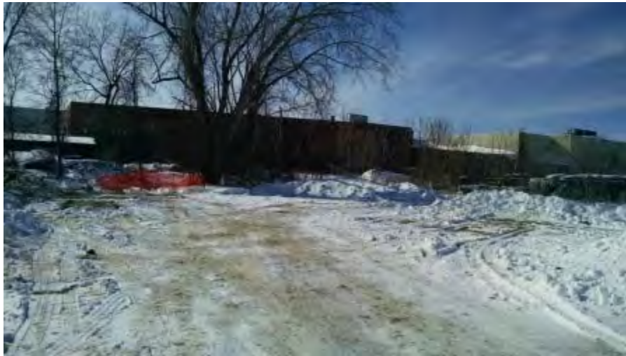
March 6, 2015 - View west, staging area after soil bins have been removed from site.
