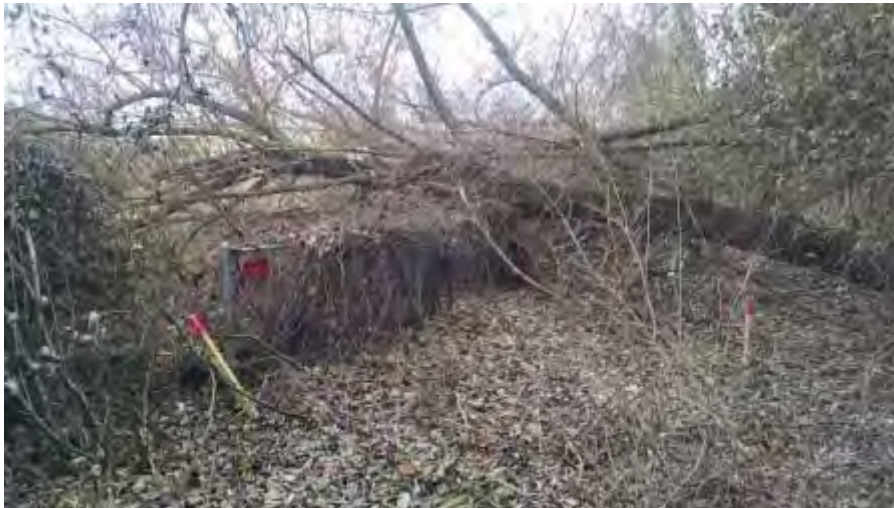
December 1, 2014 - View southeast, fence marks the southern edge of work area.
