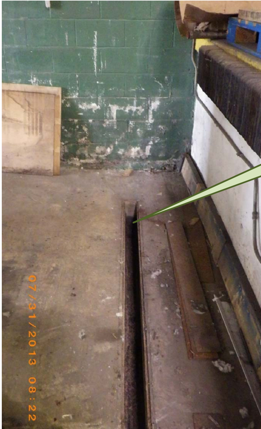
Trench Drain in Loading Dock – Location of 2-Inch Drain Pipe
