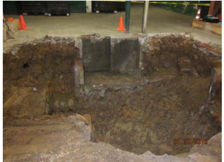
Photograph of southern portion of the vapor degreaser left in place.
