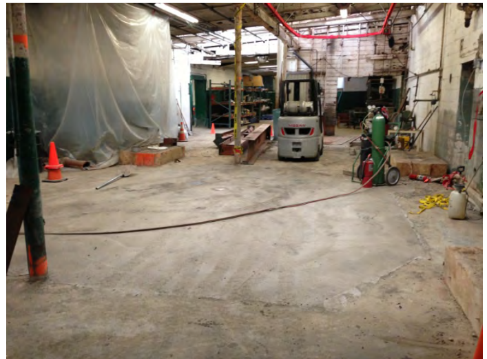
Photographed of excavation completed with concrete.
