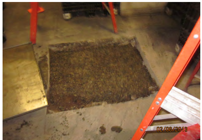
Photograph of small excavation near SB-9 partially backfilled.
