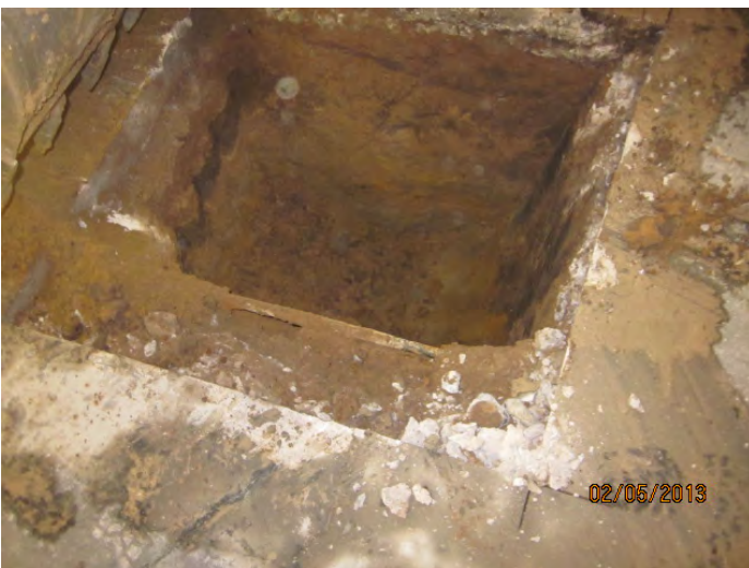
Photograph of small excavation near SB-9
