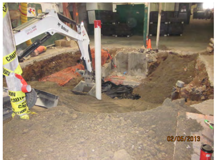
Photograph of backfill activities.
