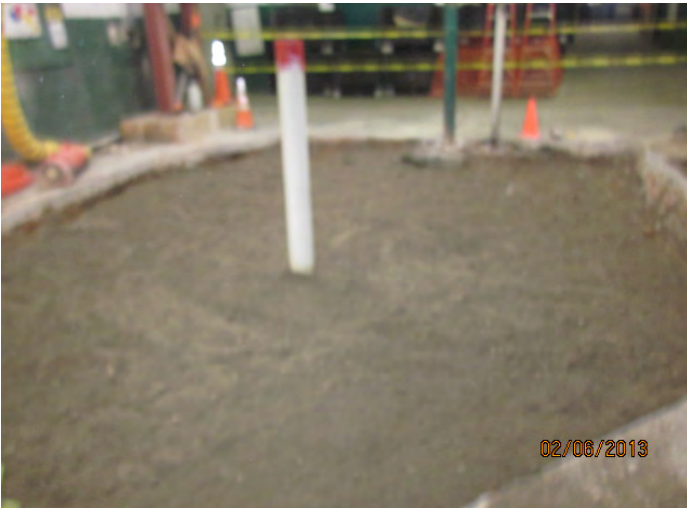
Photograph of backfilled excavation and well riser.
