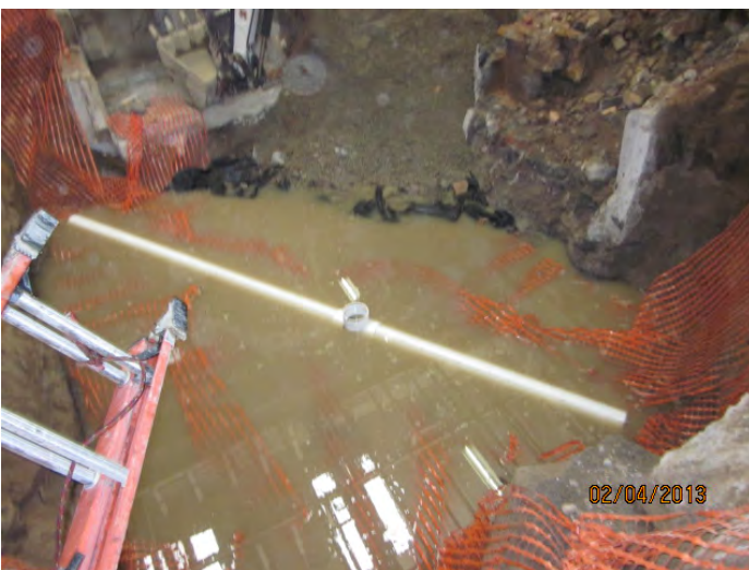
Photograph of horizontal injection well placed into excavation.
