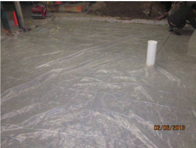
Photograph of backfilled excavation and well riser.
