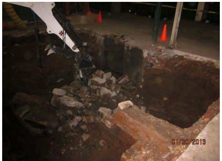
Photograph of jackhammer dismantling the southern portion of the former vapor degreaser.
