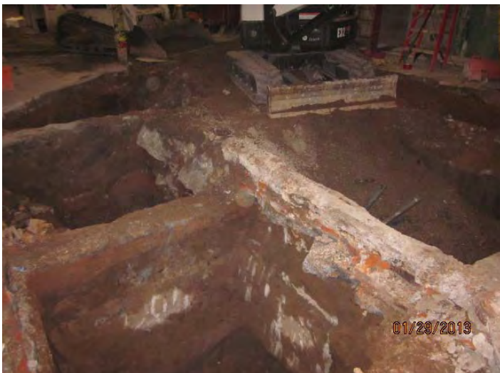
Photograph of west side of former vapor degreaser pit with concrete supports to the west.
