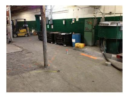
d. Excavate and stockpile impacted soils to the target excavation depth of 8-ft below the top of the concrete floor as directed by the Engineer . *See photographs below for illustration of overall excavation area.*
