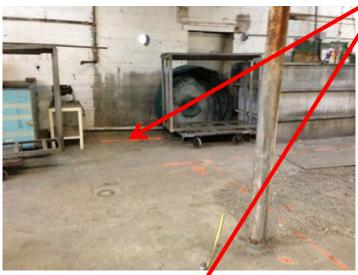
Location of Temporary Steel H-Columns to maintain 20.5-ft and 26.5-ft beam spans (spacing between the existing live electrical panels and temporary column locations can be increased as needed by reducing temporary beam length, up to 2ft can be reduced, i.e., install 24.5-ft temporary beams)
