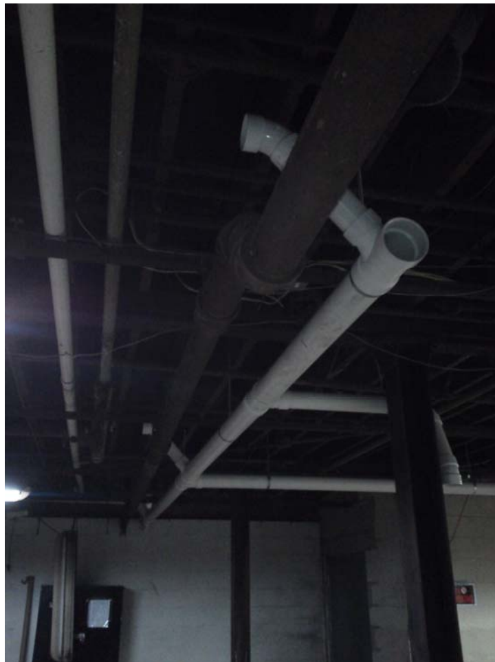
Main header in main room. Legs shown (back of picture to front): SP6, SP11, Header to SP1-SP4, SP7, SP5 and SP8/SP12
