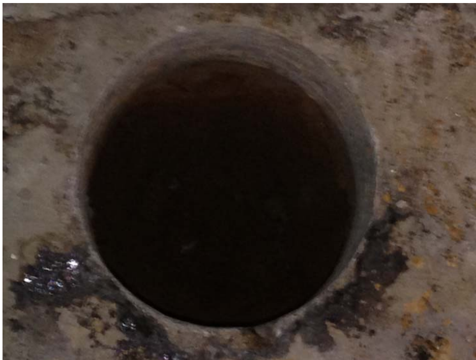
Typical core drill hole for suction points, pre-soil removal. #2
