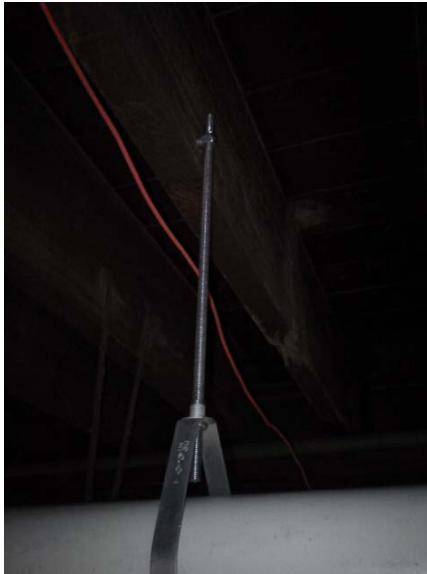
System 2 (Main System) header supported via pipe hanger, anchored to floor joist.
