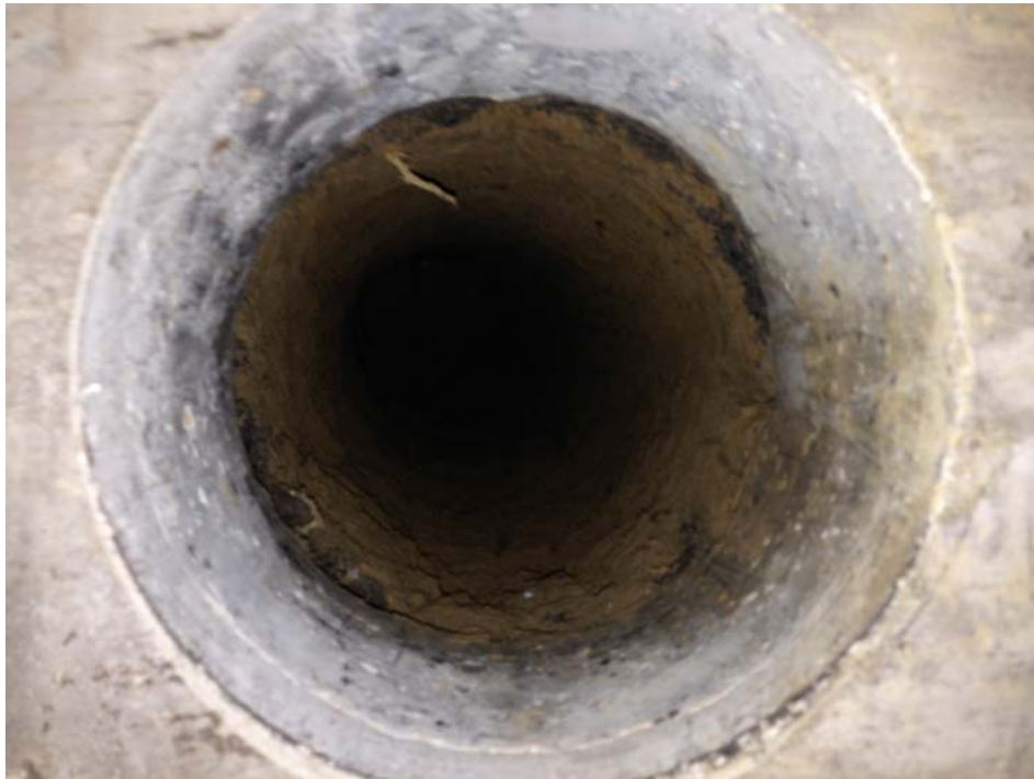
Typical core drill hole for suction points, pre-soil removal.
