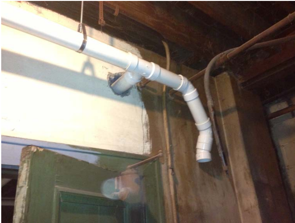
SP4 branching off header.
