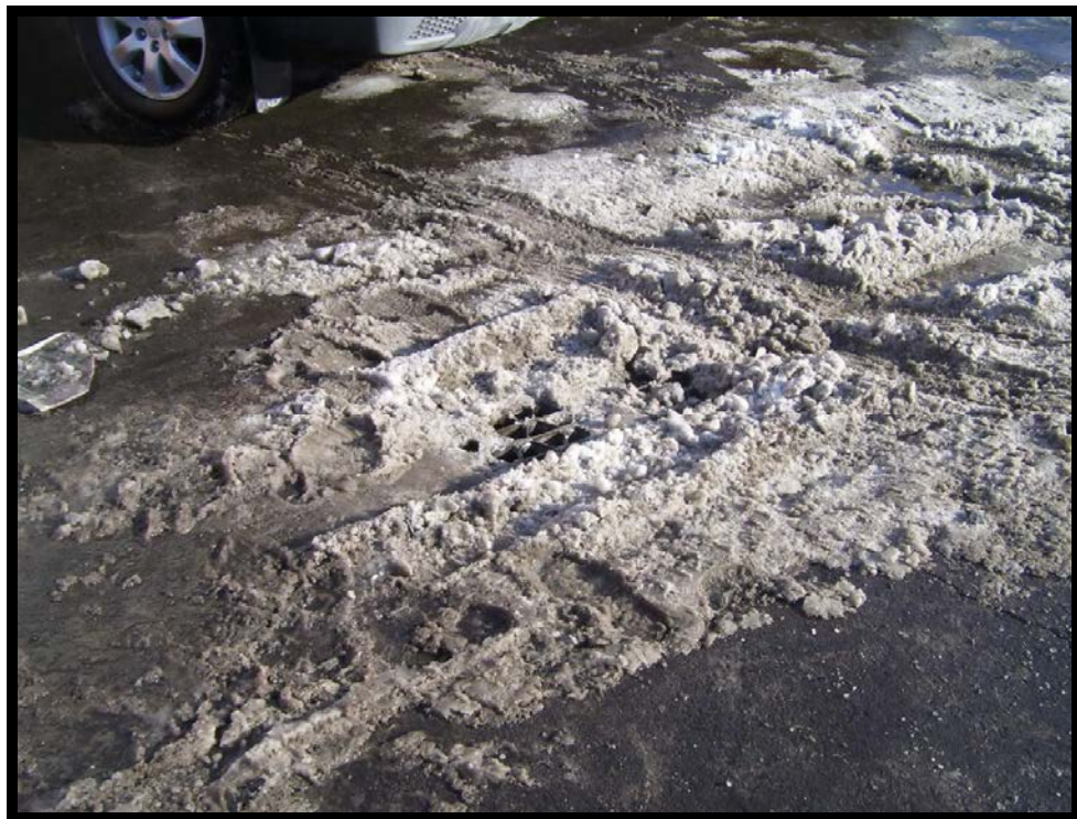
Location #104 – Exterior catch basin
