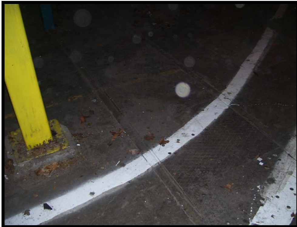
Location #30 – Trench drain
