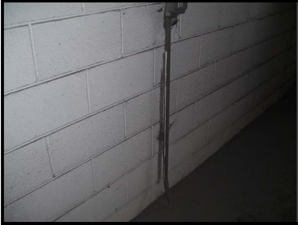
Location #68 – Utility conduit
