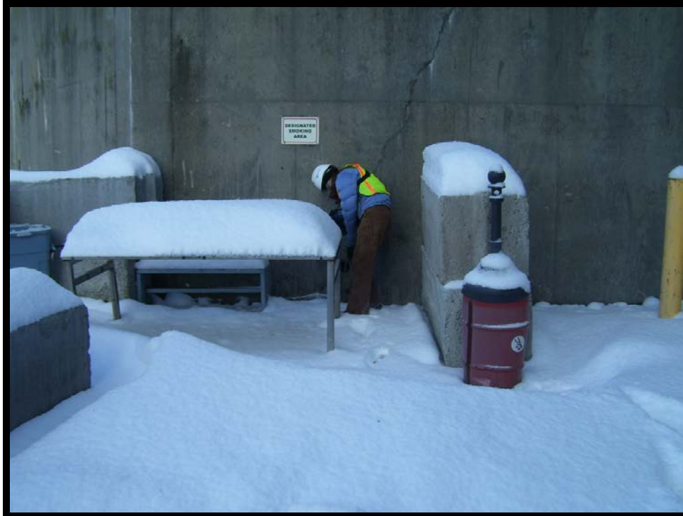
Location #108 – Retaining wall drain
