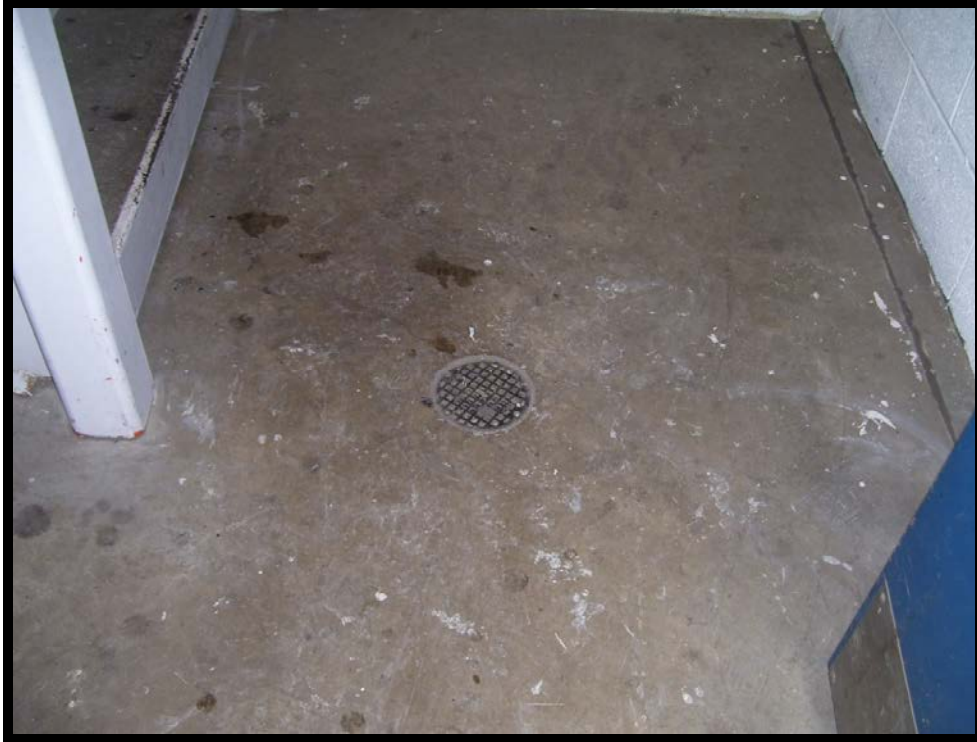
Location # 9 – Floor drain in stairwell
