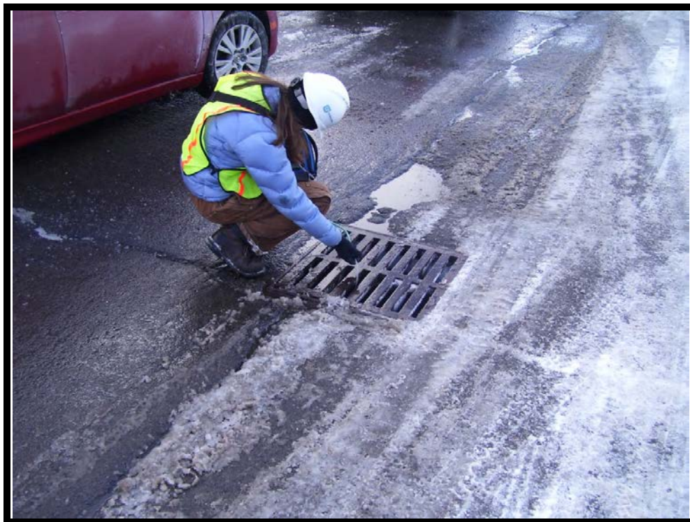
Location #109 – Exterior catch basin
