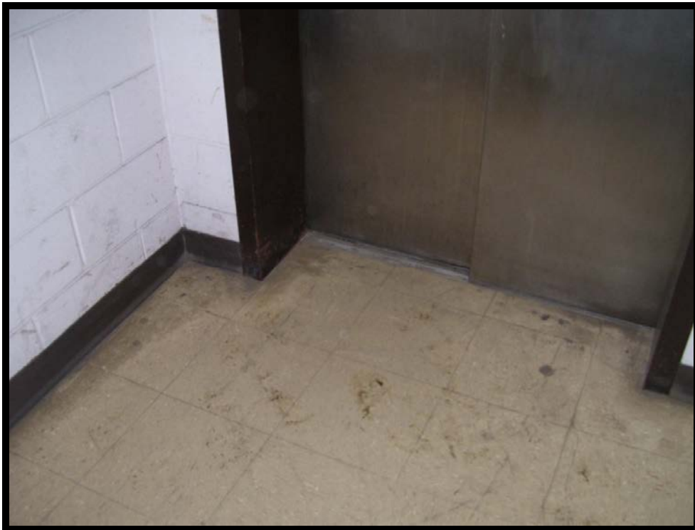
Location #10 – Bottom of elevator (not operational)
