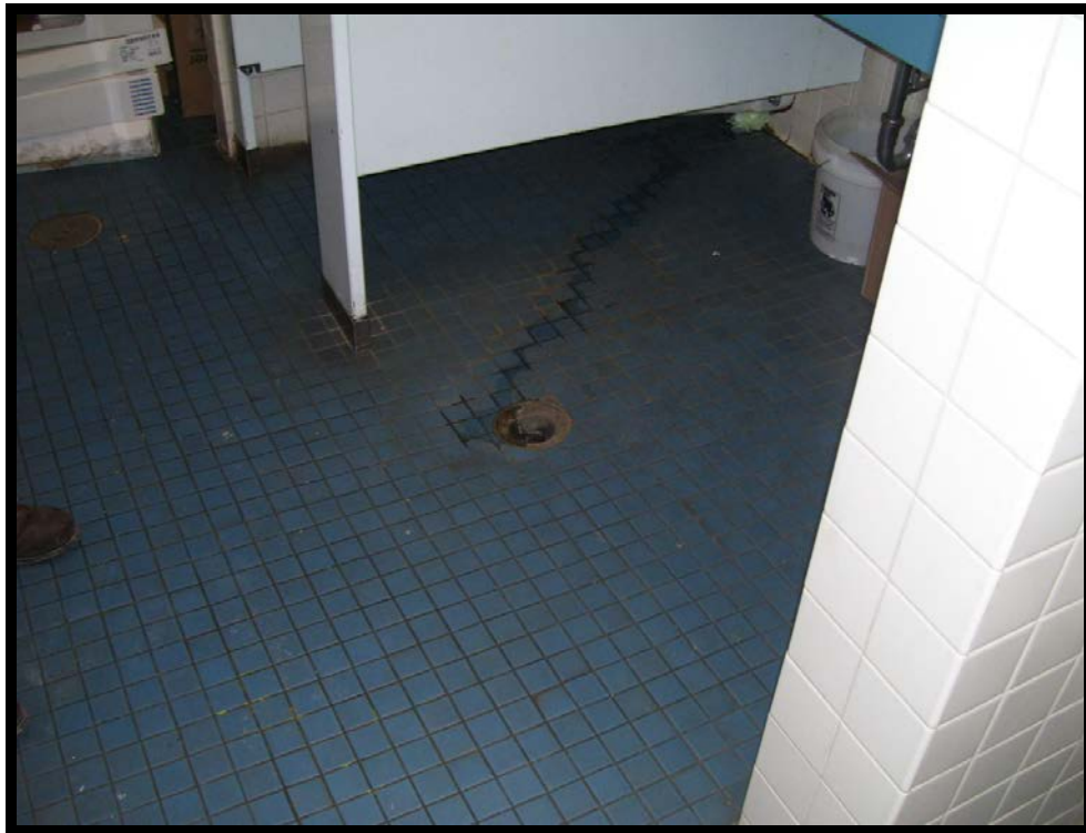
Location #91 – Floor drain ladies room (office area, base floor)
