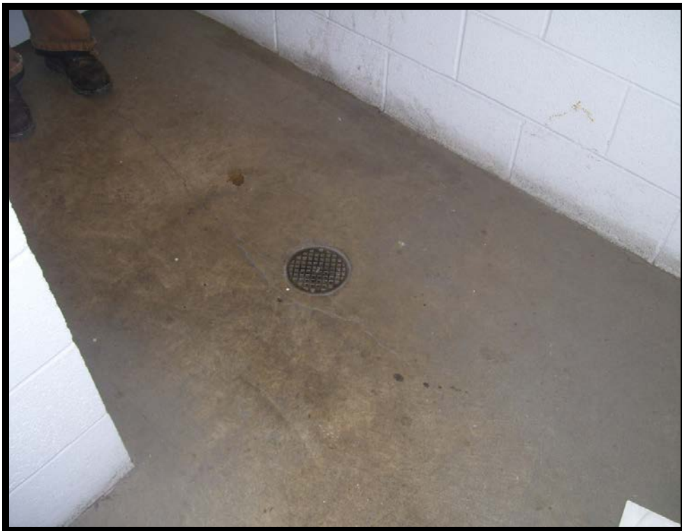
Location #93 – Floor drain staircase corridor (office area, base floor)
