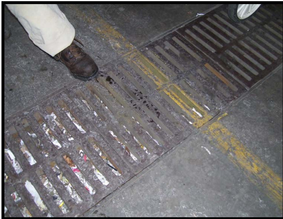
Location # 8 – Trench drain
