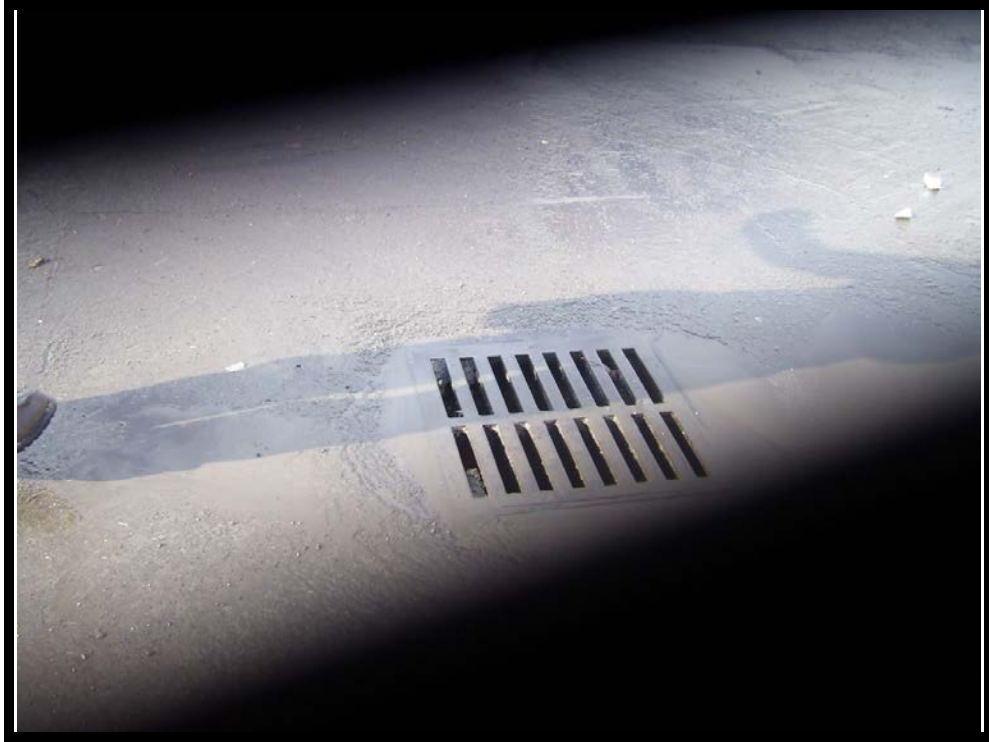
Location #112 – Exterior catch basin
