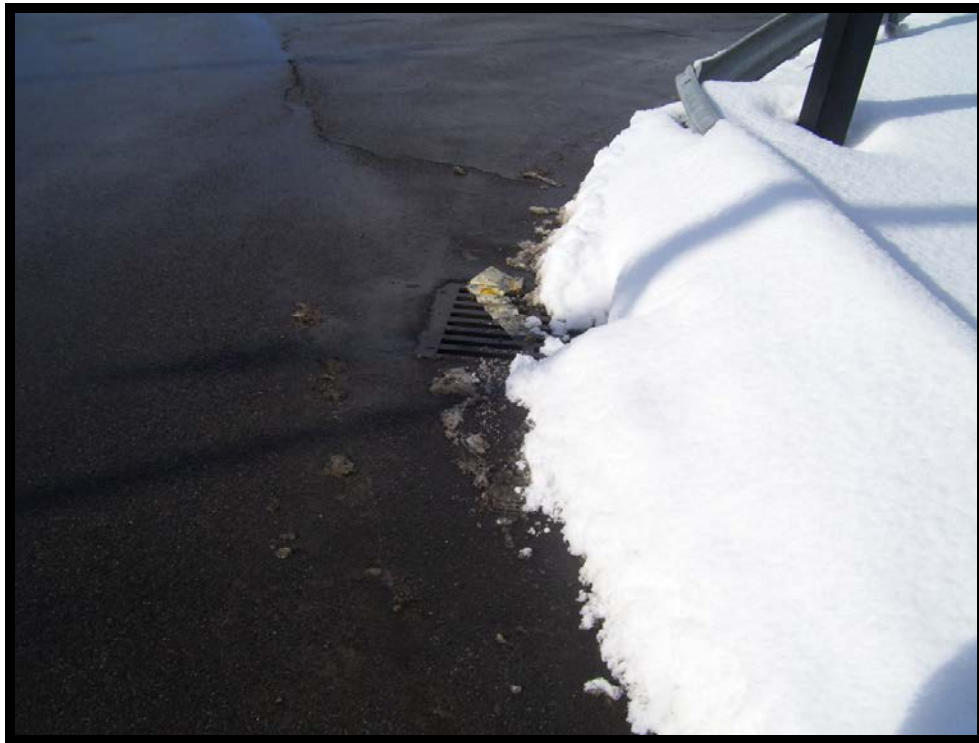
Location #111 – Exterior catch basin
