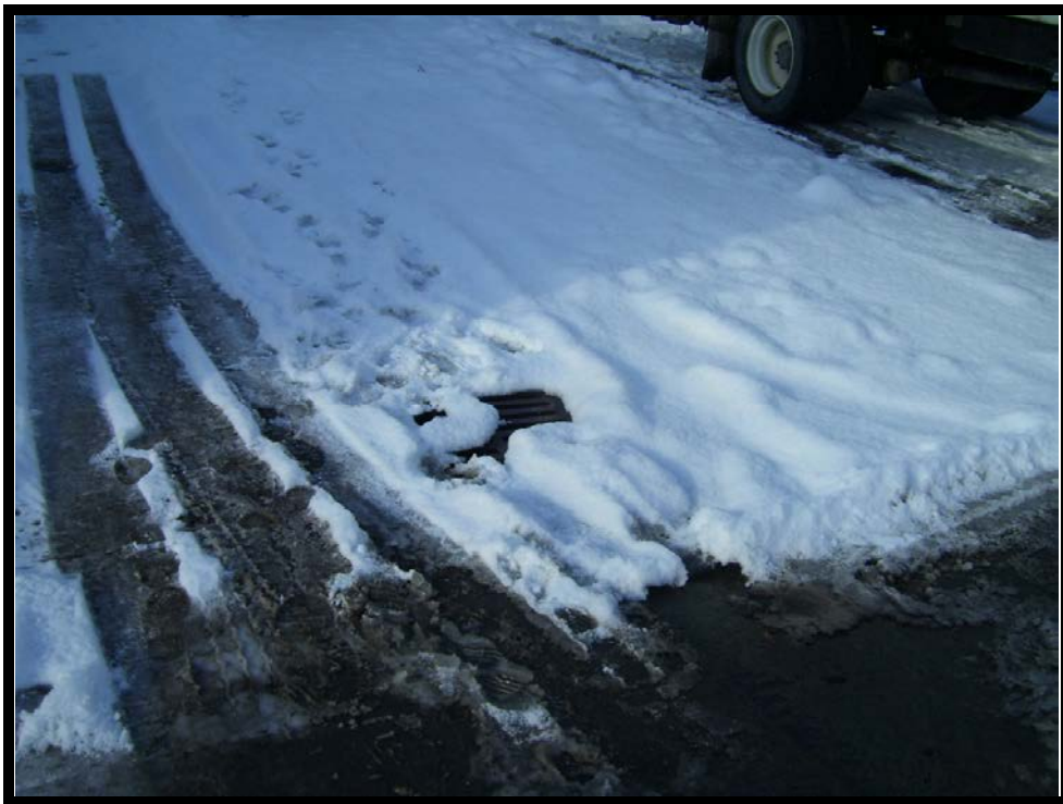
Location #107 – Exterior catch basin
