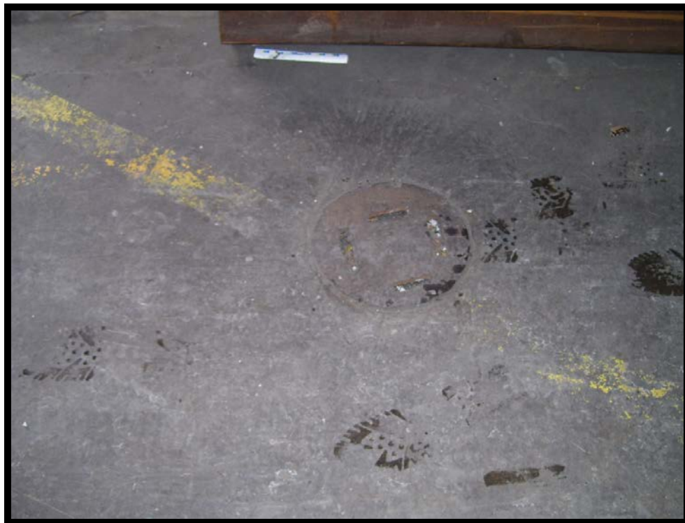
Location #83 – Floor drain
