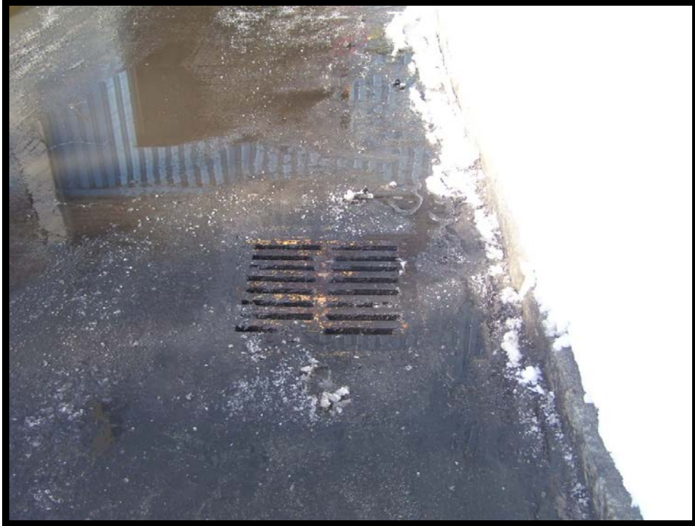
Location #110 – Exterior catch basin
