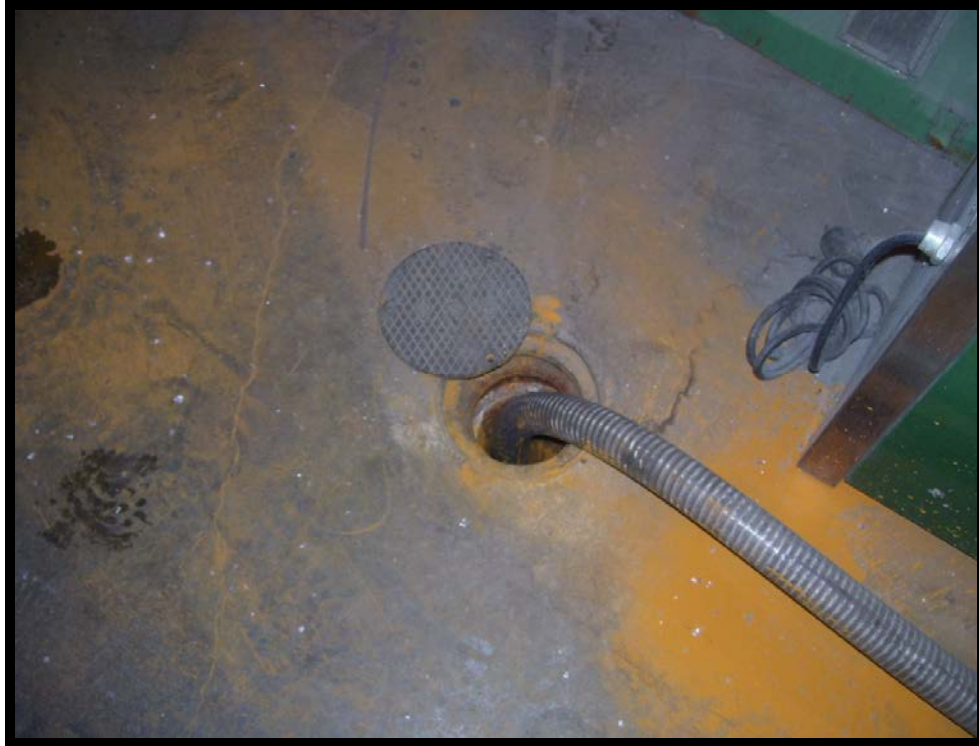
Location #87 – Drain in floor
