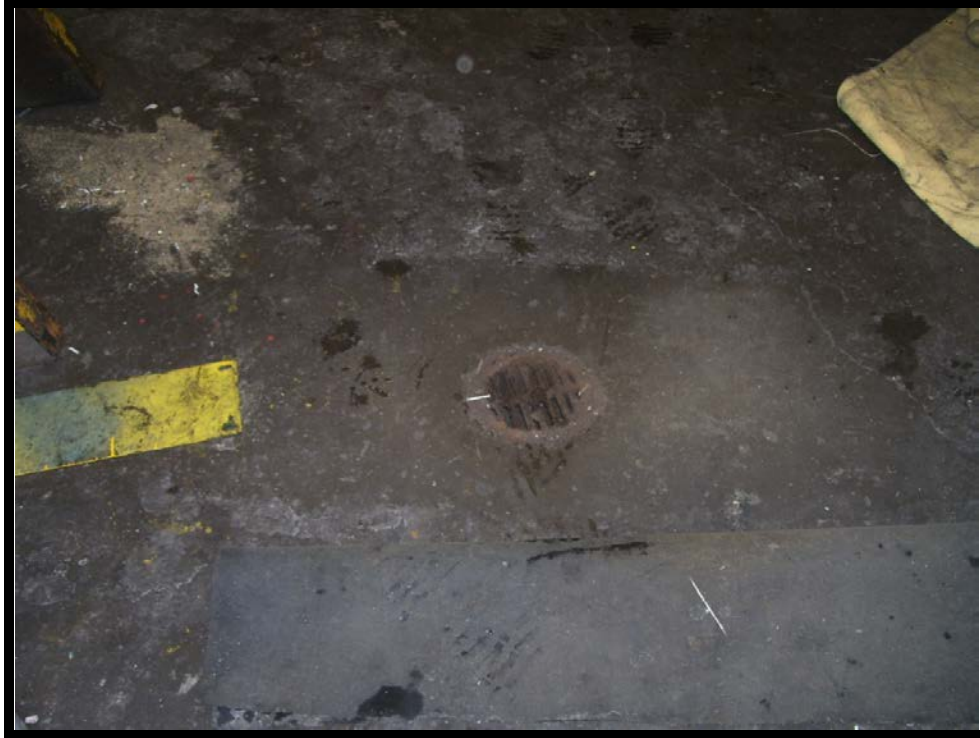
Location #100 – Floor drain in mechanic's room (MCRC)
