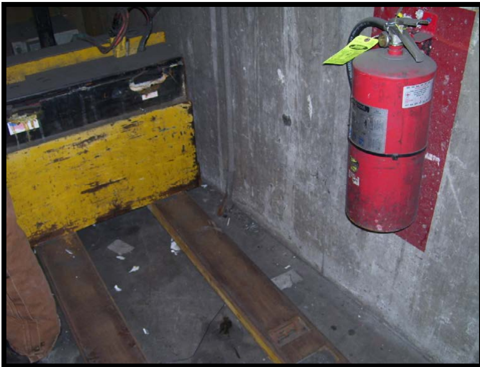
Location #116 – Wall/roof joint near conduit
