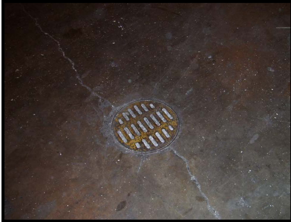
Location #29 – Floor drain
