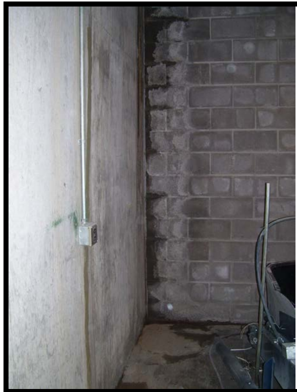
Location #94 – Broken cinder block wall at floor in shredding room
