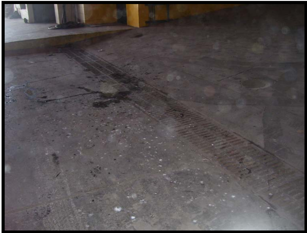
Location #52 – Floor trench
