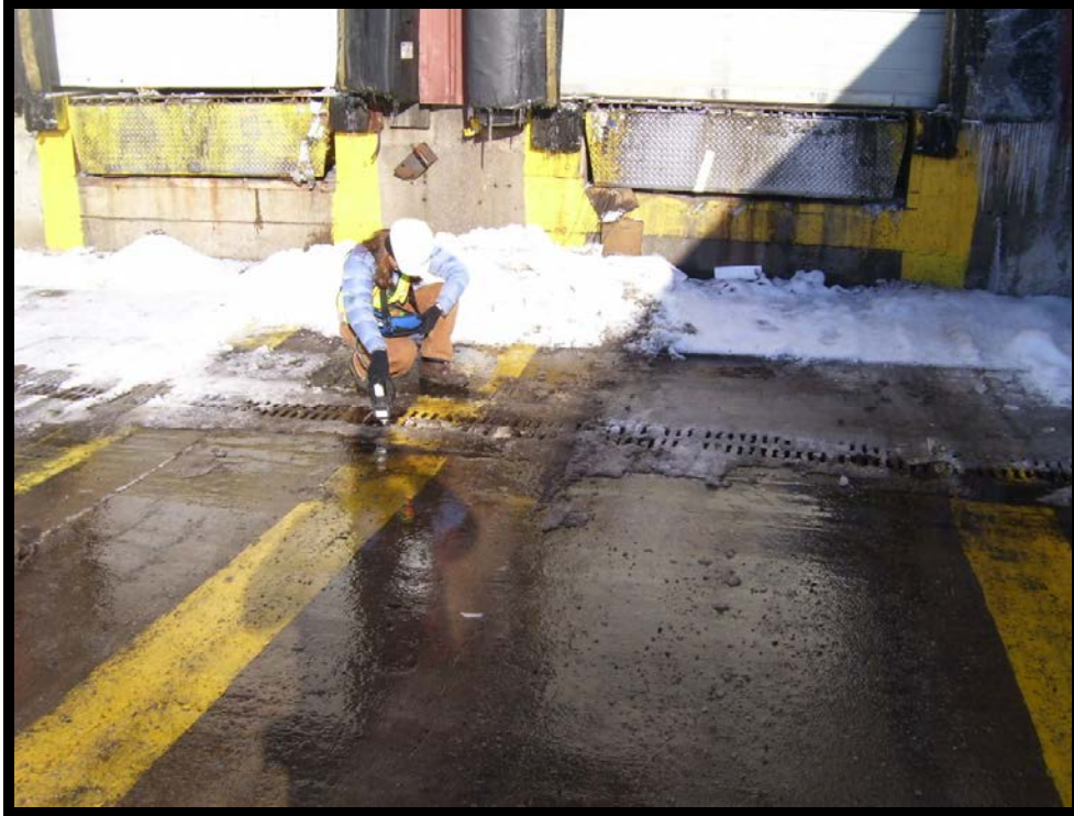
Location #103 – Exterior trench drain
