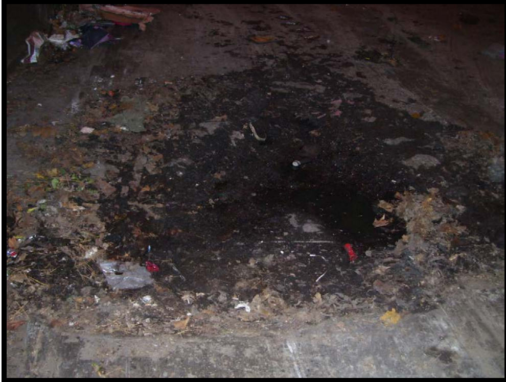
Location #48 – Large open floor space
