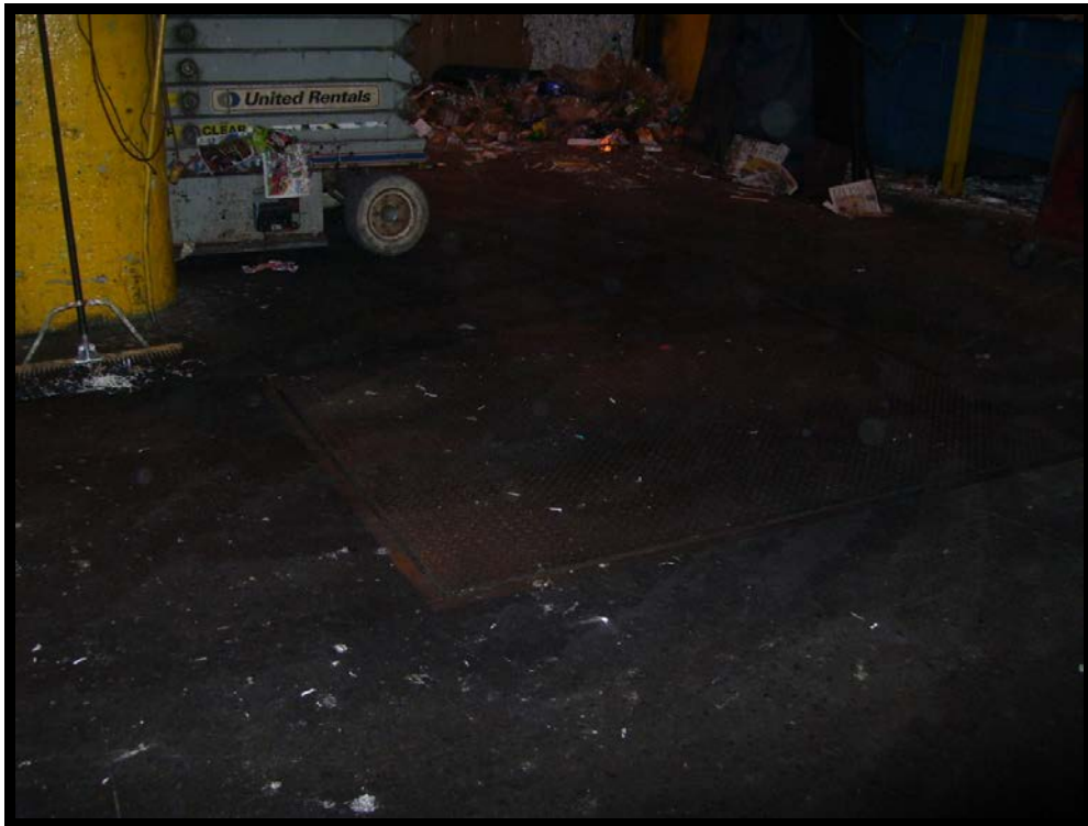
Location #75 – Steel plated vault area
