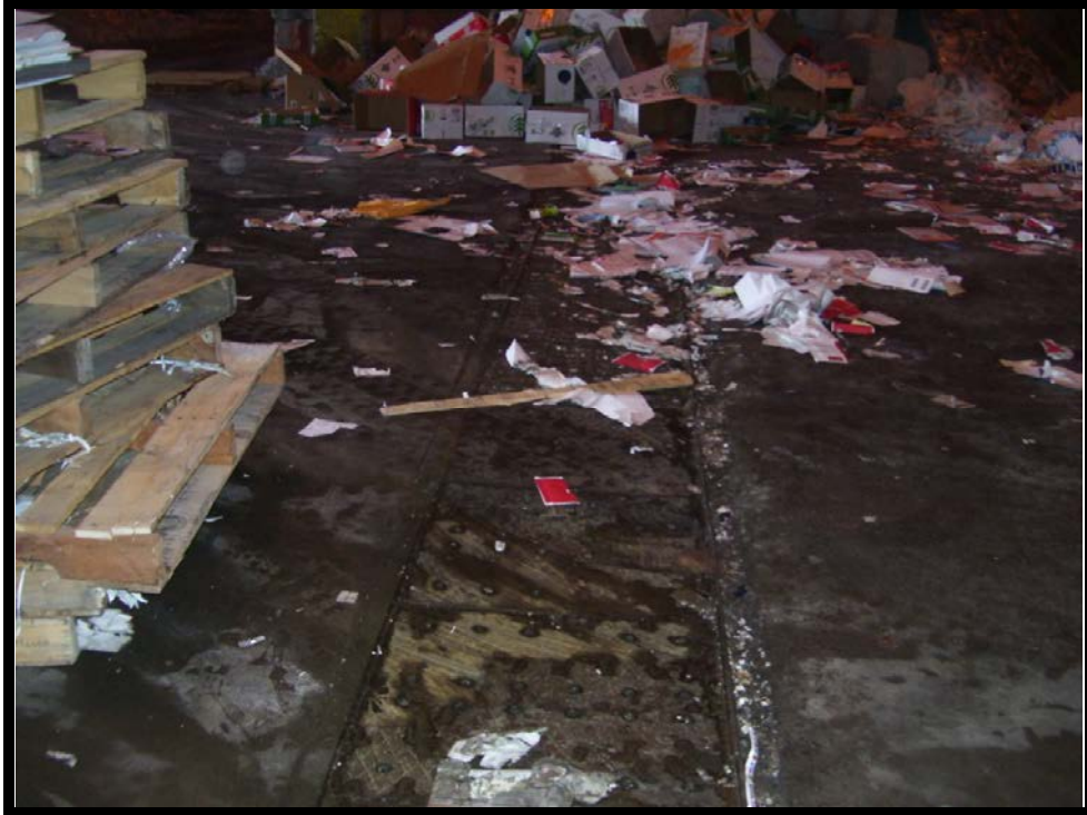
Location #24 – Trench drain
