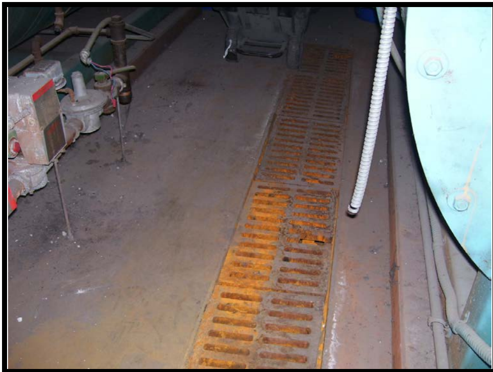
Locations #5 & #6 – Trench drain in boiler room
