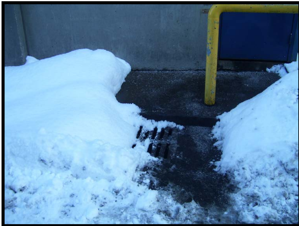
Location #99 – Catch basin
