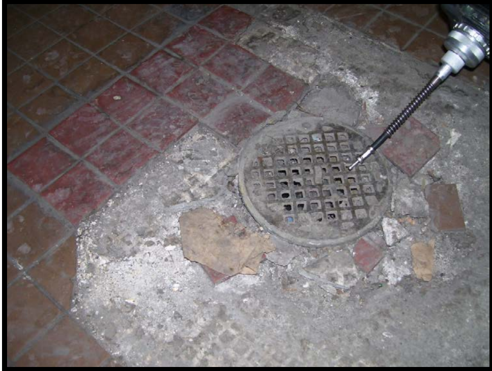
Location #44 – Floor drain
