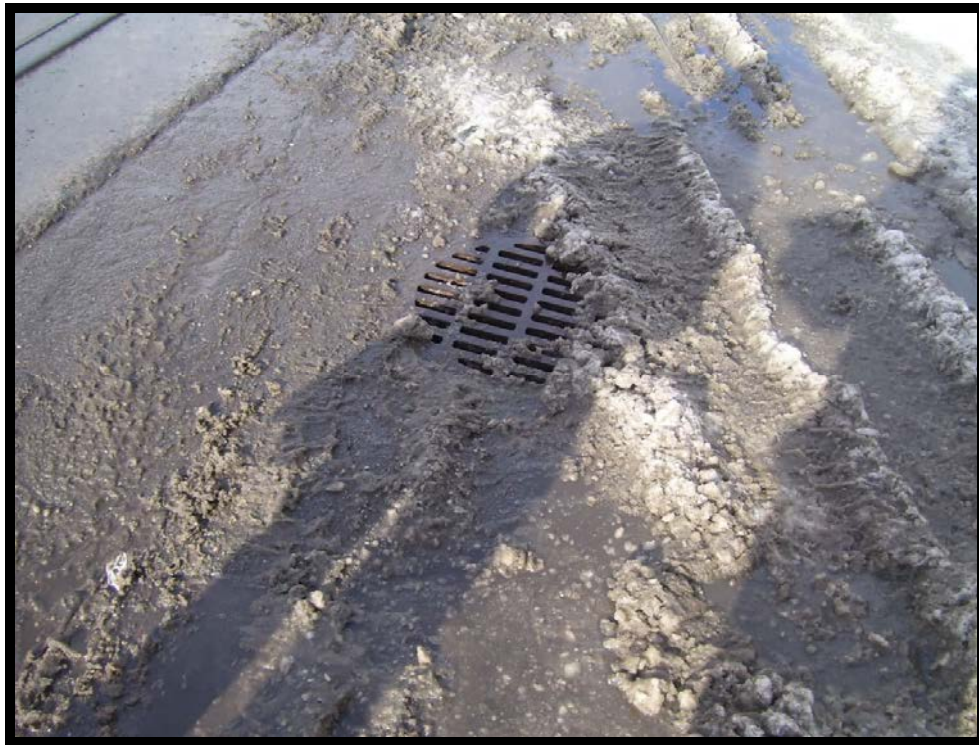
Location #113 – Exterior catch basin
