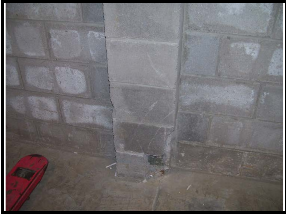
Location #94 – Broken cinder block wall at floor in shredding room
