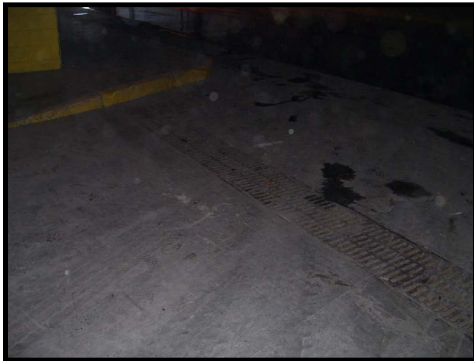
Location #55 – Floor trench
