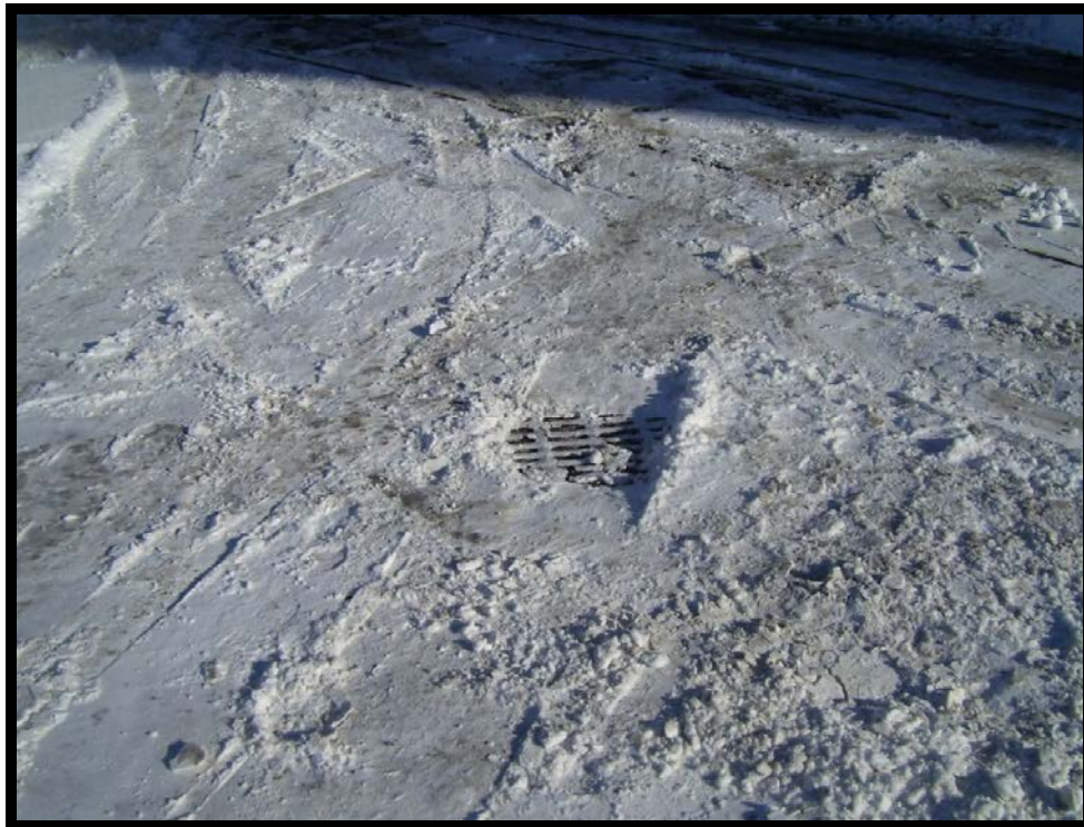
Location #102 – Exterior catch basin
