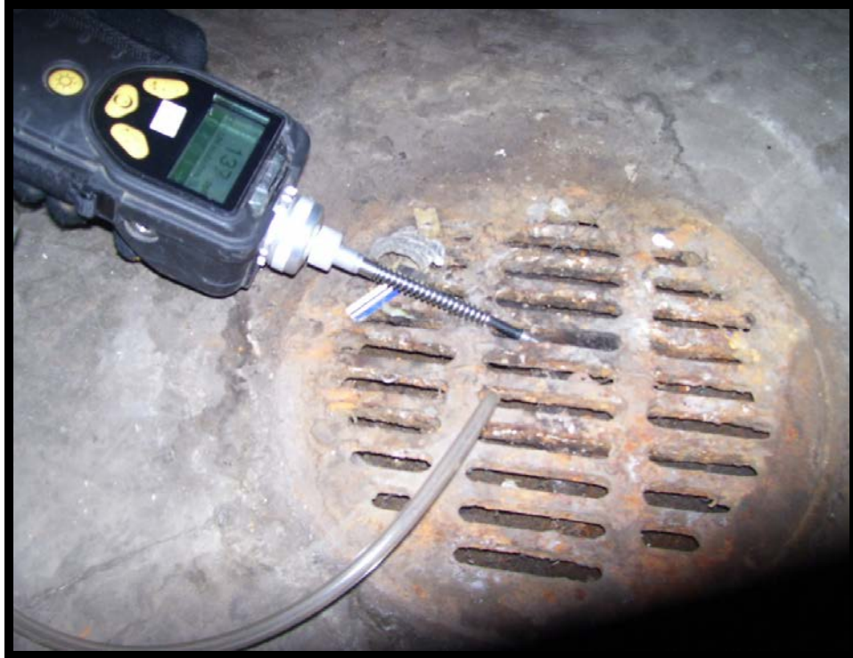
Location # 7 – Floor drain in boiler room
