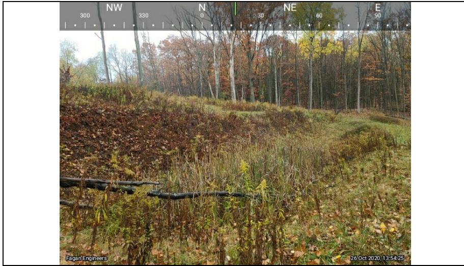
5.) Facing northeast toward the side slopes of Sediment Trap 2. A view of the erosion that appears to have ceased with increased vegetation, minor bare areas are due to the slope and rocky nature of the soil.
