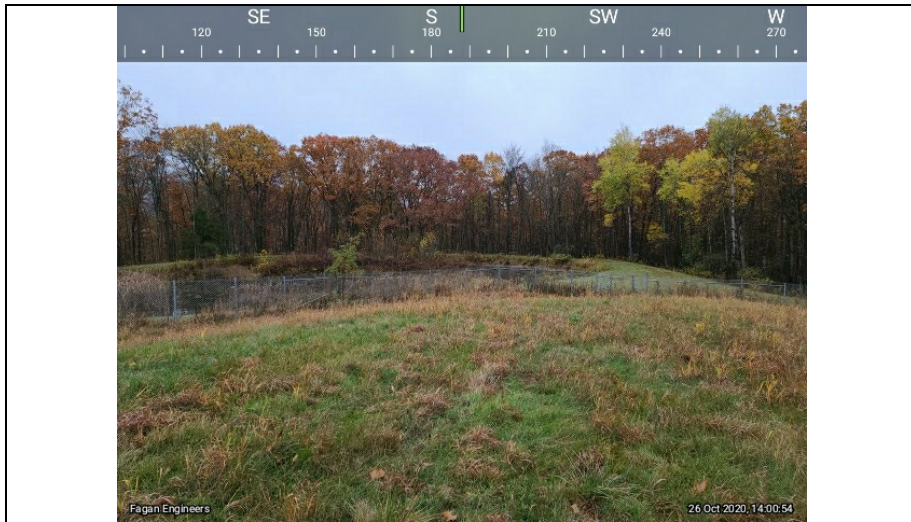
13.) A current view of the upper WMA. Stabilization was observed to be in good condition.
