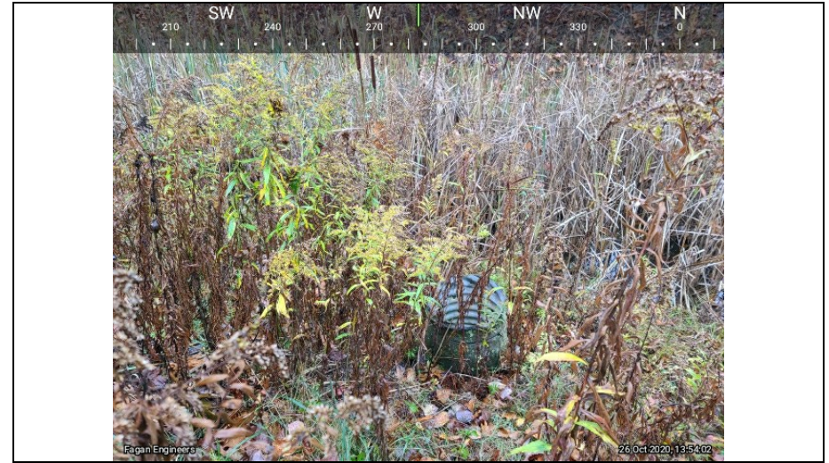
6.) A closeup view of the outlet structure in Sediment Trap 2.
