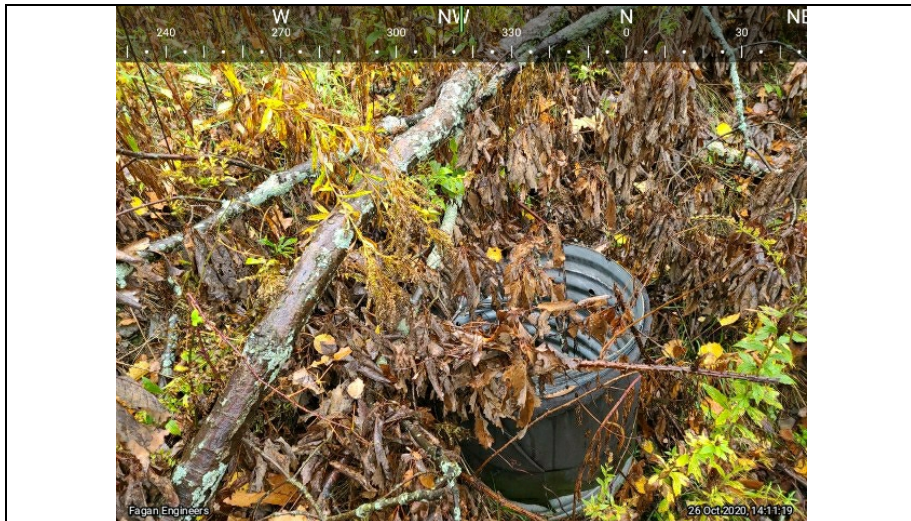
23.) A closeup view of Outlet Structure of sediment trap 1.
