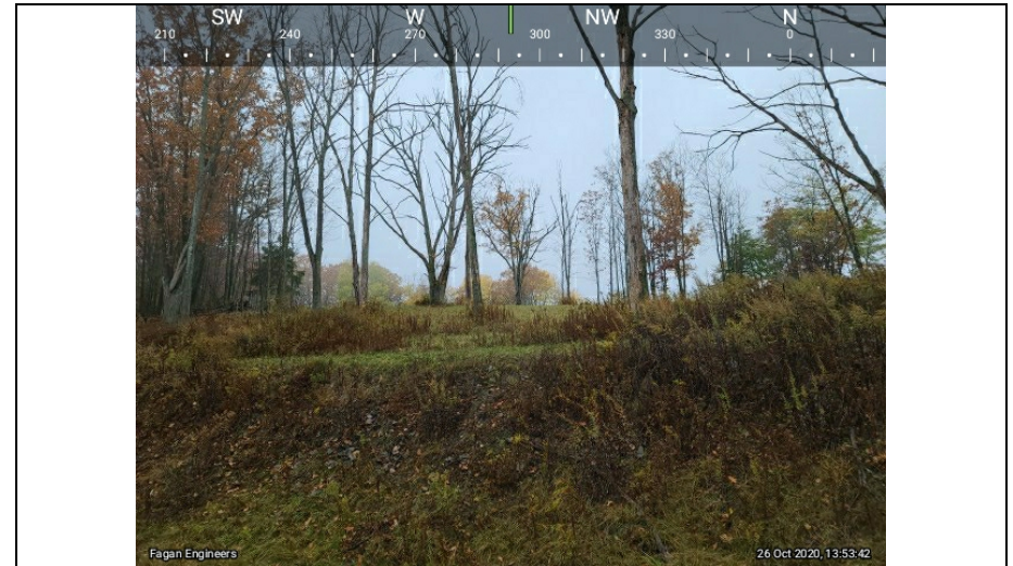
4.) Facing north toward the side slope Sediment Trap 2. Erosion appears to have ceased with increased vegetation, minor bare areas are due to slope and rocky nature of the soil.
