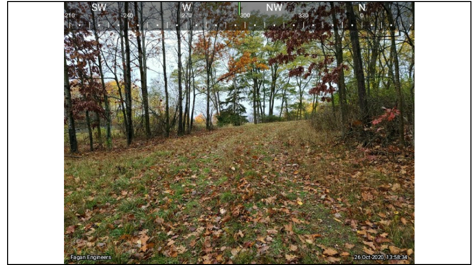
10.) Facing northwesterly along access road, note grass vegetation establishing itself in center and along edges of road. Function does not seem to be affected.
