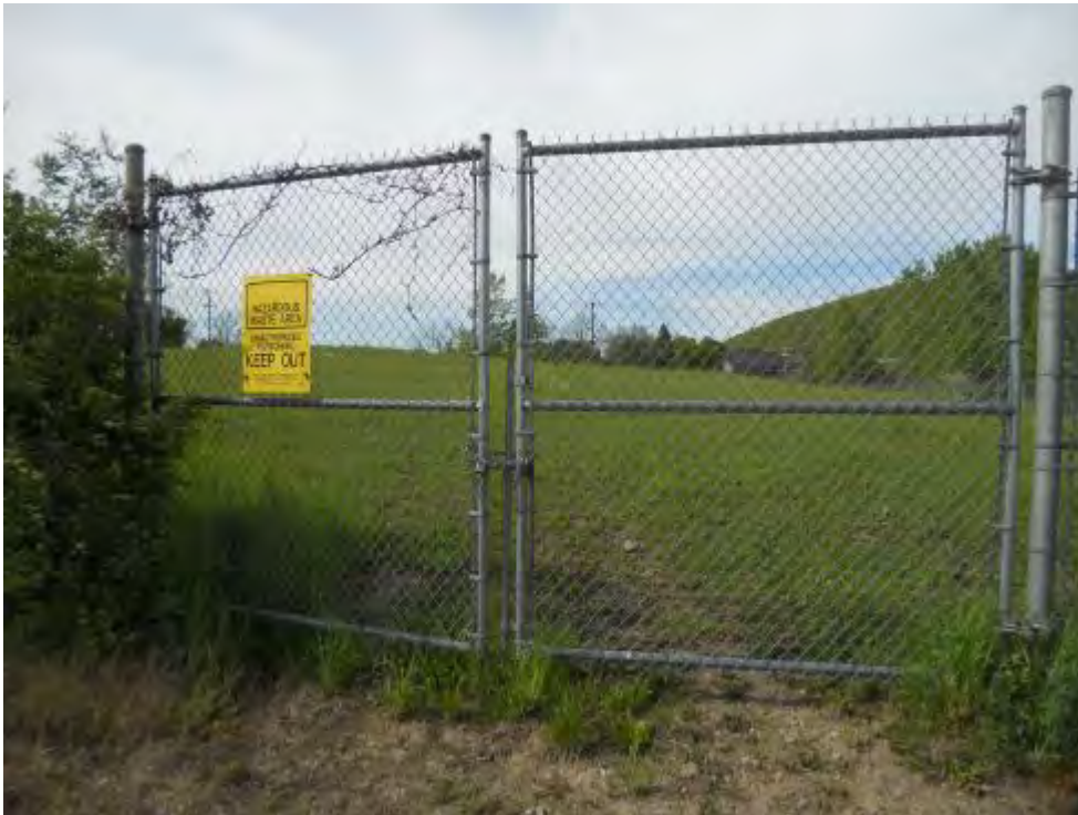
Landfill Access Gate
