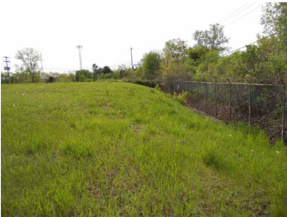
North side of landfill – looking west.
