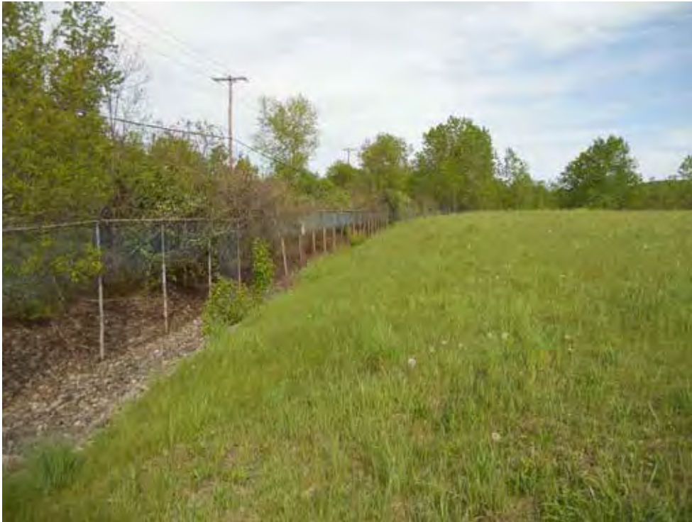
North side of landfill – looking east.
