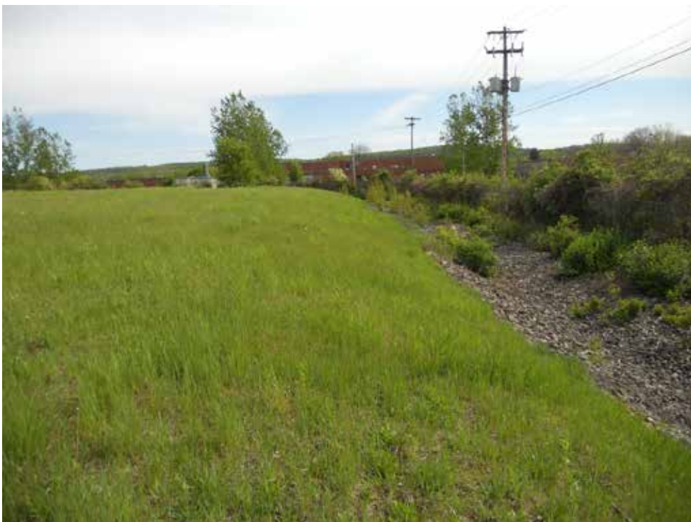
West side of landfill – looking south.
