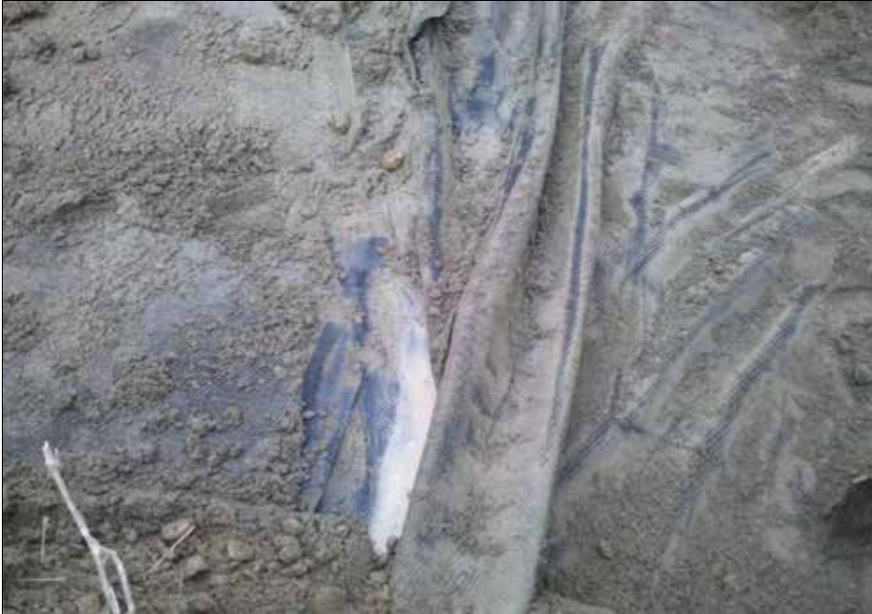
Liner fold in the northeast area.
