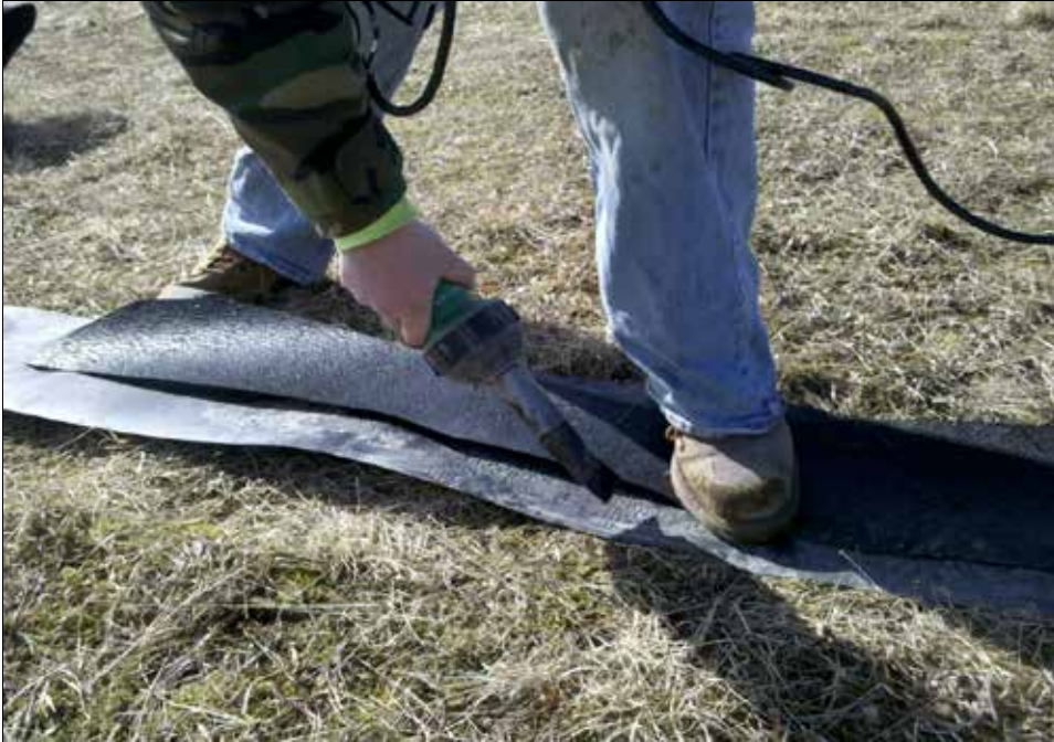
Preparing liner weld test strip.
