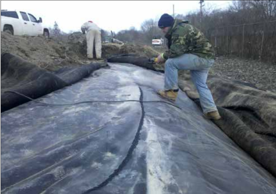
Grinding new seam in northeast area.
