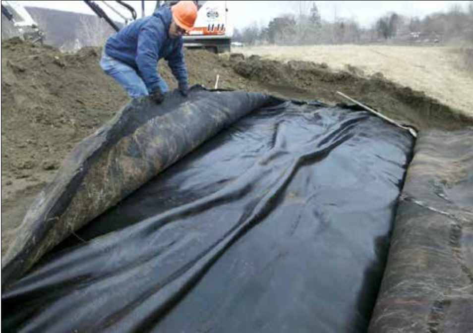
Liner folds flatten as they extend to the east.
