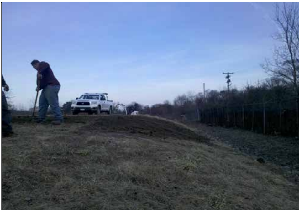
Rake and seed backfilled areas.
