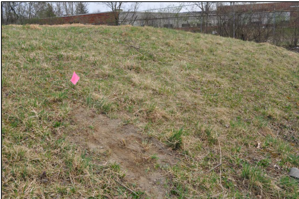
Close-up of filled rodent burrow.
