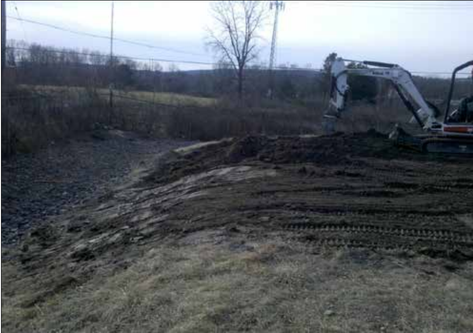
Backfilling repair areas.
