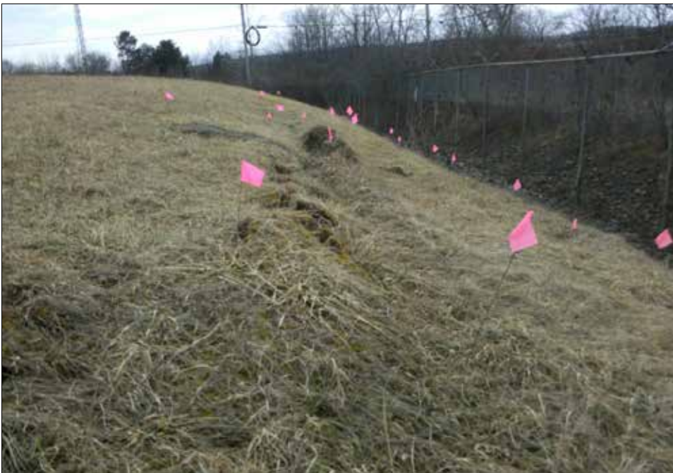
Liner visibly protruding through surface material.
