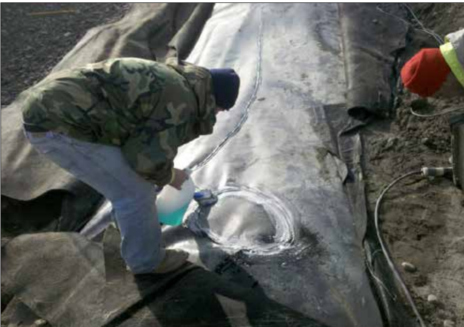
Prepping the weld with a soapy solution for vacuum testing.
