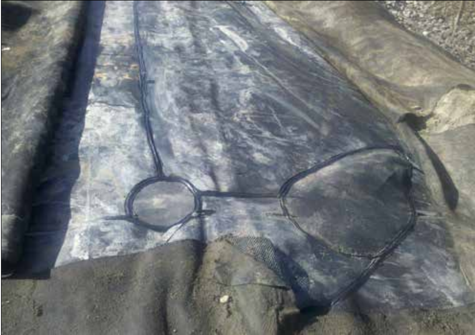
Finished patches and welds.
