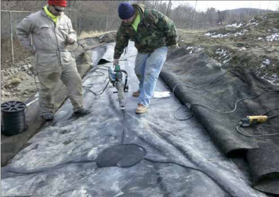
Welding of the liner area after folds and slack was removed.
