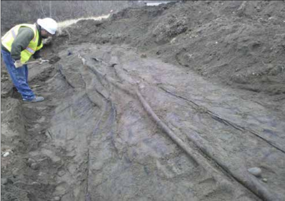
Inspecting fabric and liner.
