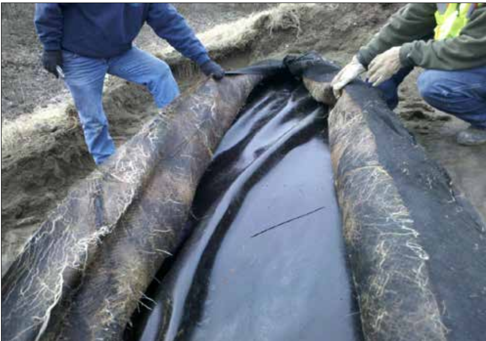
The exposed liner with wrinkles.
