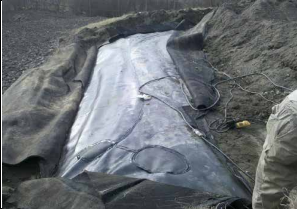
Finished liner repair. Folds and wrinkles removed.
