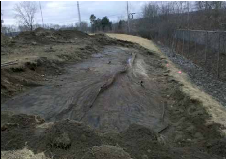
Liner fold extends approximately 50'.
