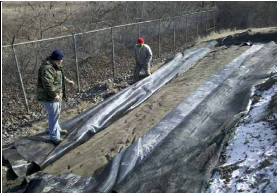
The liner is cut and slack removed.
