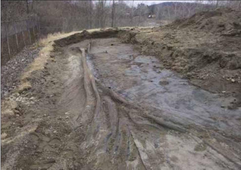
Northeast area - Folds flatten at the east and west extent of the excavation.
