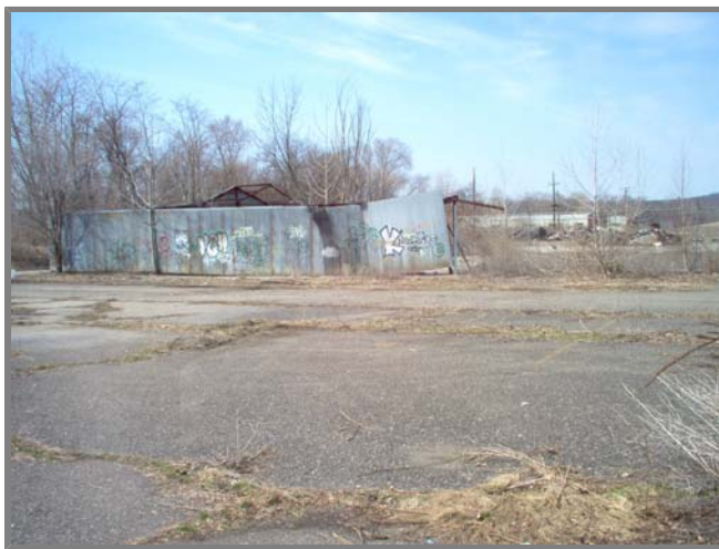
Photo left. View across the leveled foundary site. The school is in the background.
