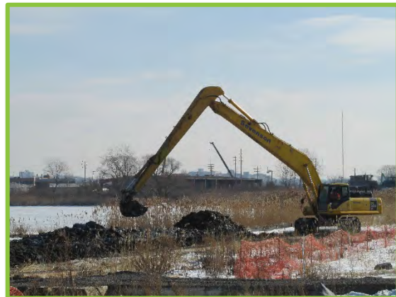
Figure 10: View of Onondaga Lake Outboard Area Excavation
