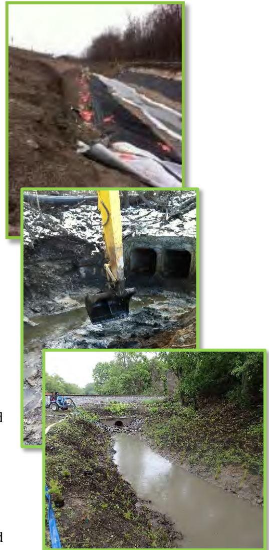
Figure 9: Excavation and Restoration of Site Ditches
