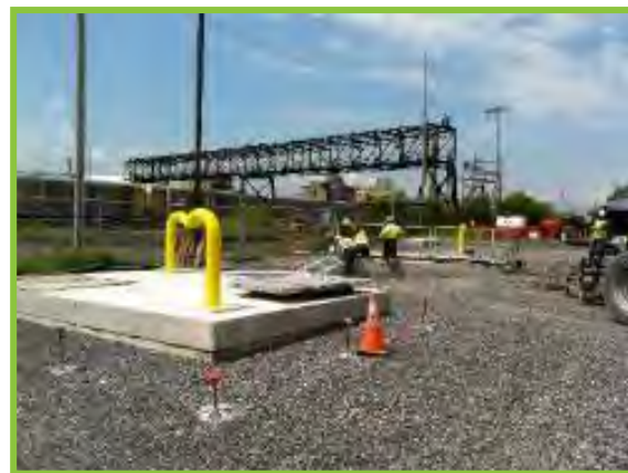
Figure 5: Installation of East Flume IRM Storm Sewer Modifications
