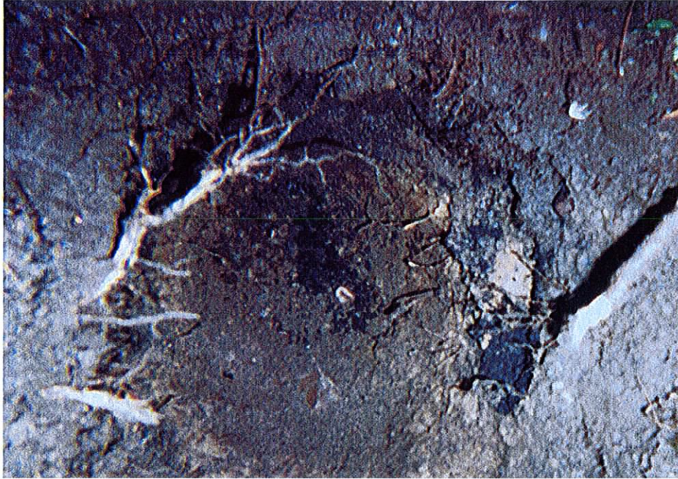
Test Pit #2 Photo taken on: 5/14/02 Teall Avenue-Nimo station
