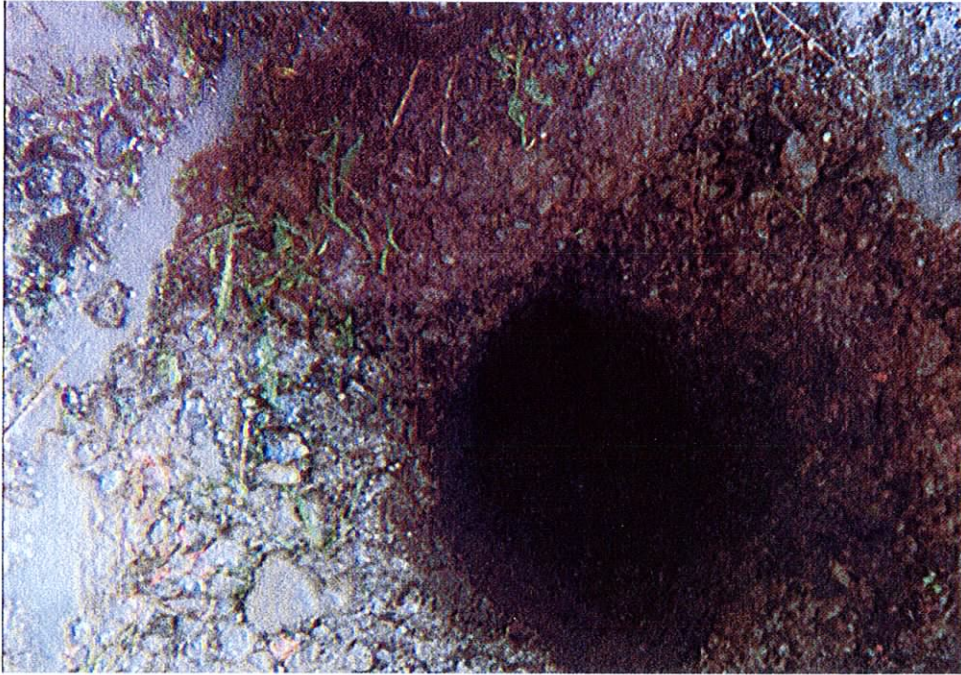
Test Pit #1 Photo taken on: 5/14/02 Teall Avenue-Nimo station
