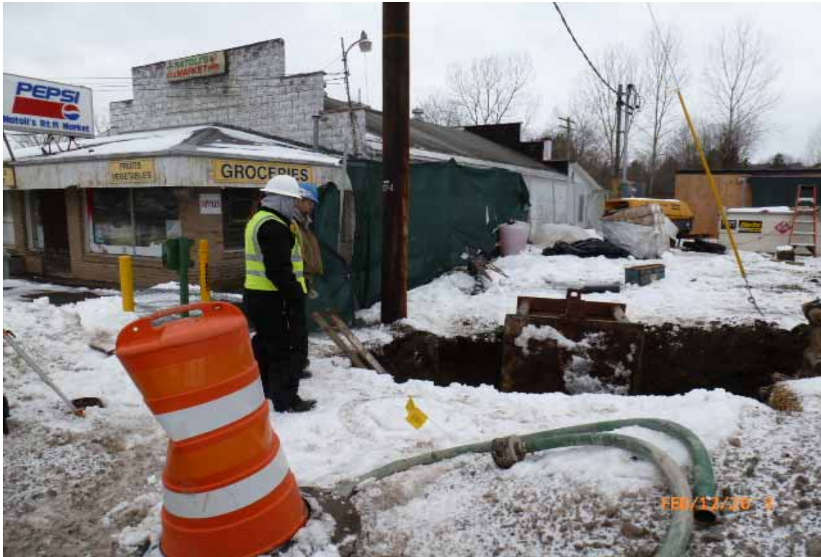
Photo #5: View of southern most end of water main installation trench
