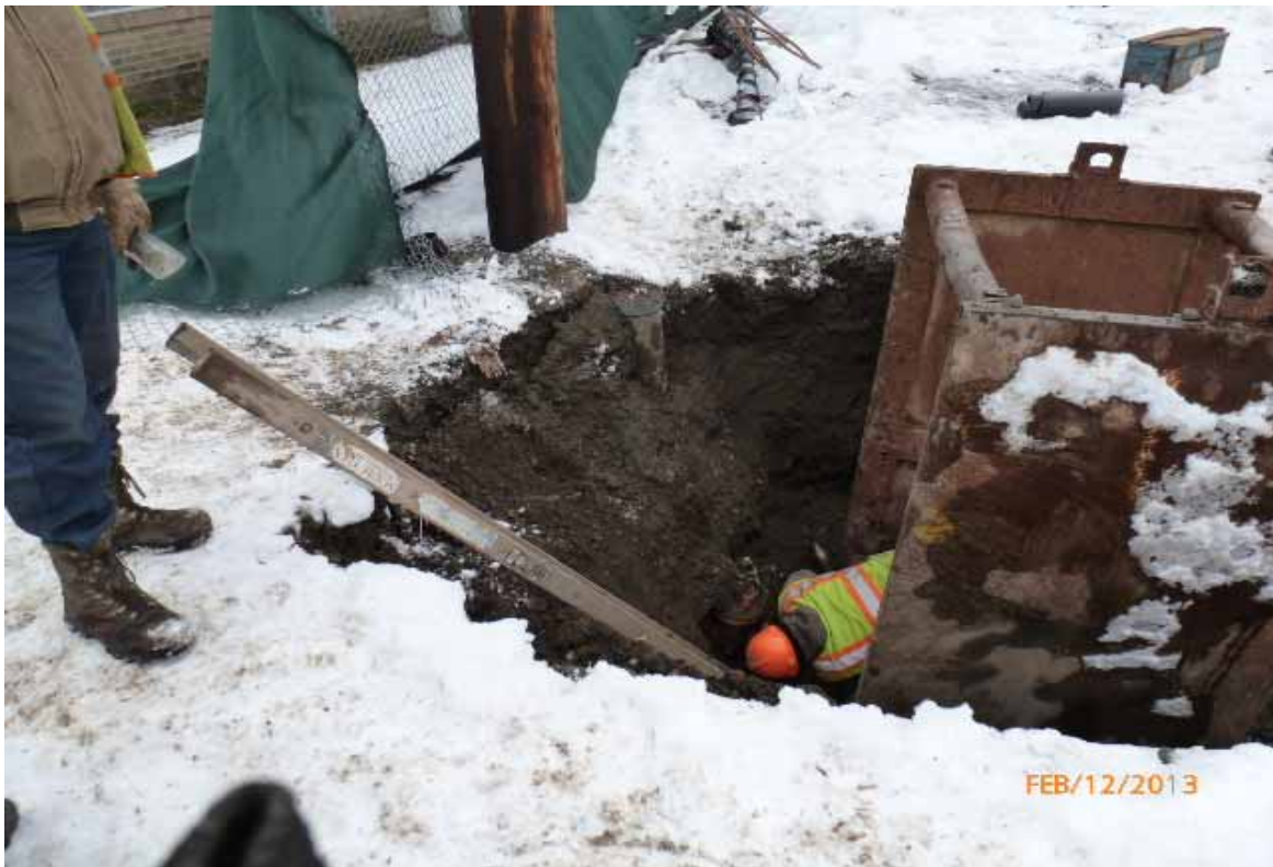
Photo #4: Waterline installation trench southeast of monitoring well MW-11
