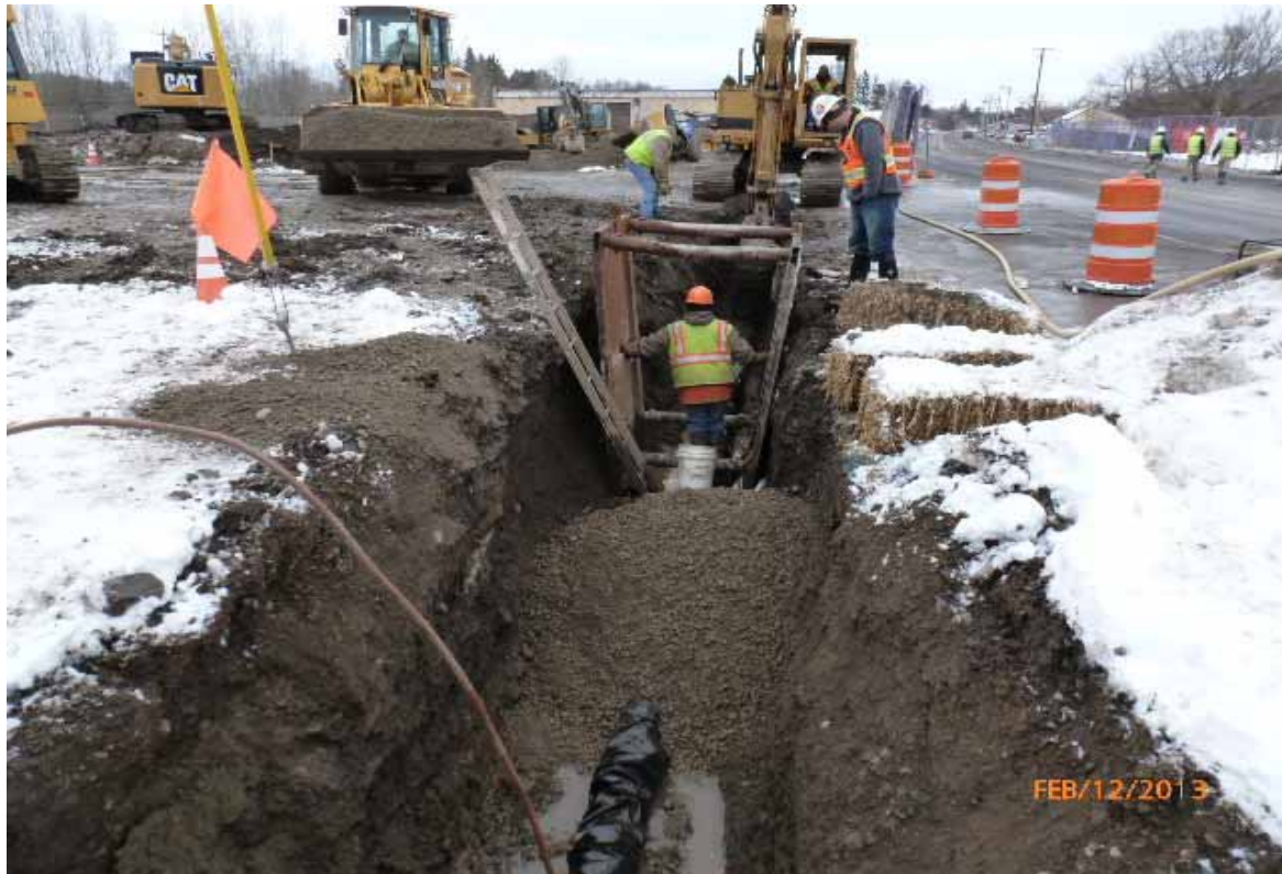
Photo #7: Water main installation trench (additional view)
