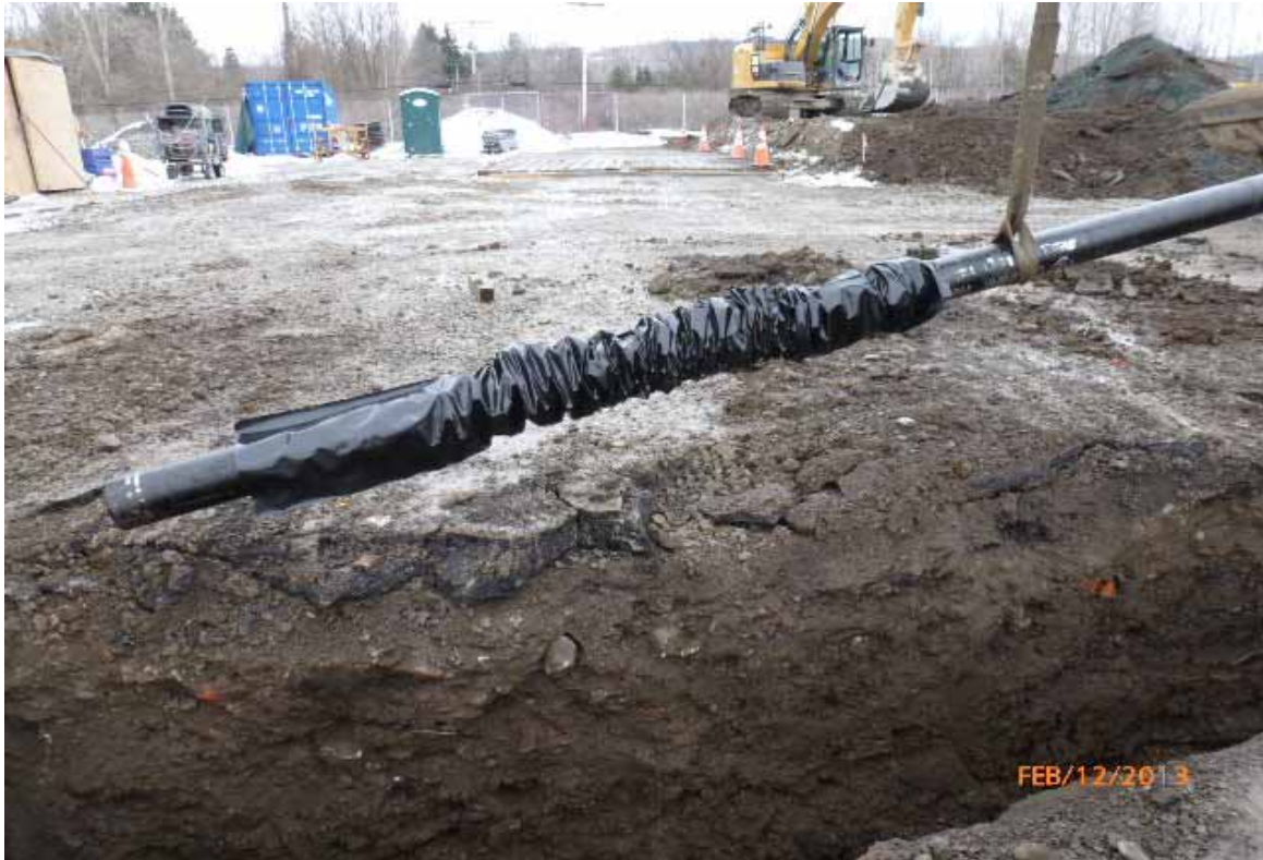
Photo #9: Water main installation trench northeast of MW-11.
