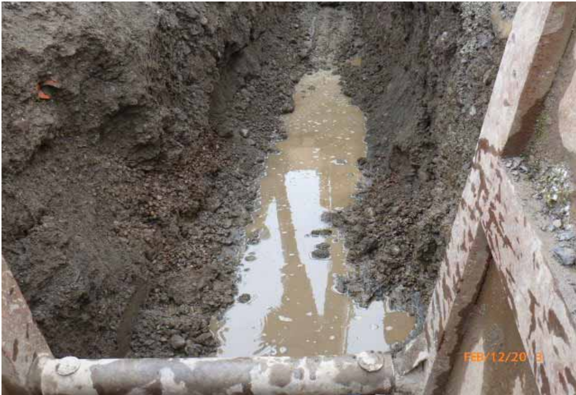
Photo #6: Water in water main installation trench (no sheen present)
