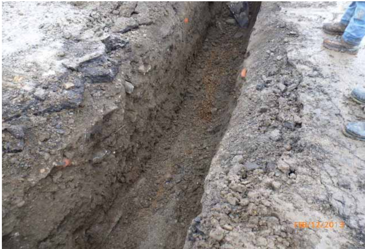
Photo #8: Backfilling of water main installation trench
