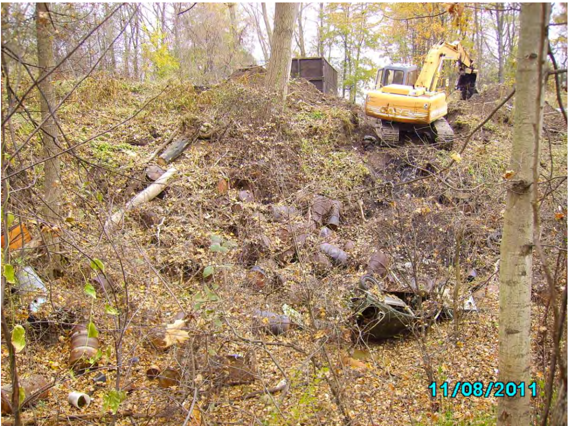
Photo 8. Pond #4 – Removing Debris
