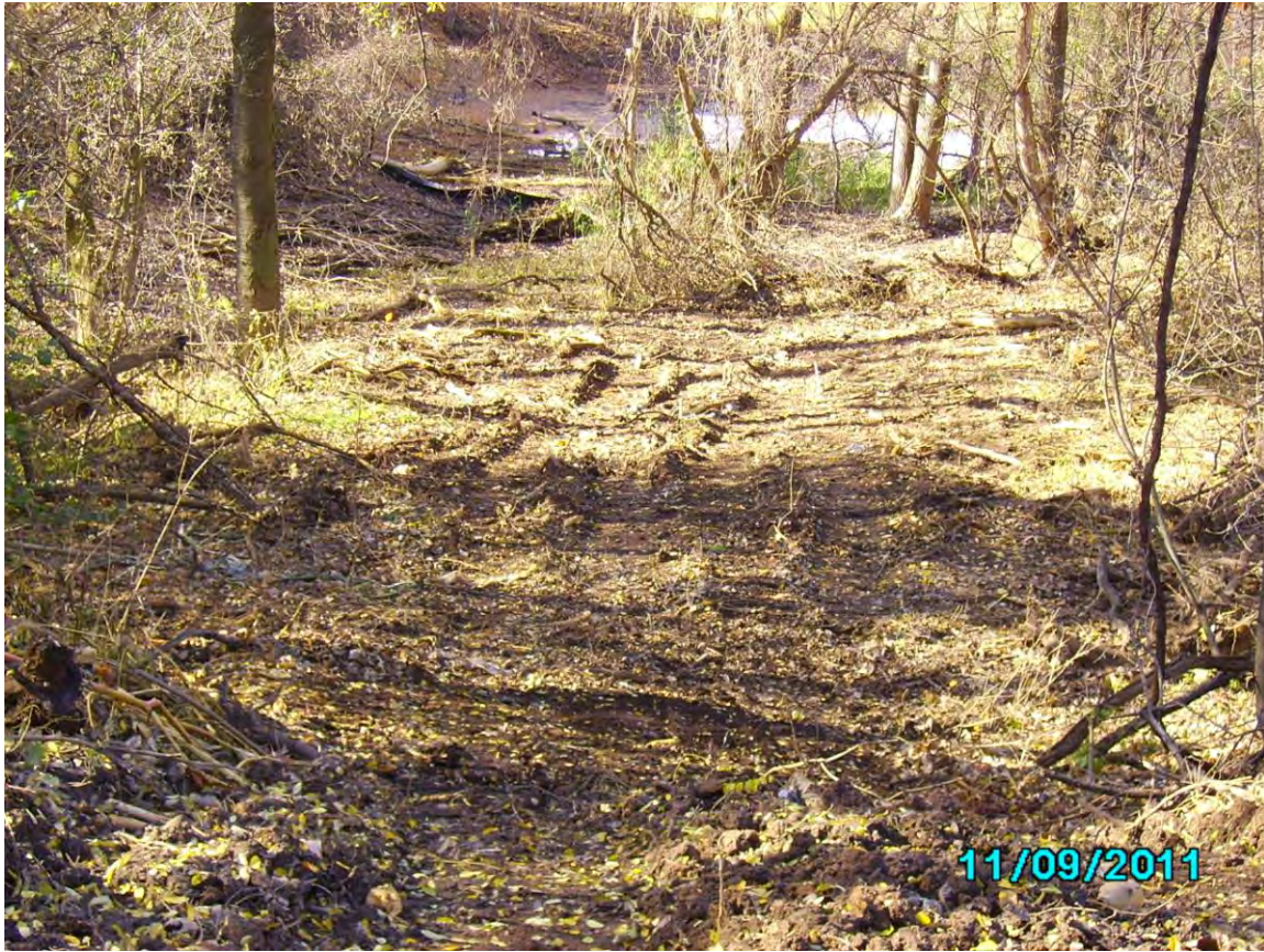
Photo 11. North Area of Pond #3 After Debris Removal
