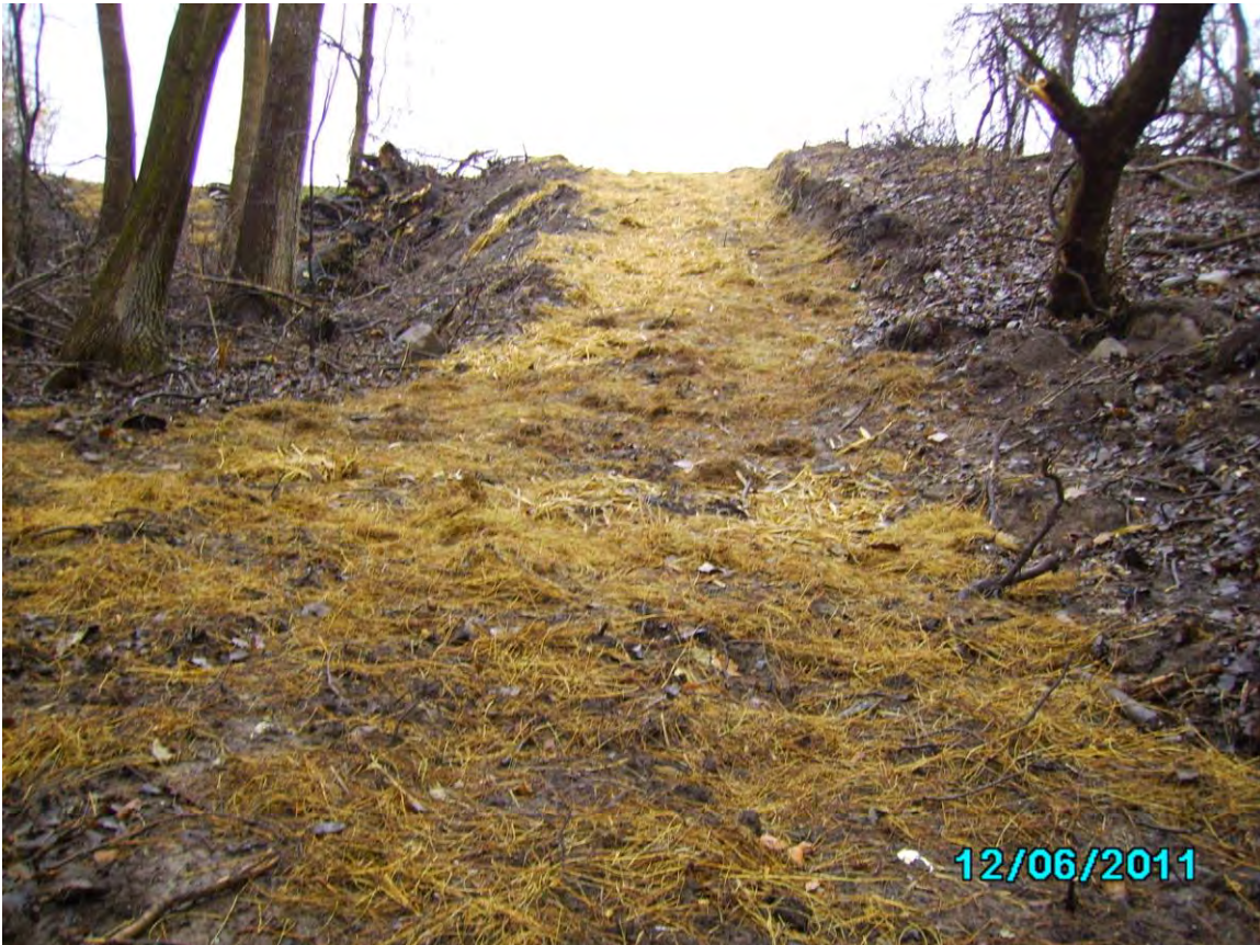
Photo 20. Pond #3 East Area Mulched
