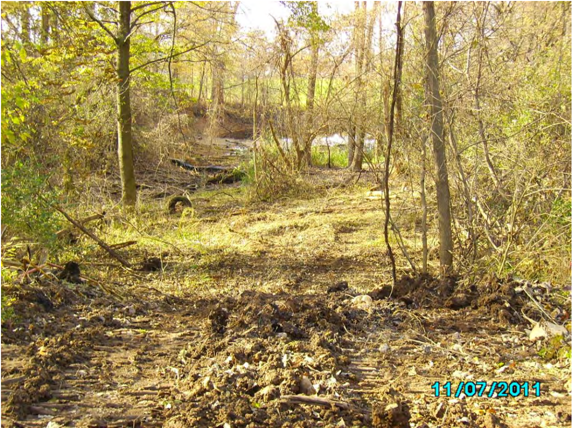
Photo 1. North Area at Pond #3 – Start of Debris Removal
