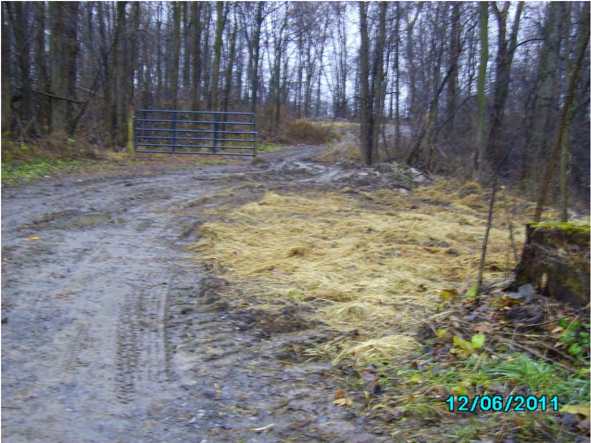
Photo 15. Gate at Access Road – Soil Berm Removed to Bypass the Gate
