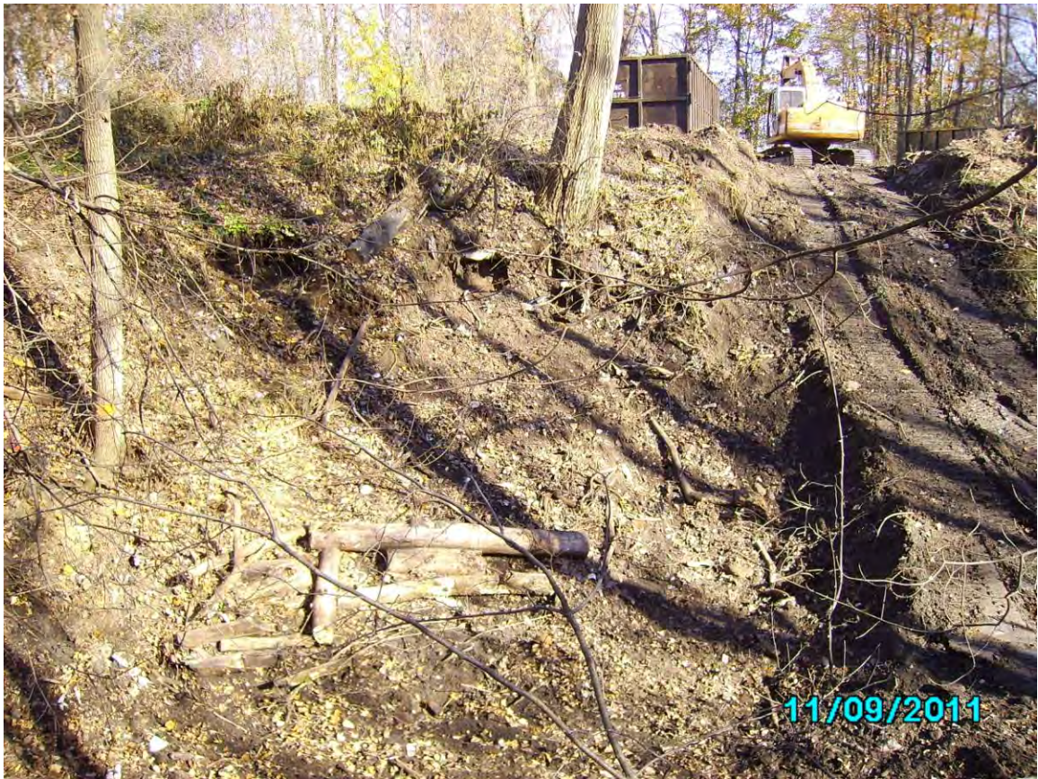
Photo 9. Pond #4 Access Ramp
