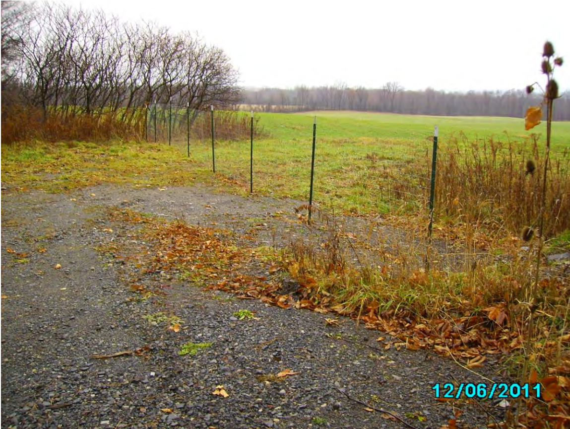
Photo 19. Fence Installed to Limit Access
