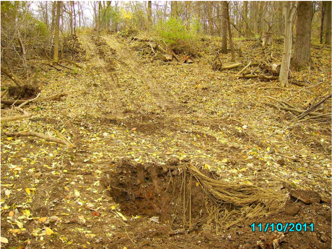
Photo 14. Post Debris Removal – East Area of Pond #3
