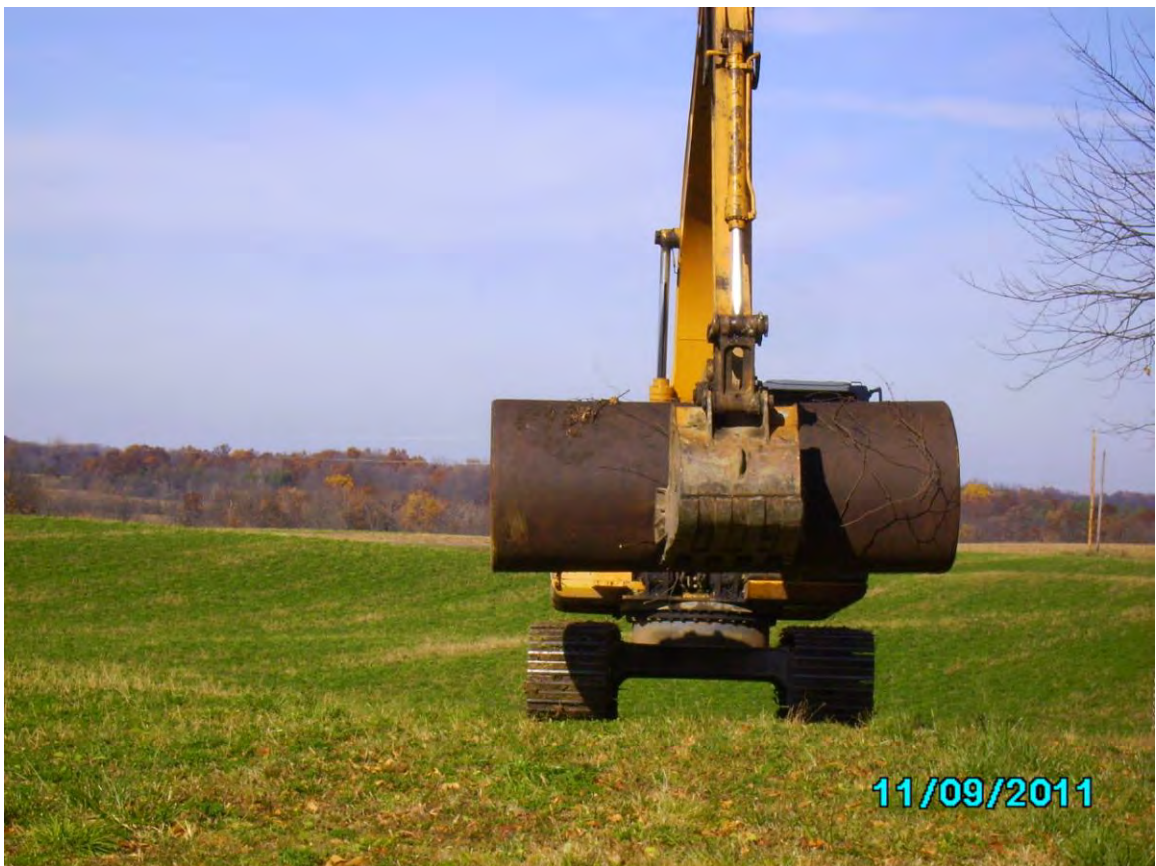
Photo 10. Storage Tank Being Transported to Roll-off for Disposal
