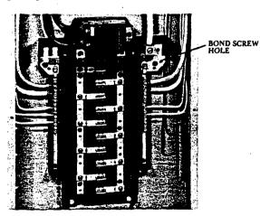
Wire neutral and equipment ground only in direction indicated by arrows. If required, ground and bond neutral to box using screw or straps provided. Straps must be placed in screw or large neutral holes.
