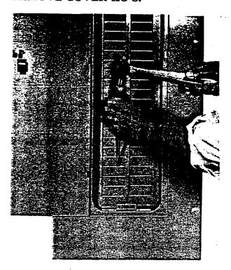
Place screwdriver as shown and tap with hammer.
