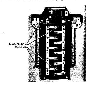
Back out mounting screws and save for reuse.
