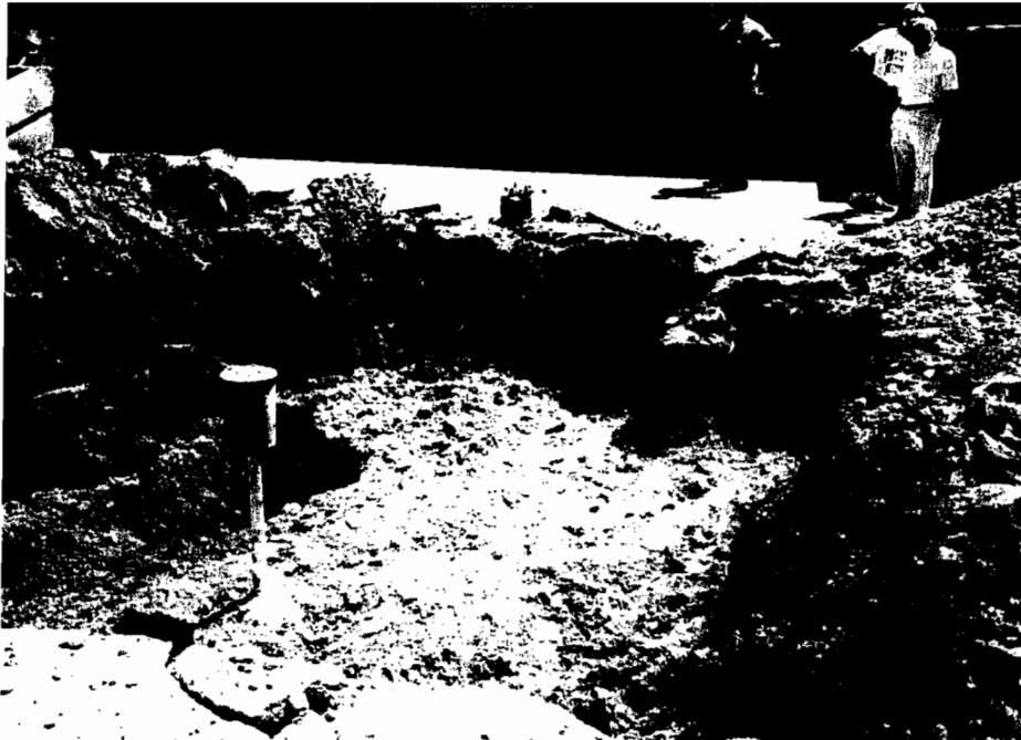
Photograph of the soil excavation taken from the southwest corner of the excavation, looking northeast. Monitoring well 6 is visible in the center of the excavation. (June 17, 1993)
