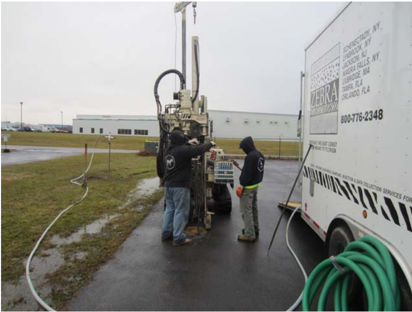
Injection Point Installation
