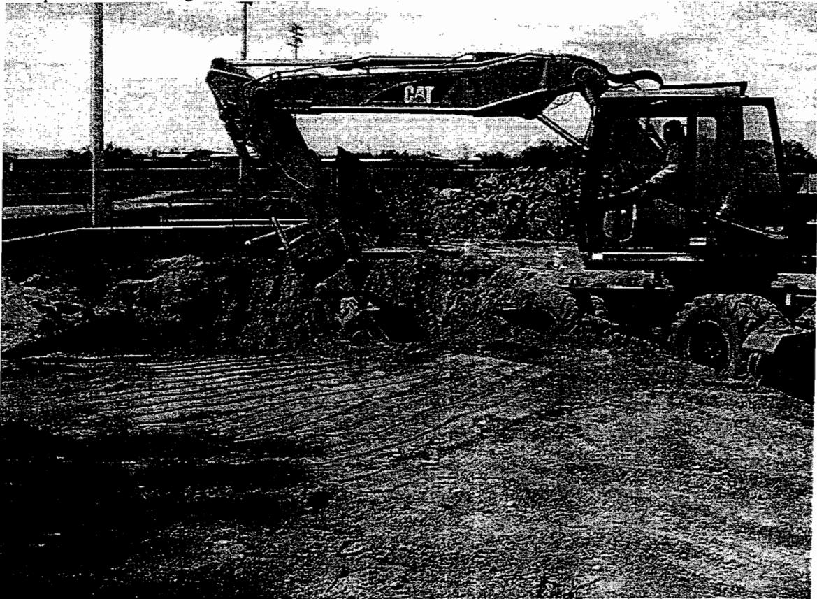
The excavator is compacting the material while backfilling in lifts for compaction.
