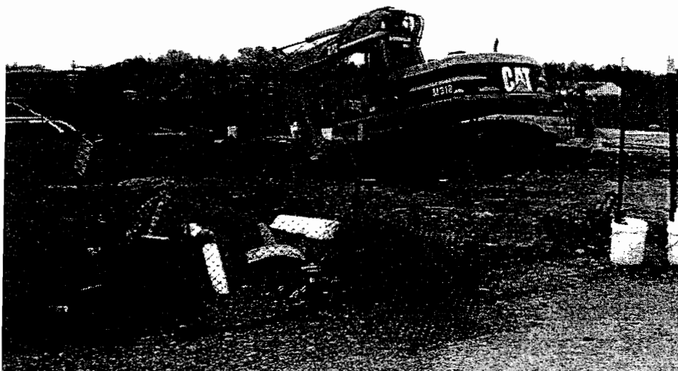
Excavating soil at LCP 6.
