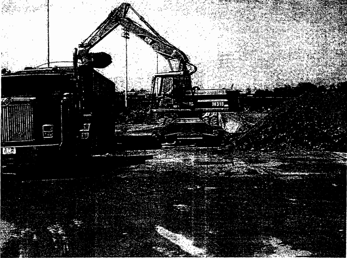
The excavator is loading the truck from the LCP-6 contaminated soil stockpile.
