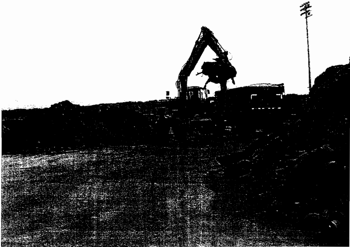
Continue load trucks for offsite disposal.
