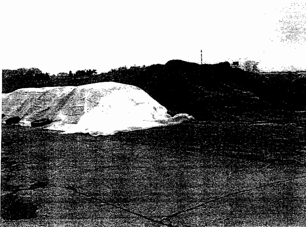
Covering soil stockpiles with poly sheeting.
