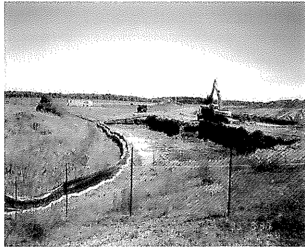
Pumphouse 5 Site -1999 Initial Excavation
