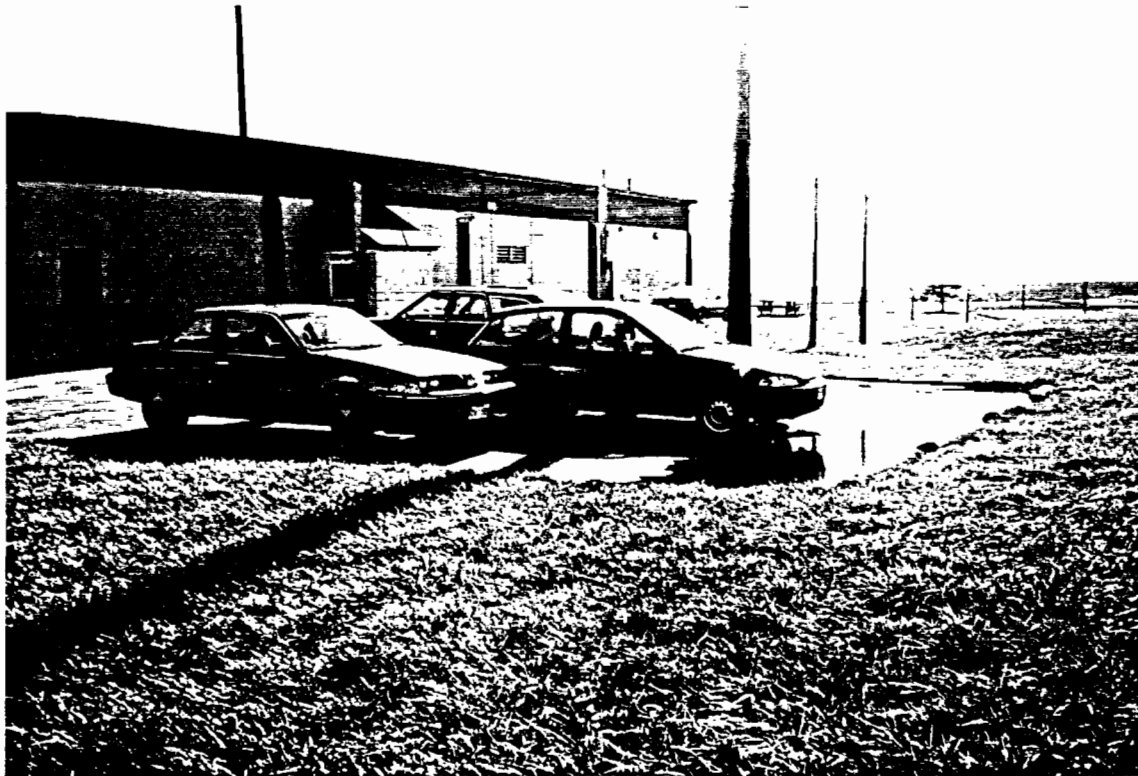
Photograph 53. Lockport Annex; note standing water on top of hillock, asphalt parking area, and office building.
