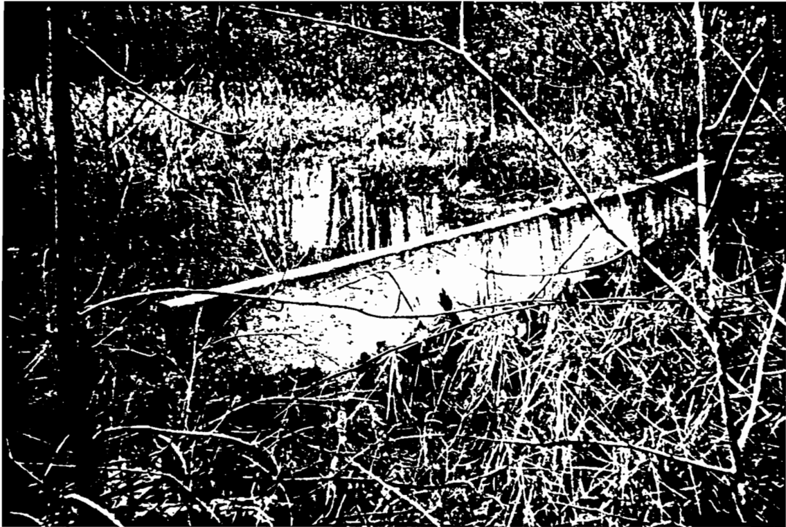
Photograph 38. Area 12; concrete dam for former fishing pond, now adjacent to a landfill.
