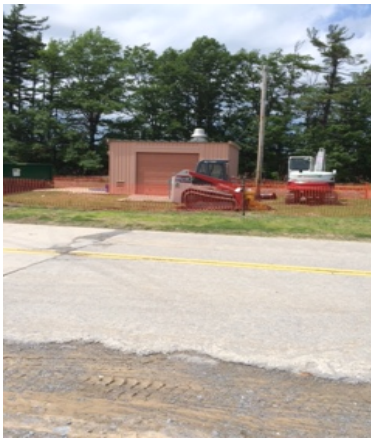
Equipment Delivered and Exclusion Zone Established
