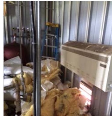
Manual Removal of Fiberglass Insulation
