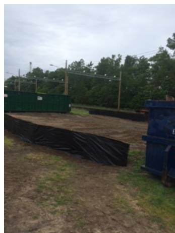
Final Grading with Silt Fence
