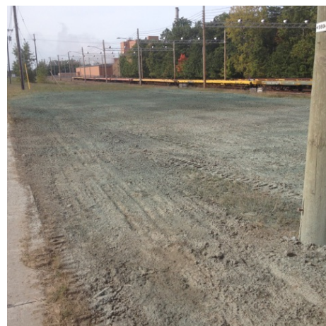
Final Site Restoration (Soil and Seed) at Area 1395
