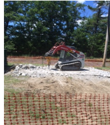
Concrete Slab Removal
