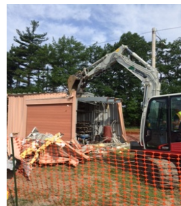
Building Demolition in Progress
