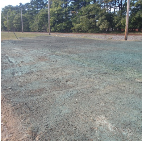
Final Site Restoration (Soil and Seed) at Area 1495
