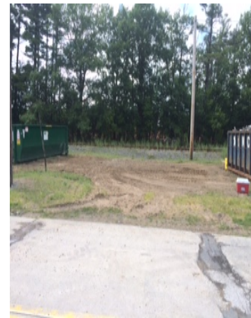
Post Demolition Clean Up
