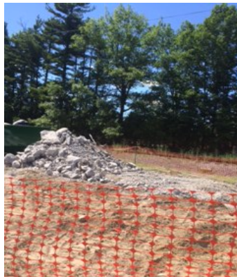
Concrete Slab Removal
