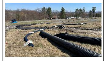
9. Sediment Control Wattle installed at Test Pit #2
