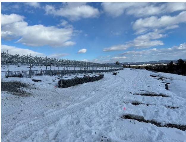
5. Relocated baskets filled with riprap.
