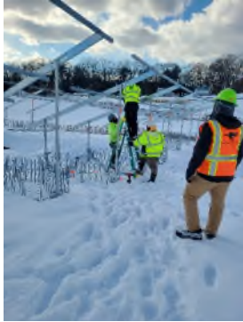
1. I-Build crew in progress of removing racking braces.
